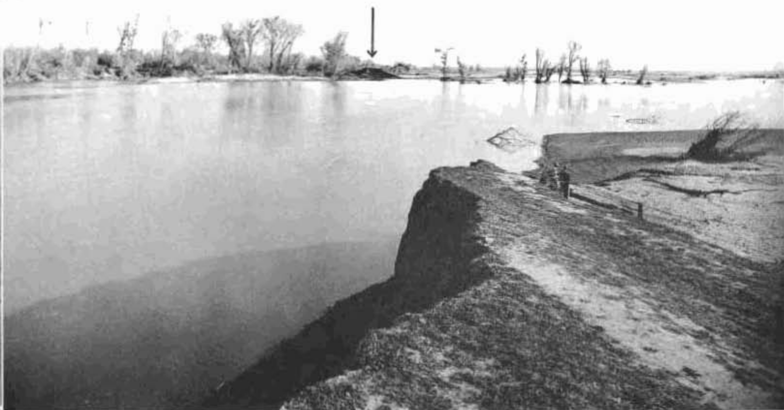
Break in Butte Slough Levee in Sutter County on March 1, 1940. Flood waters flowed through 1200 foot gap, inundating 35,000 acres of farm lands. Arrow marks far side of break.
