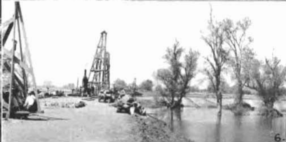
Construction views of timber and steel sheet pile emergency overfall dam in Butte Slough, 700 feet long with two wing levees. Total length, 1100 feet. 1—Bulkhead showing 3 drivers at work. 2—Final closing of steel piling. 3—Laborers wheeling cobbles for bottom protection in closure section. 4—Bulkhead showing steel piling. 5—Drivers at work on structure. 6—One of wing levees.
