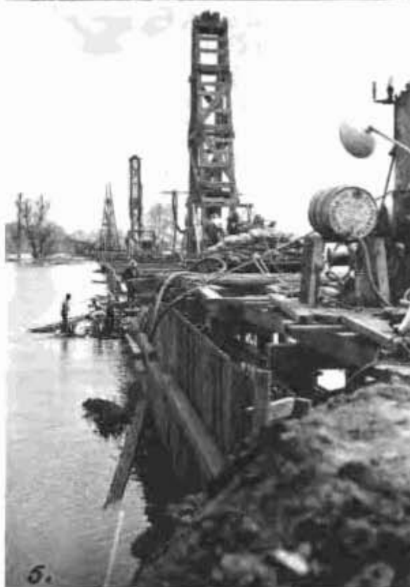
Construction views of timber and steel sheet pile emergency overfall dam in Butte Slough, 700 feet long with two wing levees. Total length, 1100 feet. 1—Bulkhead showing 3 drivers at work. 2—Final closing of steel piling. 3—Laborers wheeling cobbles for bottom protection in closure section. 4—Bulkhead showing steel piling. 5—Drivers at work on structure. 6—One of wing levees.
