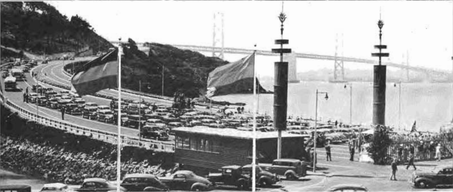
At top—Treasure Island showing how the Golden Gate International Exposition is reached via the San Francisco-Oakland Bay Bridge. Below is a portion of the 6-lane State-built ramp approach. At bottom—Automobiles waiting for the gates to open early on the first day.
