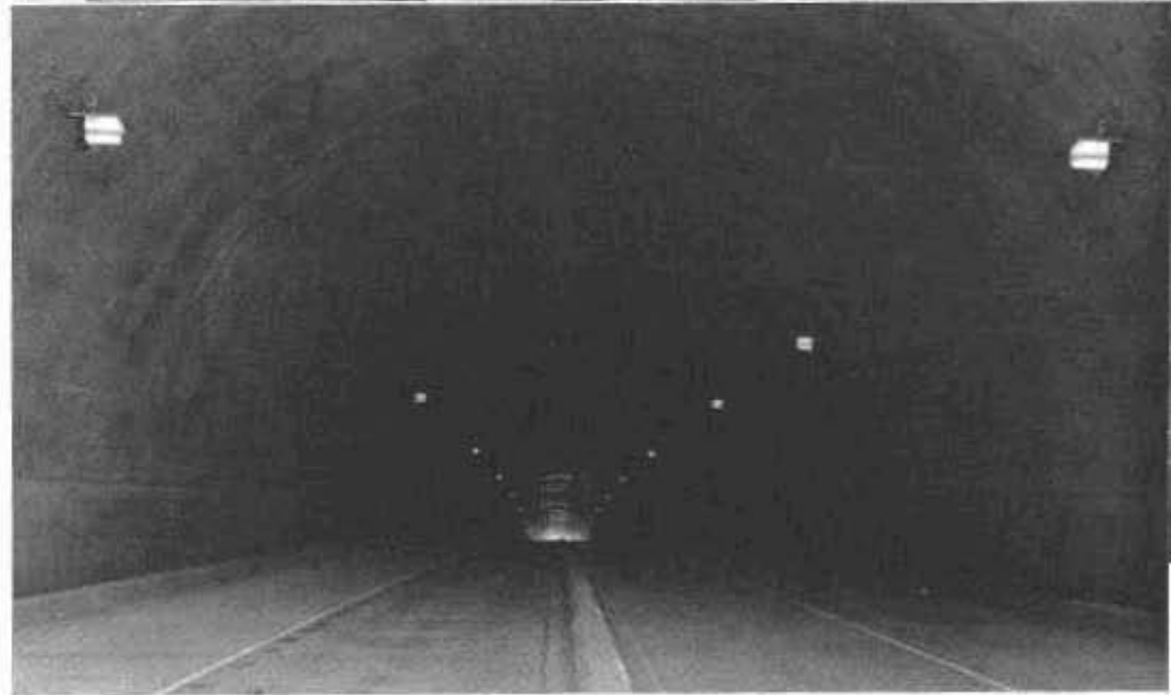
Upper—Traffic starts over Funston Avenue Approach. Lower—View of tunnel under golf course in U. S. Presidio.
