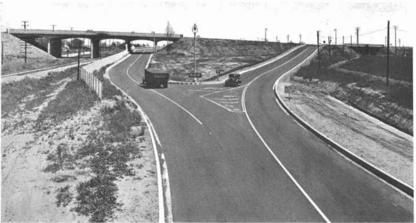
Pomona grade separations. Southern Pacific underpass on left. Top of Union Pacific underpass can be seen in right background.
