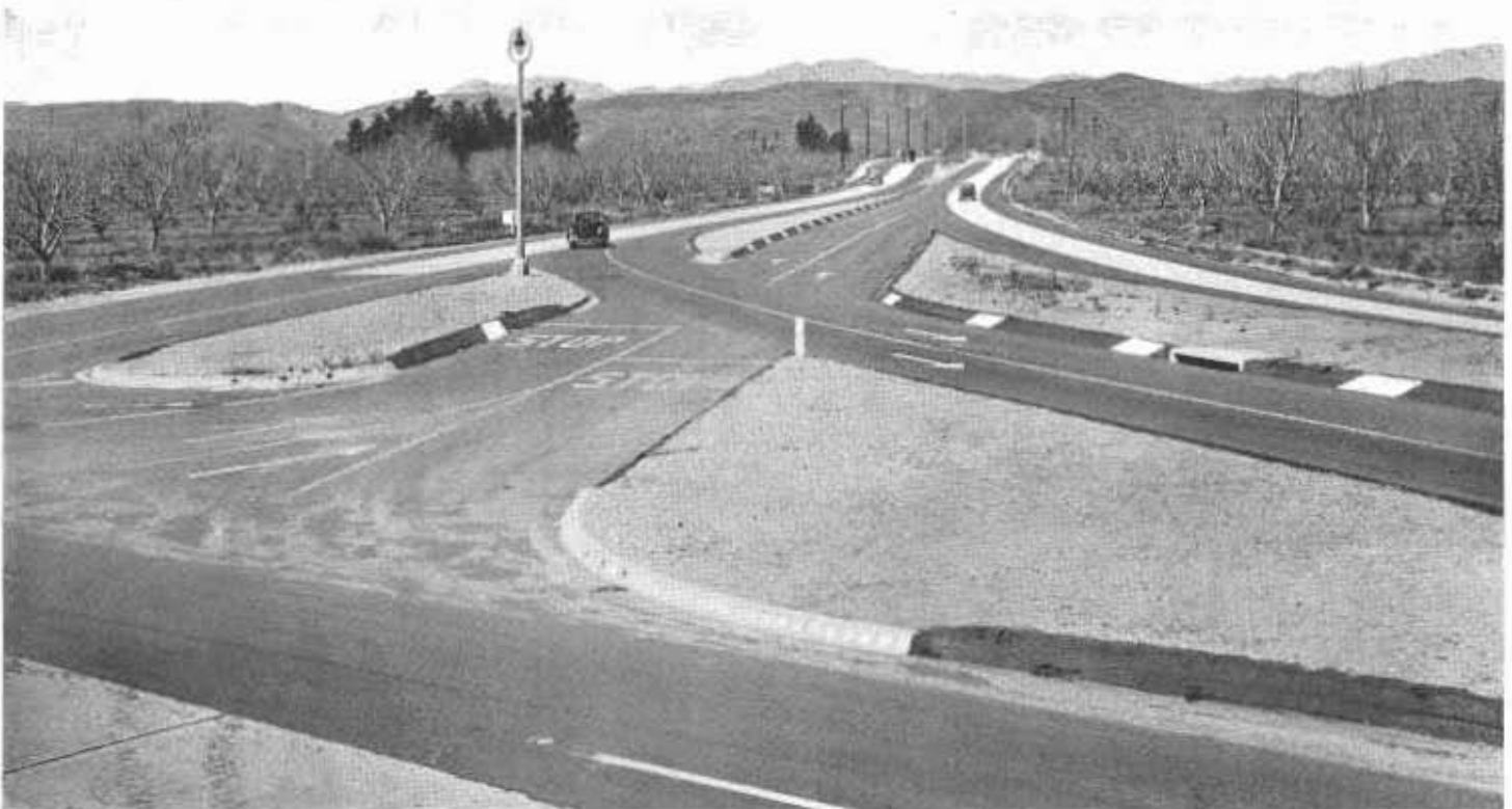
South channelization of approach to Pomona grade separations. Highway Route 19, Pomona to Fullerton, in foreground.
