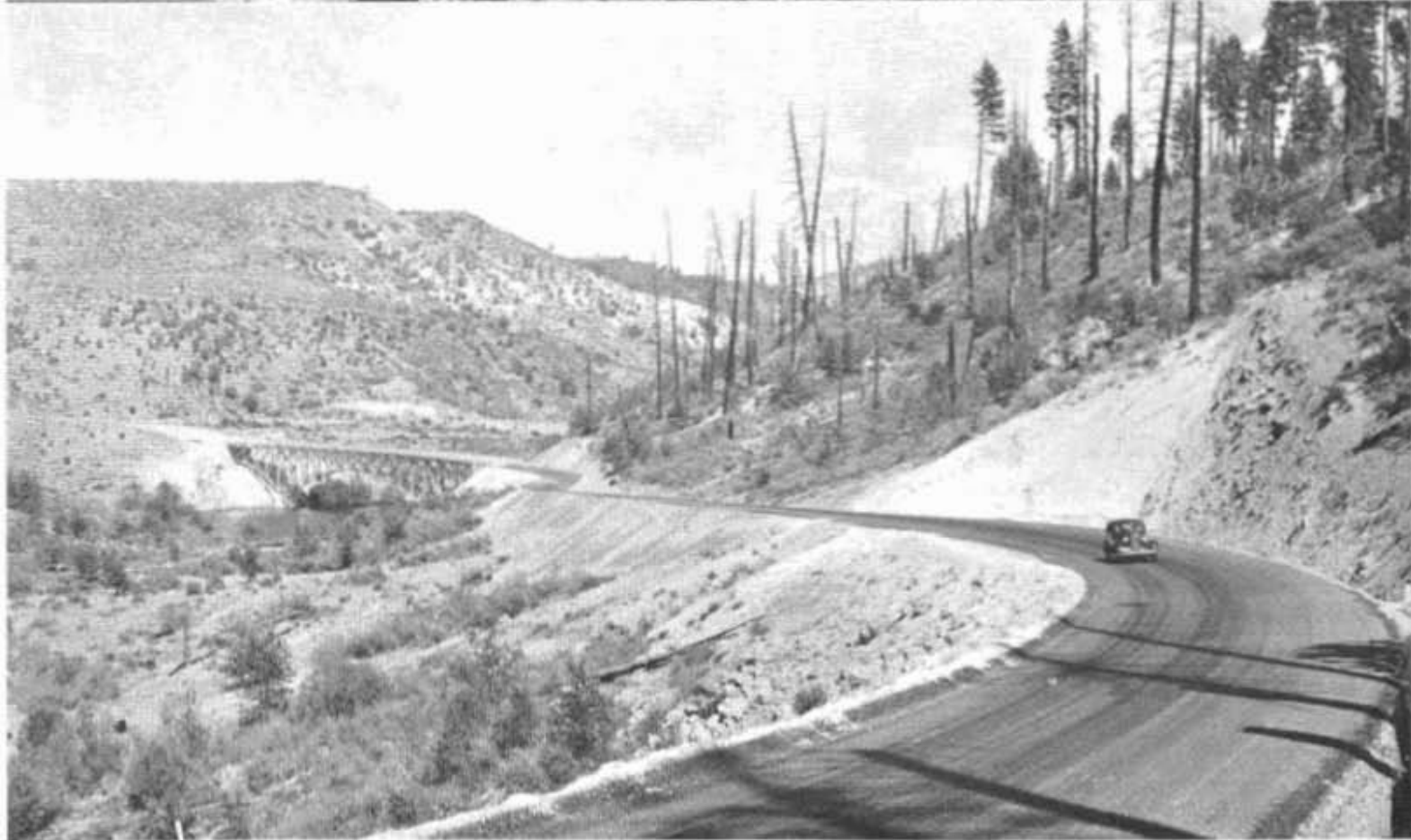
Upper—New bridge across Lake Britton. Lower—Looking northwesterly down grade towards Pit River Bridge across Lake Britton
