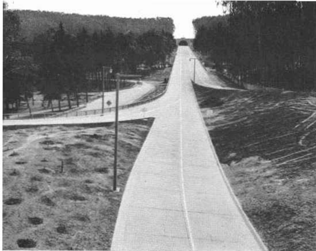
Funston Avenue Approach, tunnel in distance, before being opened to traffic.
