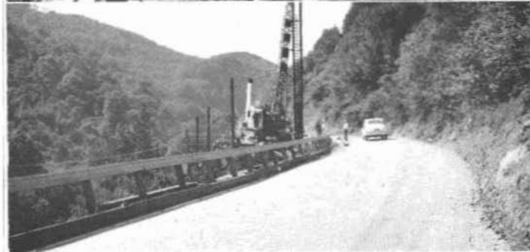
Views showing viaduct pile driving operations. Completed roadway will be 50 feet wide.
