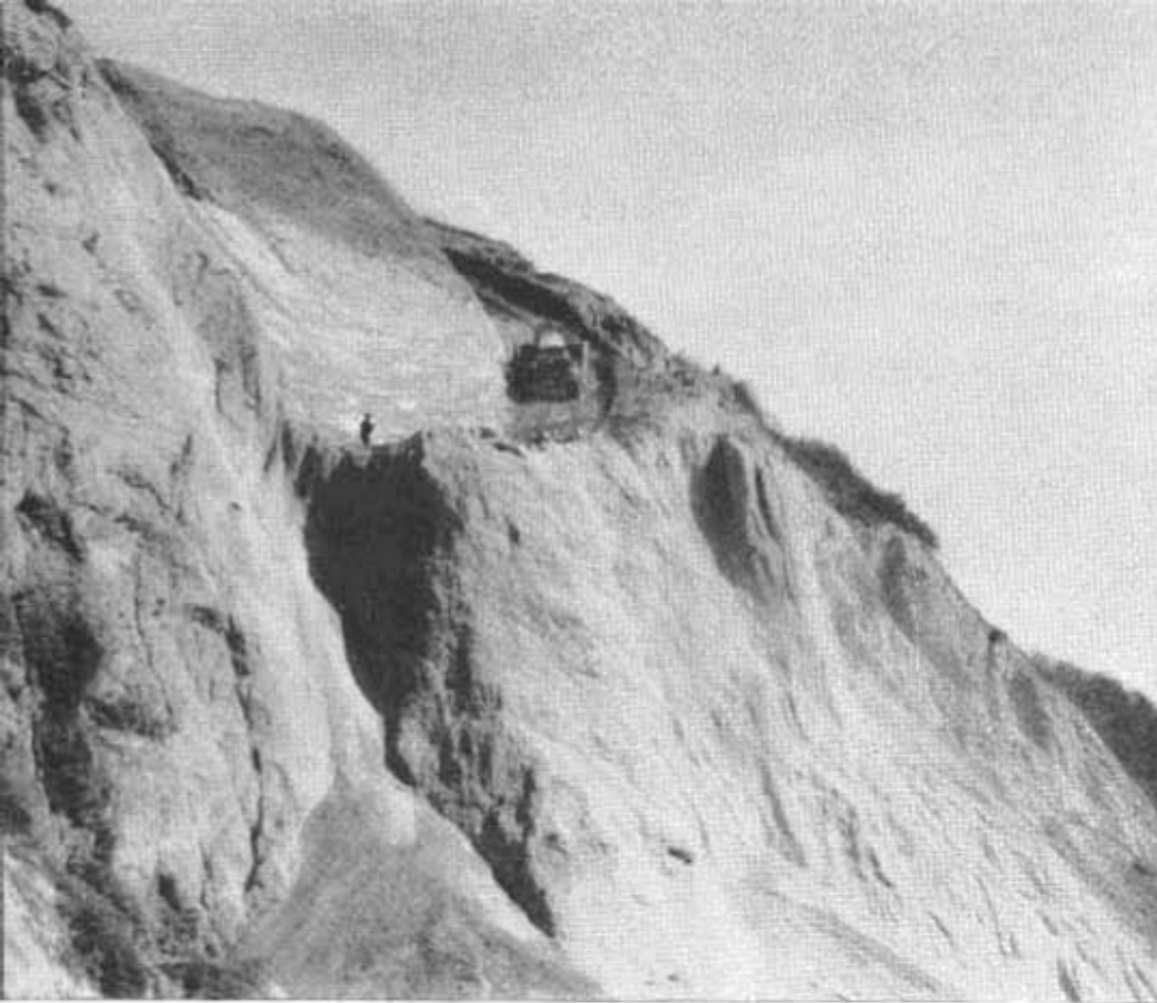
Clearing summit of Santa Monica Palisades of dangerous slide material
