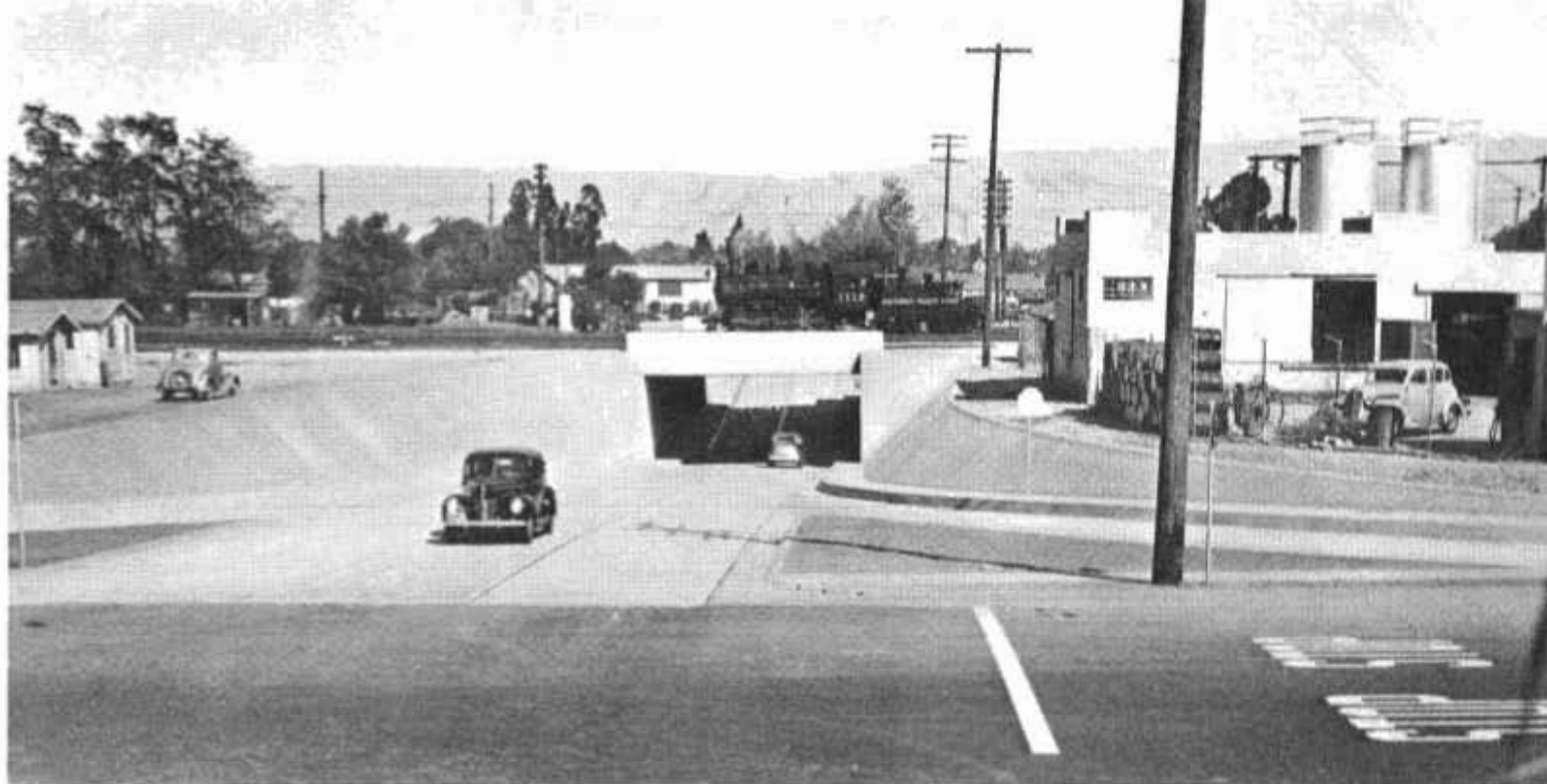
New Polhemus Street underpass in San Jose eliminating dangerous railroad grade crossing on heavy traffic highway arterial
