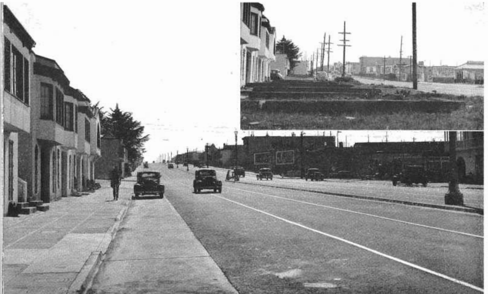
Views on Nineteenth Avenue, San Francisco, before (upper) and after (lower) widening of pavement and setting back of residences
