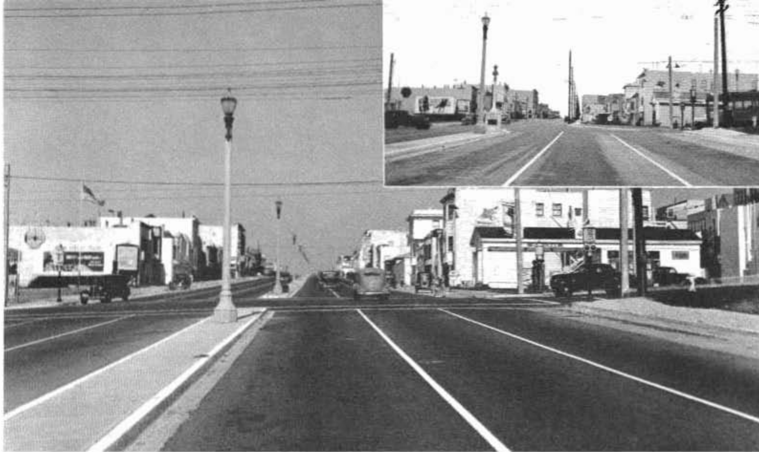
Looking north on Nineteenth Ave. across Taraval St. in San Francisco before (upper) and after (lower) thoroughfare was widened
