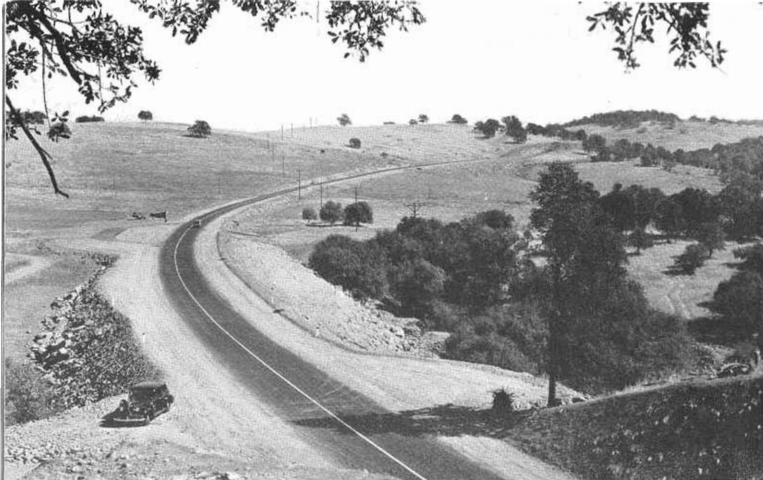
Looking up new Clarksville grade on the realignment of U. S. 50 between Folsom and Placerville
