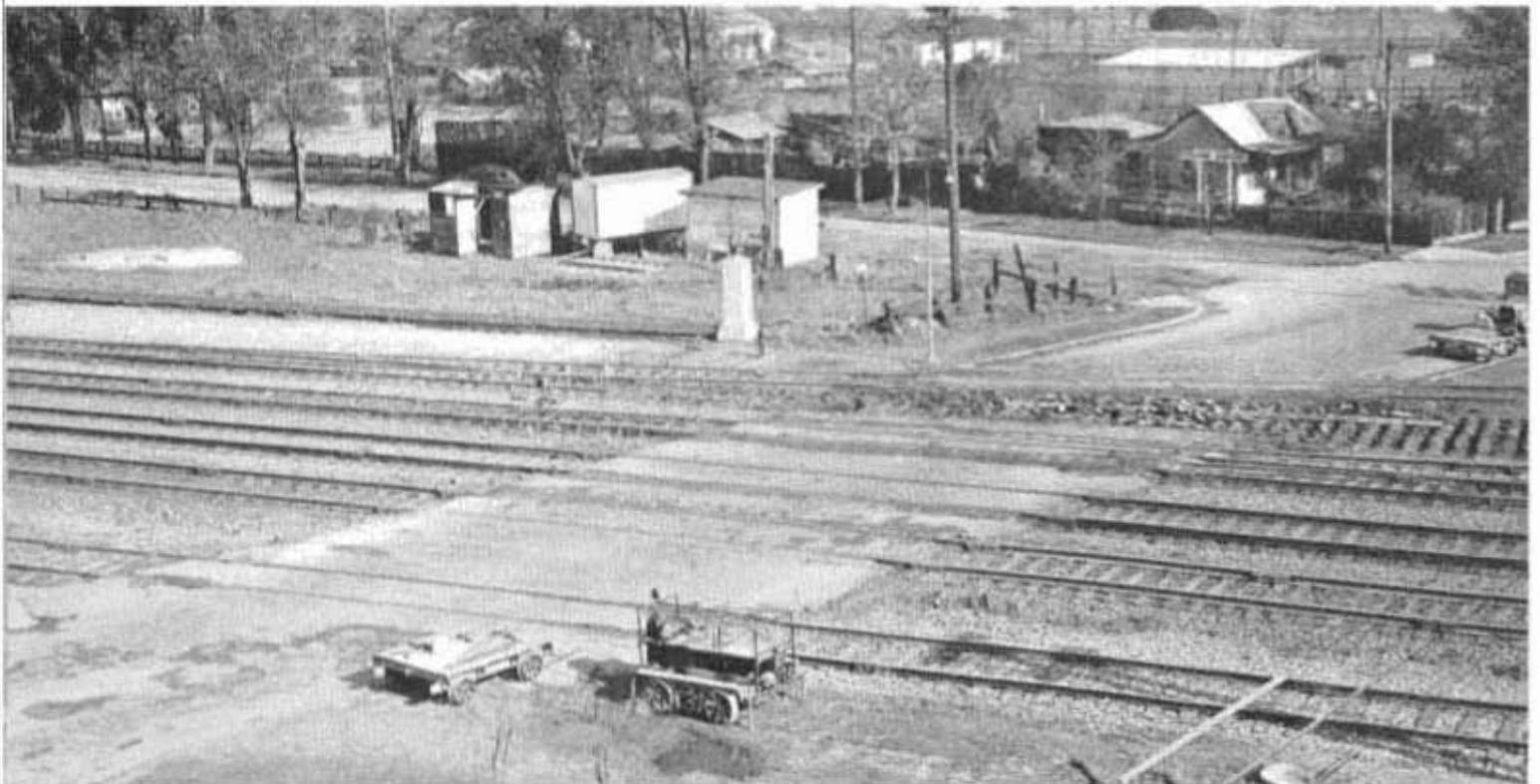
View of Polhemus Street Crossing in San Jose before improvement where highway crossed nine tracks used by eighty trains daily
