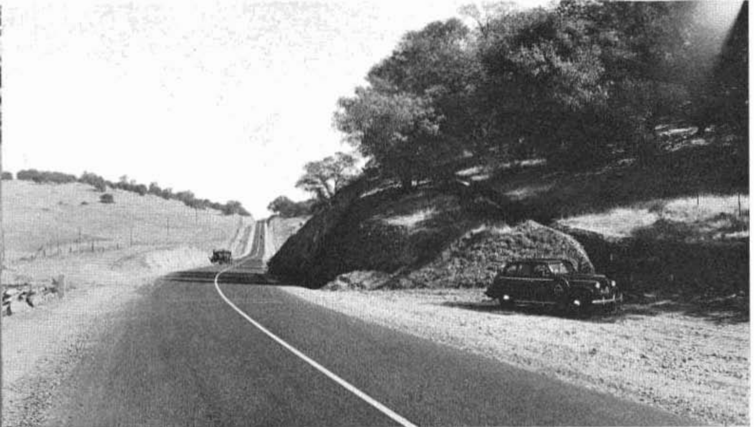
East of Clarksville the new straight route, eliminating numerous sharp curves, affords excellent sight distance
