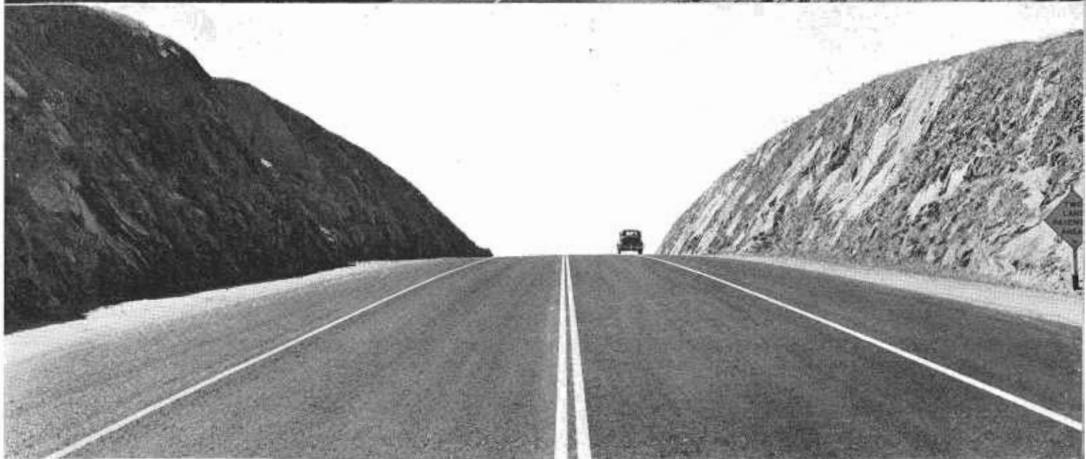
Top and bottom pictures of U. S. 50 realignment east of Folsom show where 4 lanes were provided to enhance safety on vertical curves. Center picture is view of a cut through solid rock where blasting was necessary
