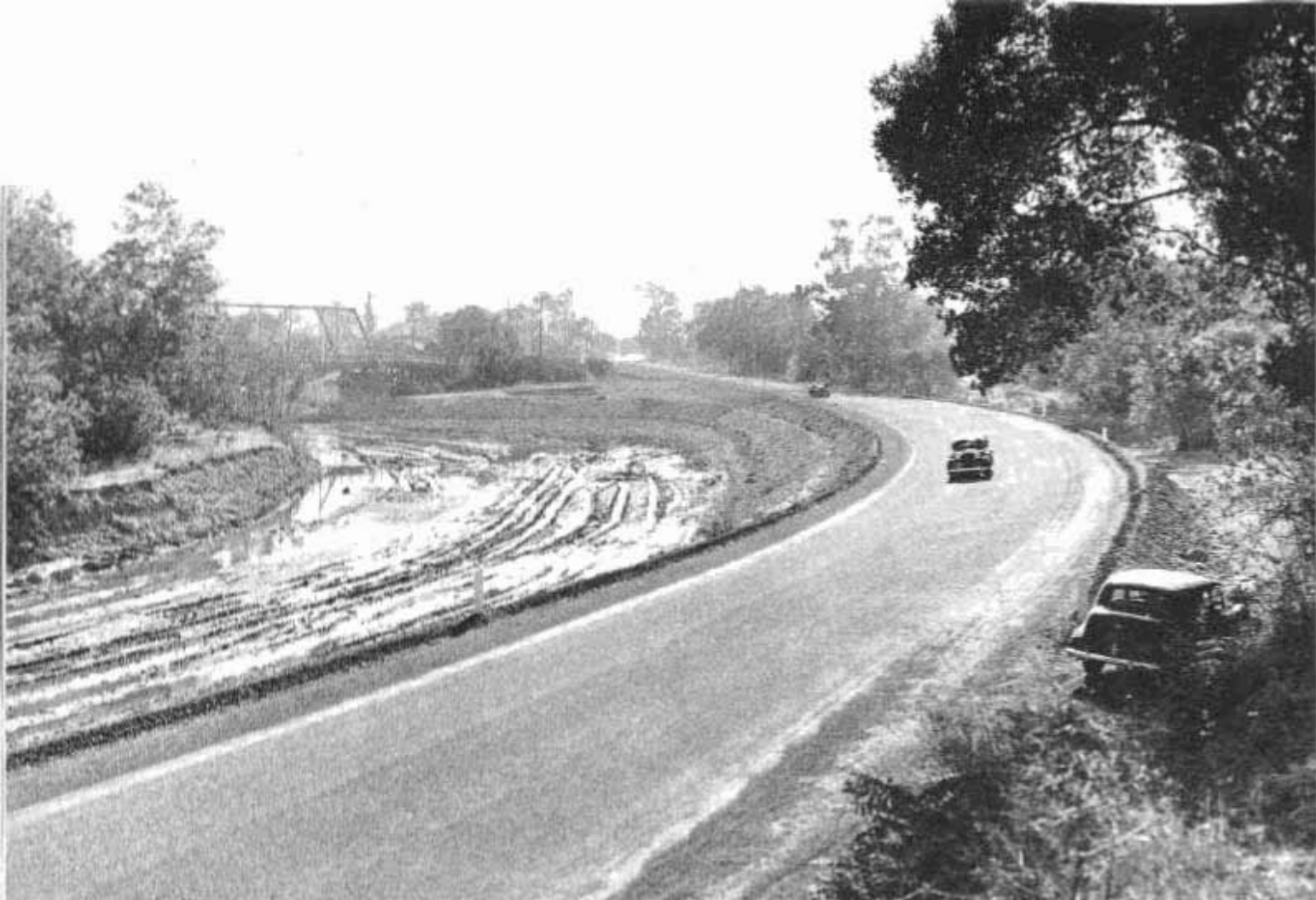
View of Niles Canyon showing new highway around relocated stream bed and one of two bridges eliminated by new alignment
