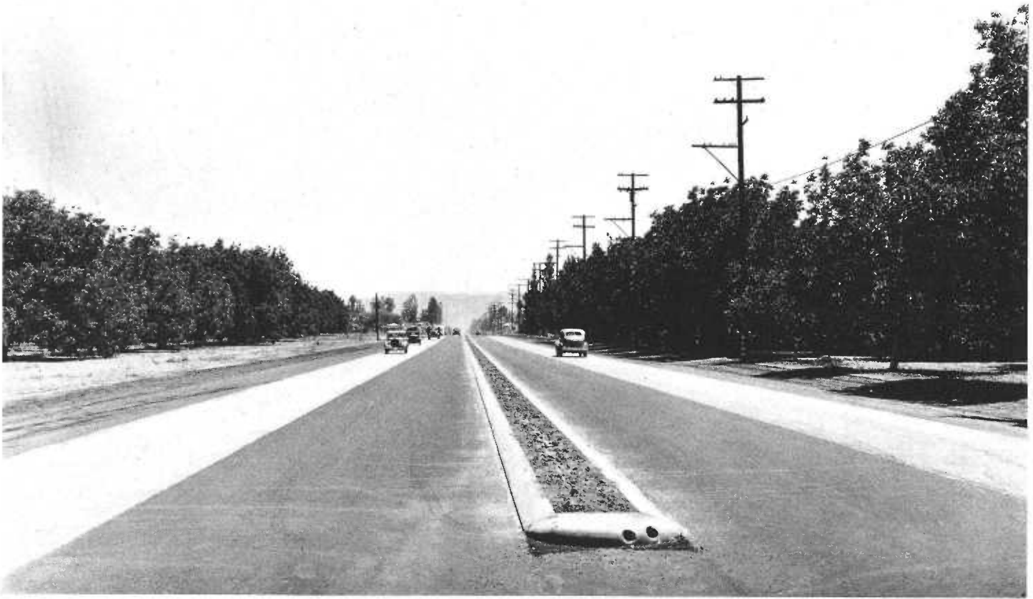
Section of Sepulveda Boulevard reconstructed as a divided highway with 4-foot center dividing strip with 5-inch P. C. curbs
