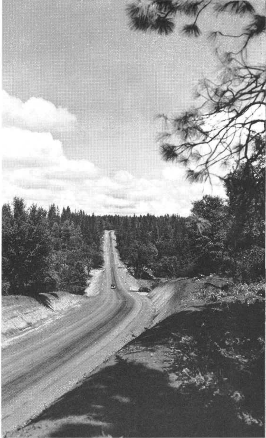
New alignment has 5 curves compared with 35 on old road
