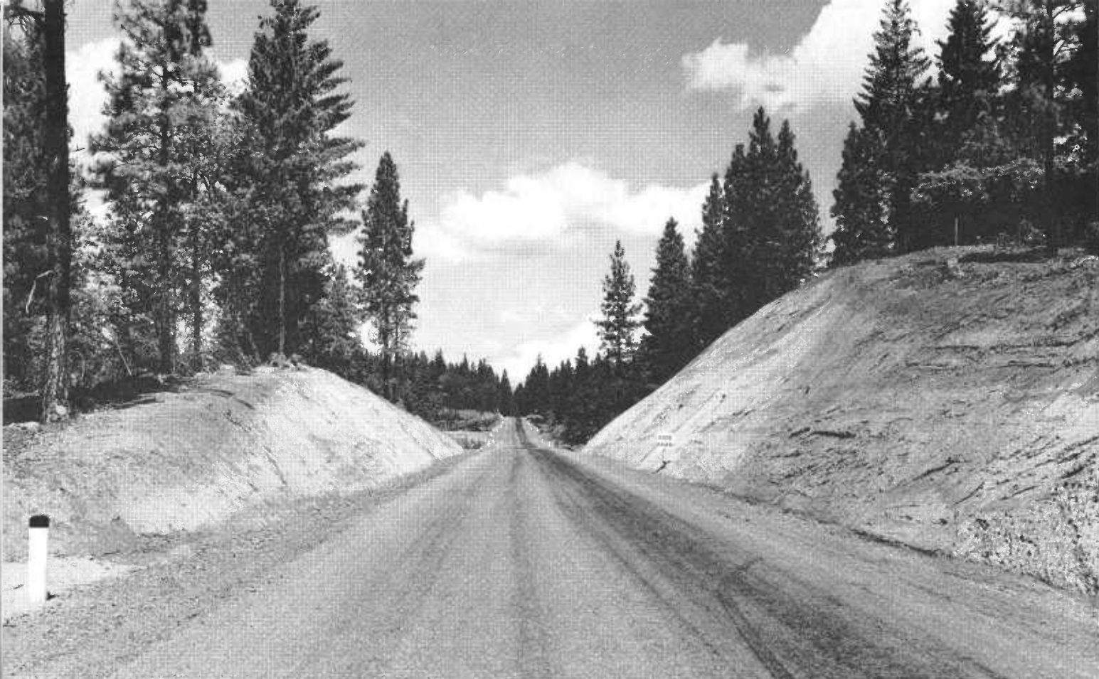
Section of recently improved State Highway No. 17 in Nevada County on new alignment eliminating many curves
