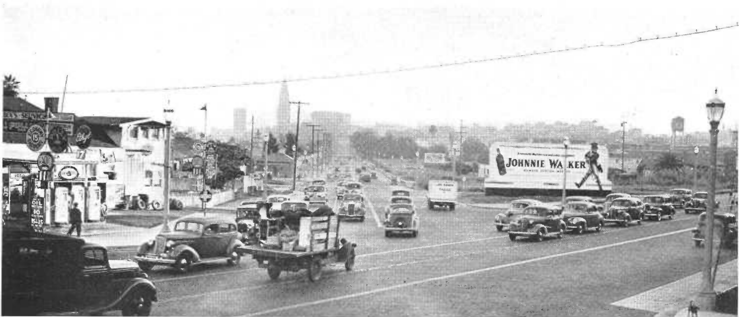
At top and bottom—Views looking southerly along Castelar Street showing interference of late afternoon traffic on North Figueroa Street by reason of southbound traffic on Figueroa Street making left turn into Castelar Street. This condition will be eliminated by a grade separation on proposed extension route
