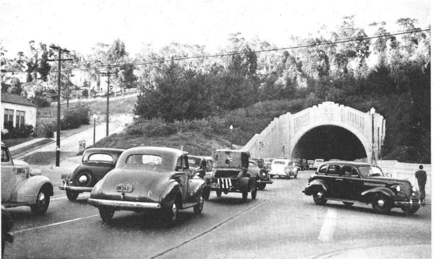
Traffic through North Figueroa Street tunnels meets cross traffic at Solano Street intersection
