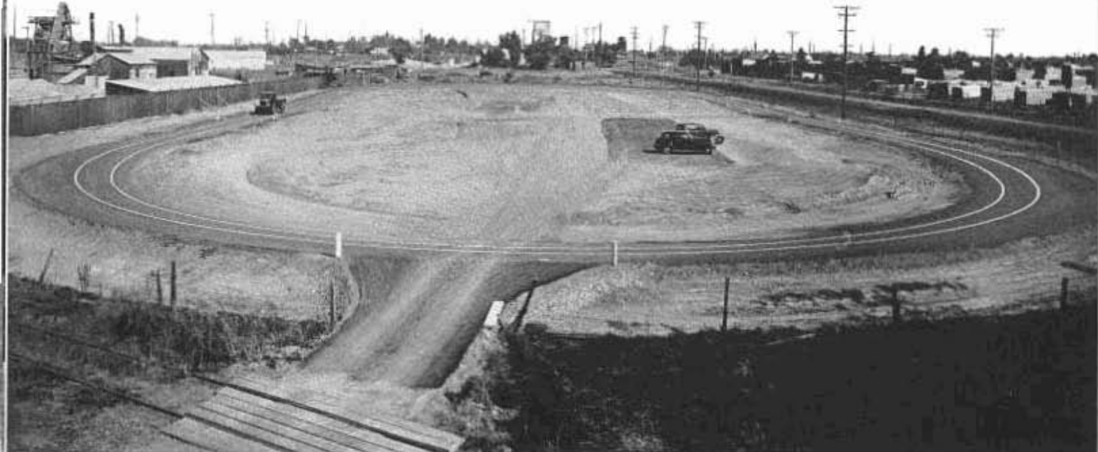
General view of oval track for testing highway construction material and surface mixtures to destruction under heavy truck traffic.
