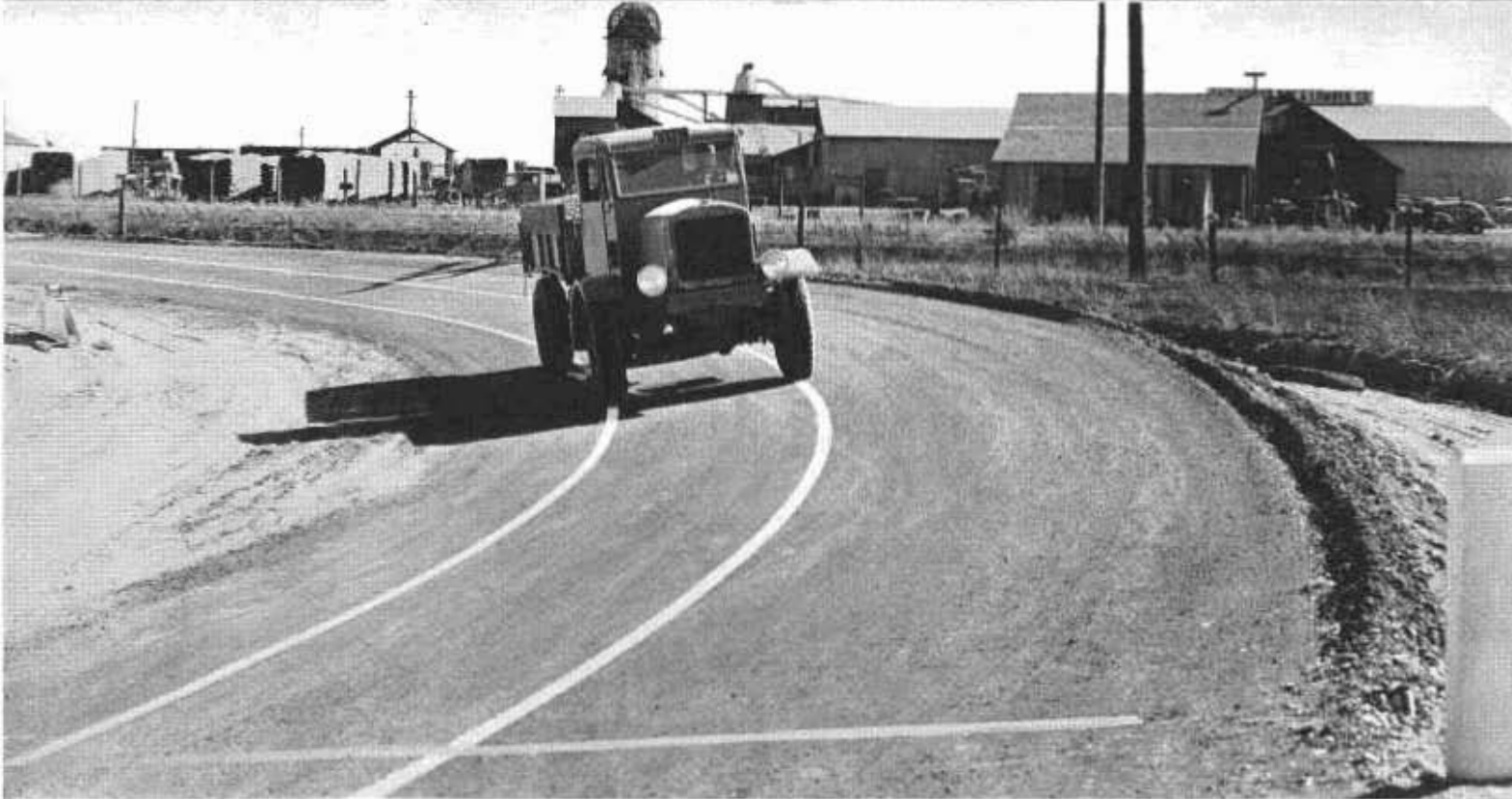
Above—Test track straightaway with 8 test sections of treated material. Below—Superelevated curve surfaced with bituminous mixtures.
