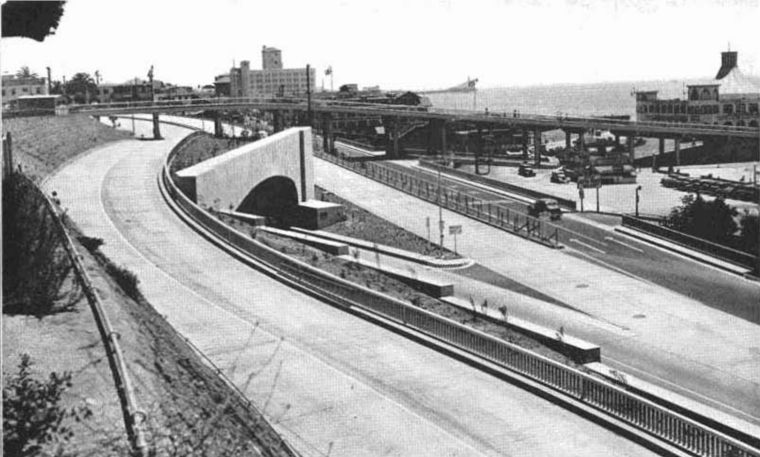
View of Coast Highway tunnel, ramps and overhead grade separation structure at Colorado Avenue intersection in Santa Monica.
