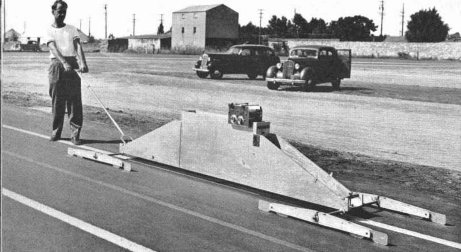
Roughometer designed and built at the Division of Highways laboratory for measuring roughness of pavement surfaces.
