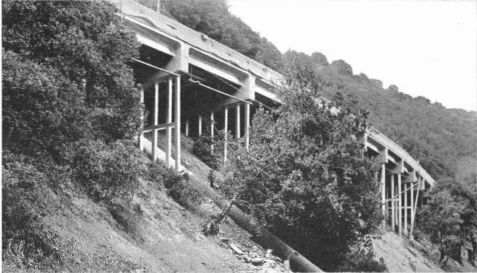
Two views of sidehill viaduct on Los Gatos-Santa Cruz 4-lane highway. Top picture shows how two lanes are carried on viaduct built on curve. Bottom picture shows steel piling and character of construction supporting the highway.
