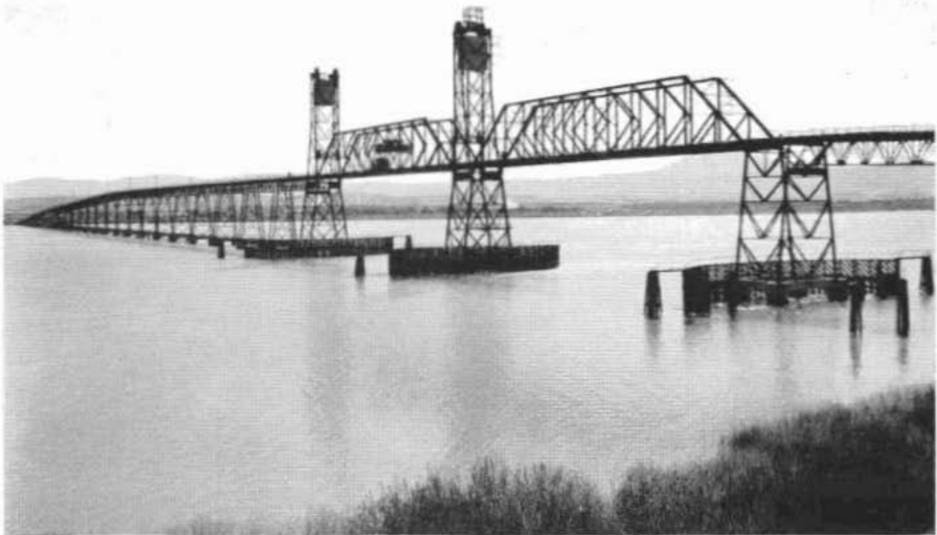
Antioch Toll Bridge across the San Joaquin River on State Highway Route 11 near Antioch, purchased by the State.
