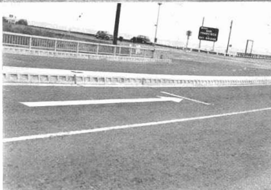
At top—Traffic actuated signal on East Shore Highway (U. S. 40) at Berkeley. Car in foreground has crossed pavement detector and is entering intersection. At bottom, arrow points to signal control treadle or traffic detector which is operated by wheel of car passing over it.
