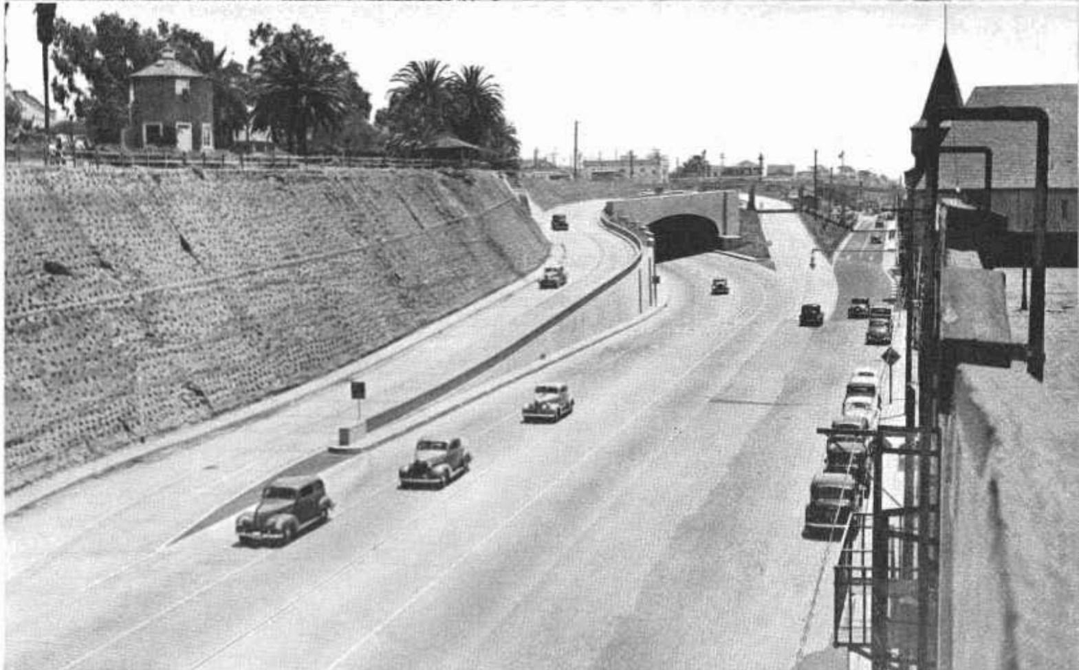
At top—Overhead structure across 4-lane Coast Highway at Santa Monica. Below—Tunnel and ramps at intersection with Appian Way.
