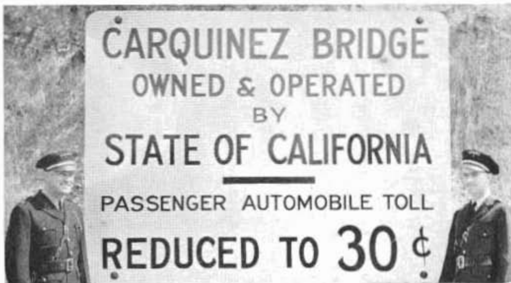
Sign announcing State-owned bridge and reduced toll price.
