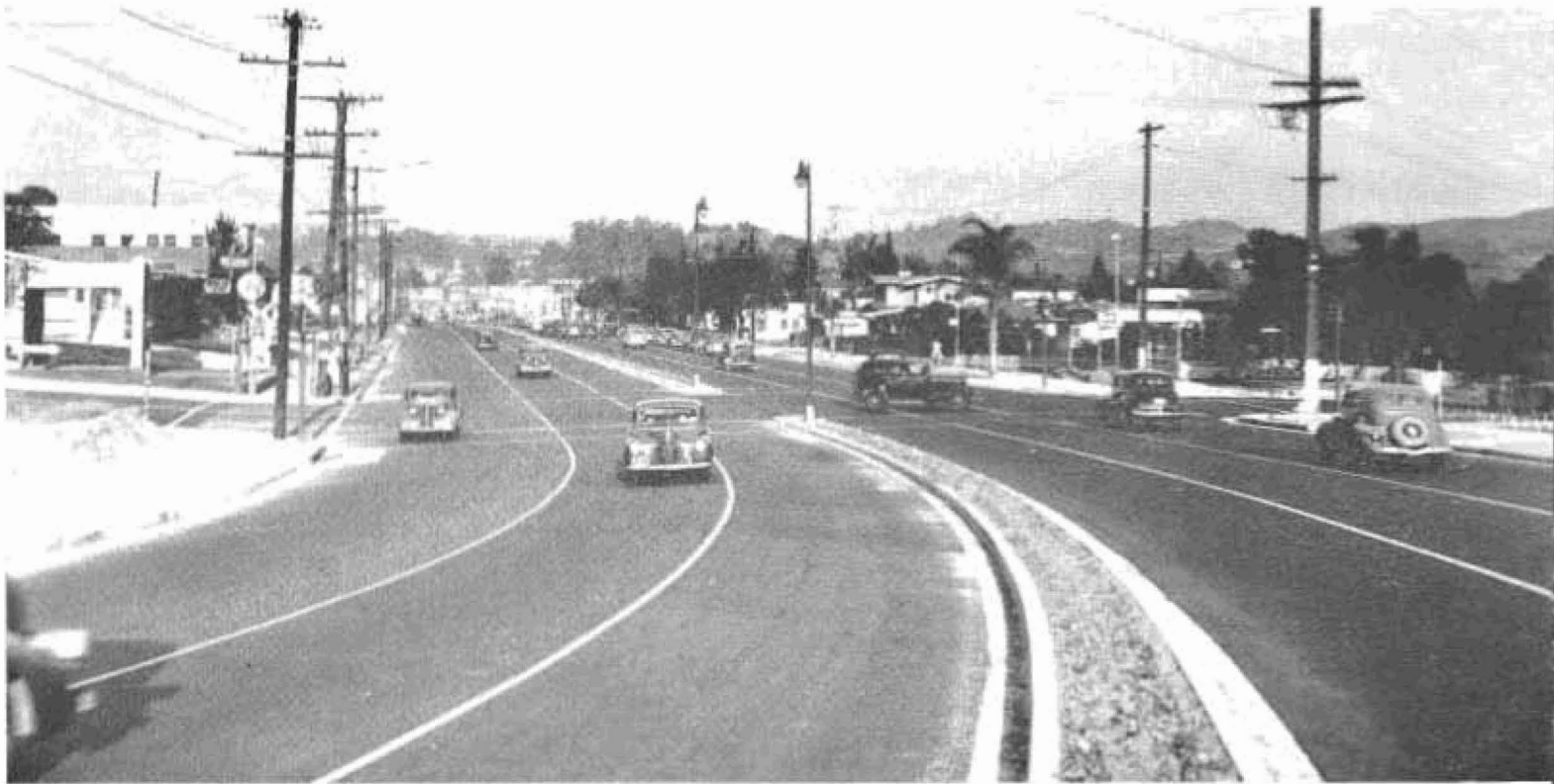
Colorado Blvd. Divided Highway in Los Angeles County paved with 2-inch asphaltic concrete on 6-inch Portland cement concrete base
