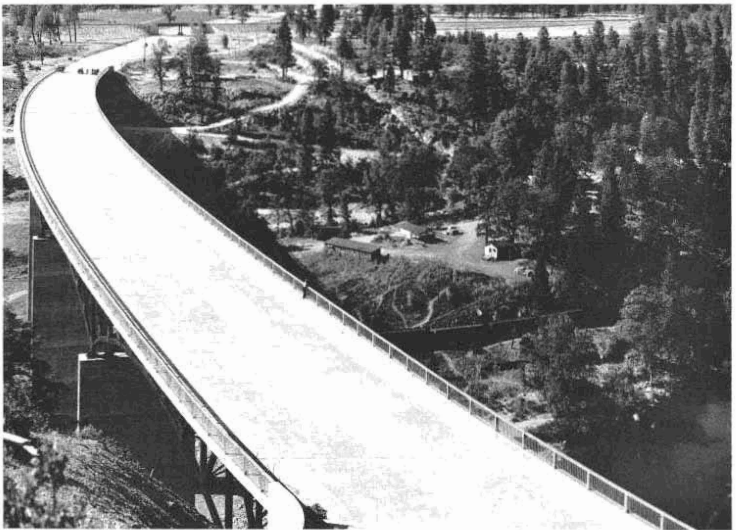
View of 50-foot roadway of Antler Bridge built on 850-foot radius curve to carry relocated 4-lane divided highway
