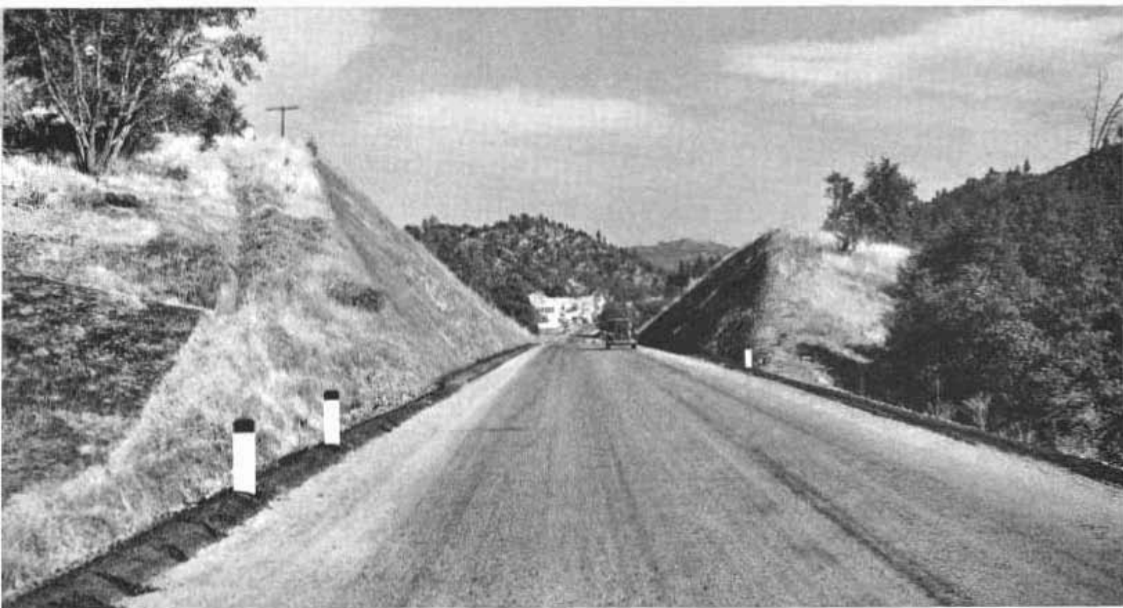
New All-Year Yosemite Highway relocation goes straight through Mariposa obviating right hand turns of old route on city streets
