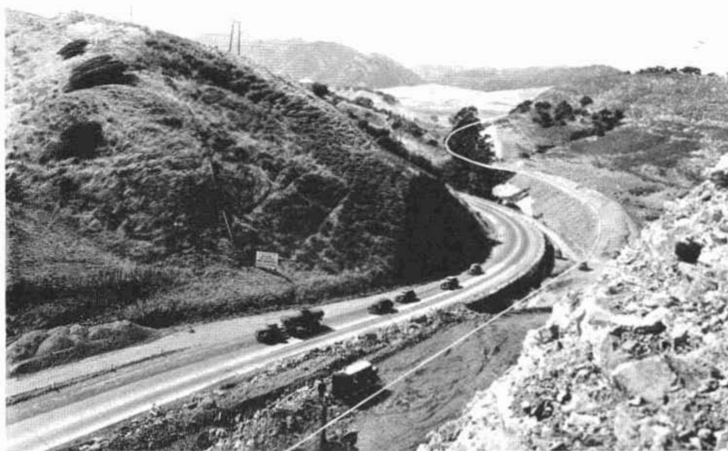
Scenes on realignment construction of U. S. 101 south of San Luis Obispo. Top picture shows bridge being built and rough grading near San Luis Obispo Creek. Below—White line indicates new route compared with existing grade
