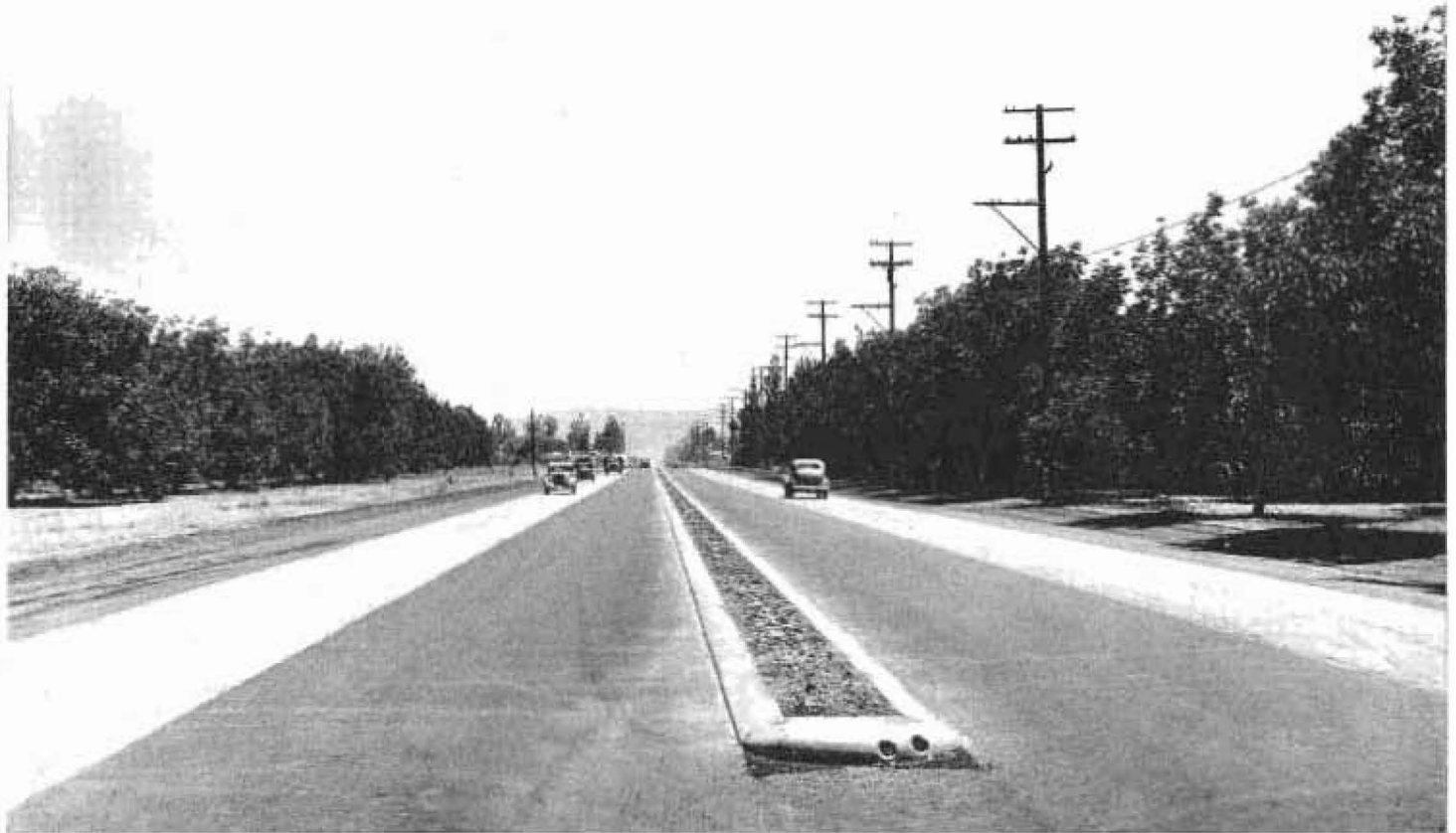
Sepulveda Boulevard in Los Angeles has two 17-foot lanes of asphaltic concrete and two 12-foot lanes of Portland cement concrete
