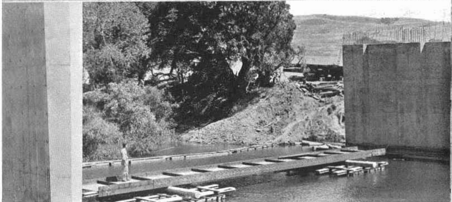
At top—Existing narrow bridge across Pajaro River. Center—Three wide concrete piers ready for steel erection. At bottom—Large steel girder floated into position on rafts preparatory to raising with power crane
