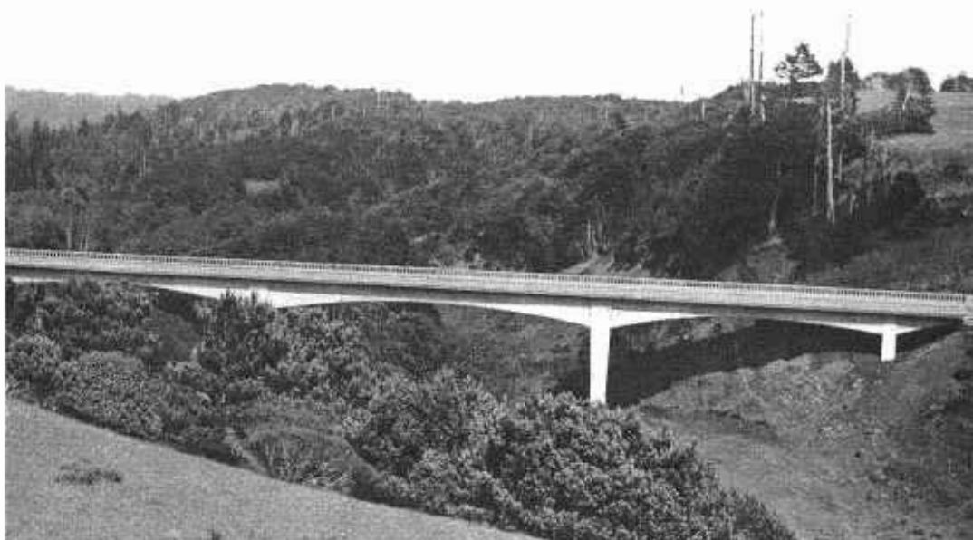
Side view of Schooner Gulch bridge shows simplicity of design
