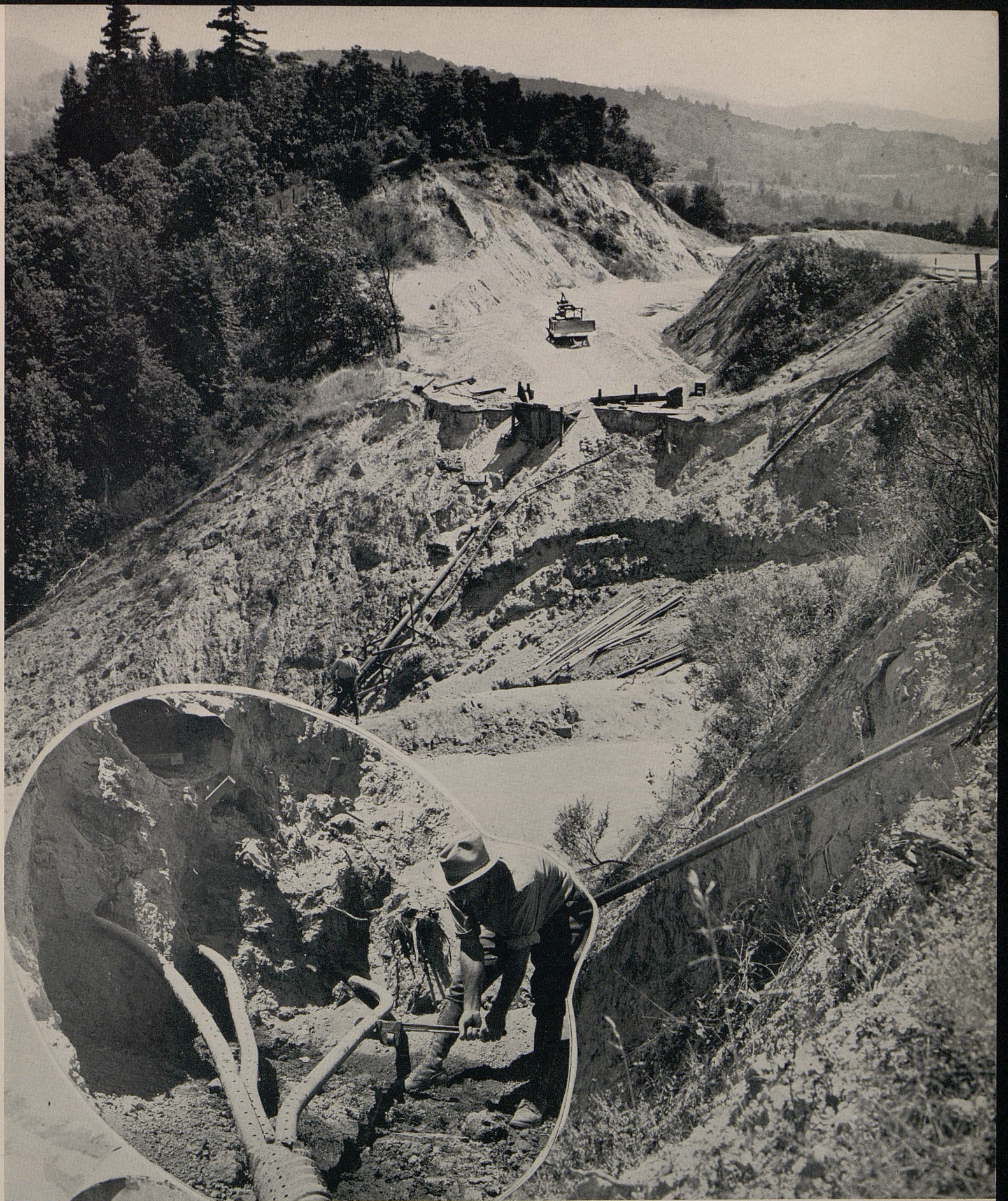
View of large slipout of fill. Installation of extensive drainage system under way. Inset shows outlets of 2-inch perforated pipe drains before covering with crushed rock.
