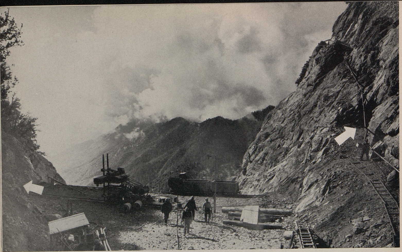
Arrows point to 2 tunnels separated by only 87 feet of highway being bored through Mt. Williamson on Angeles Crest Highway.
