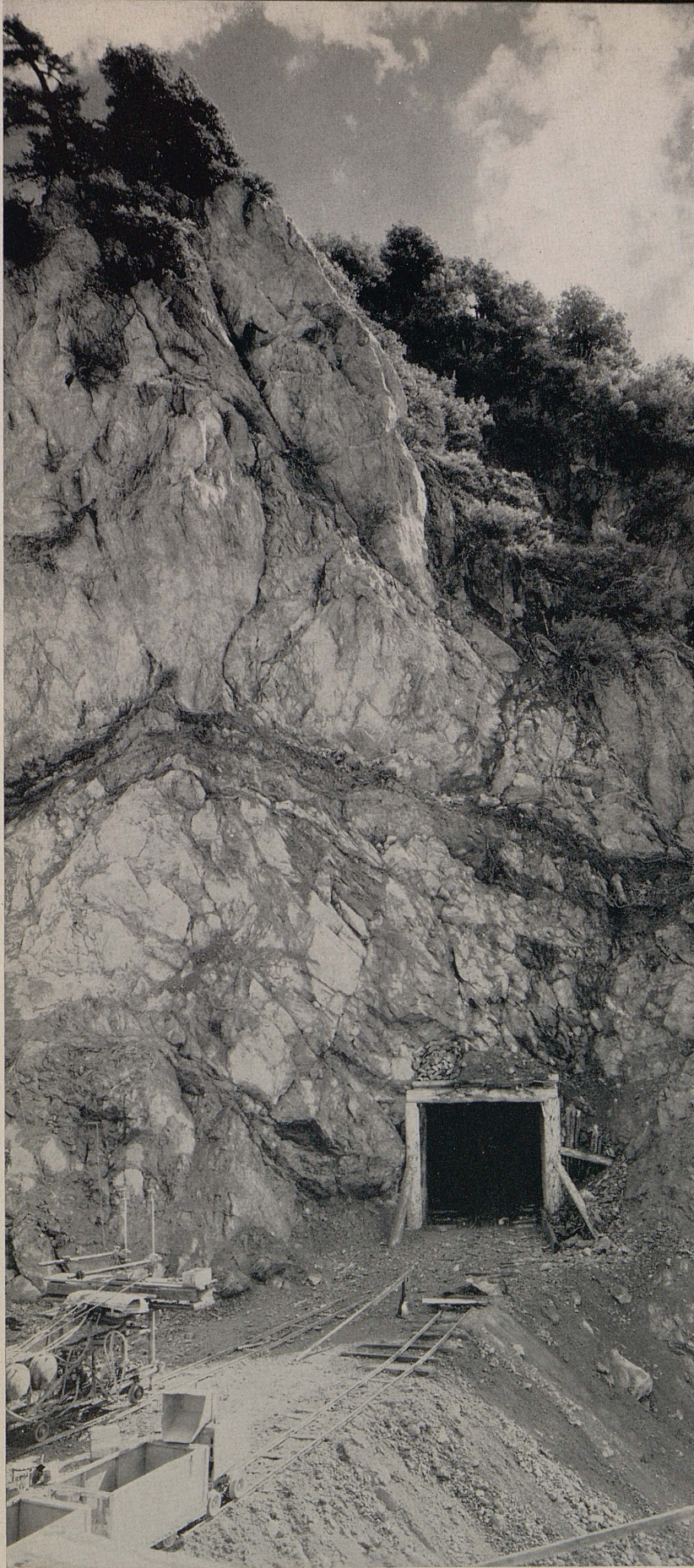
At left, portal of tunnel No. 2 through ridge of Mt. Williamson. This is a 14 x 14 foot pilot bore. At right, top, equipment mucking at main heading of tunnel No. 1, showing protective shell in use. Below, Construction yard between tunnels. Building concrete tunnel lining form. In the background may be seen the portal of tunnel No. 1.
