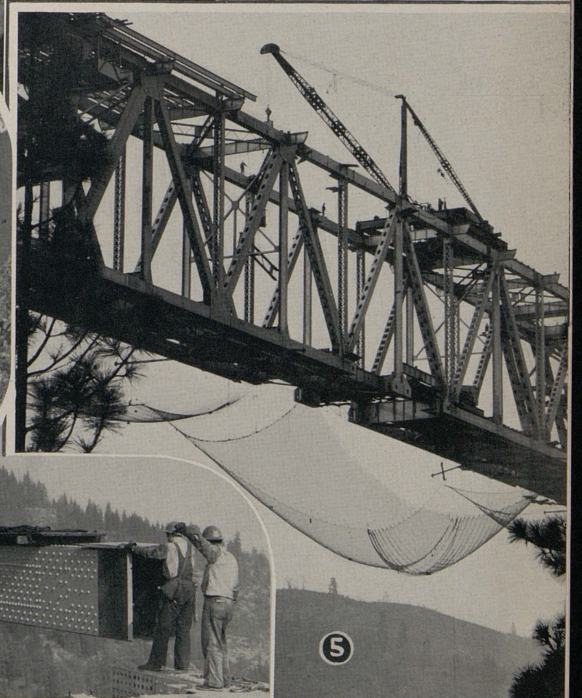
Connecting the last span: (1)—Pit River Bridge workers suspended on platform 500 feet above river ramming home 5-ton riveting pin. (2)—View of pin coming through girder. (3)—Arrow shows pin in place. (4)—Lowering connecting girder into position. (5)—Last span connection complete.
