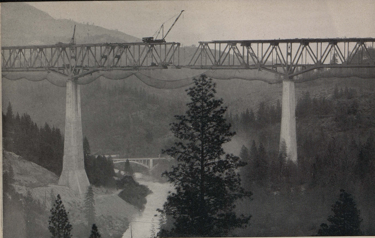
View of Pit River Bridge taken just as the central span was being placed connecting up the world's highest double deck structure.
