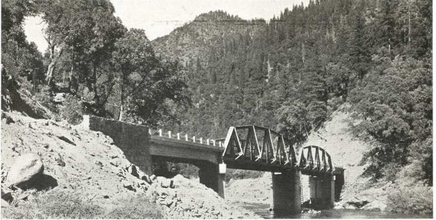
A bridge on high speed alignment at a favorable location but nevertheless it had to be skewed and super-elevated
