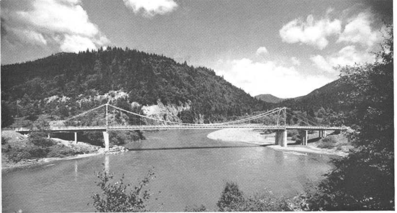
Bridge across Klamath River winner of national award for most beautiful steel bridge costing less than $250,000 built in 1940
