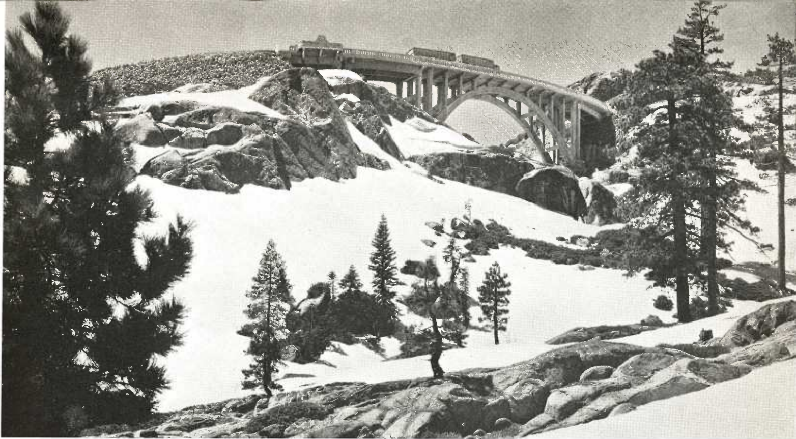
A "dry land" bridge on a summit used in place of a more expensive fill with retaining walls
