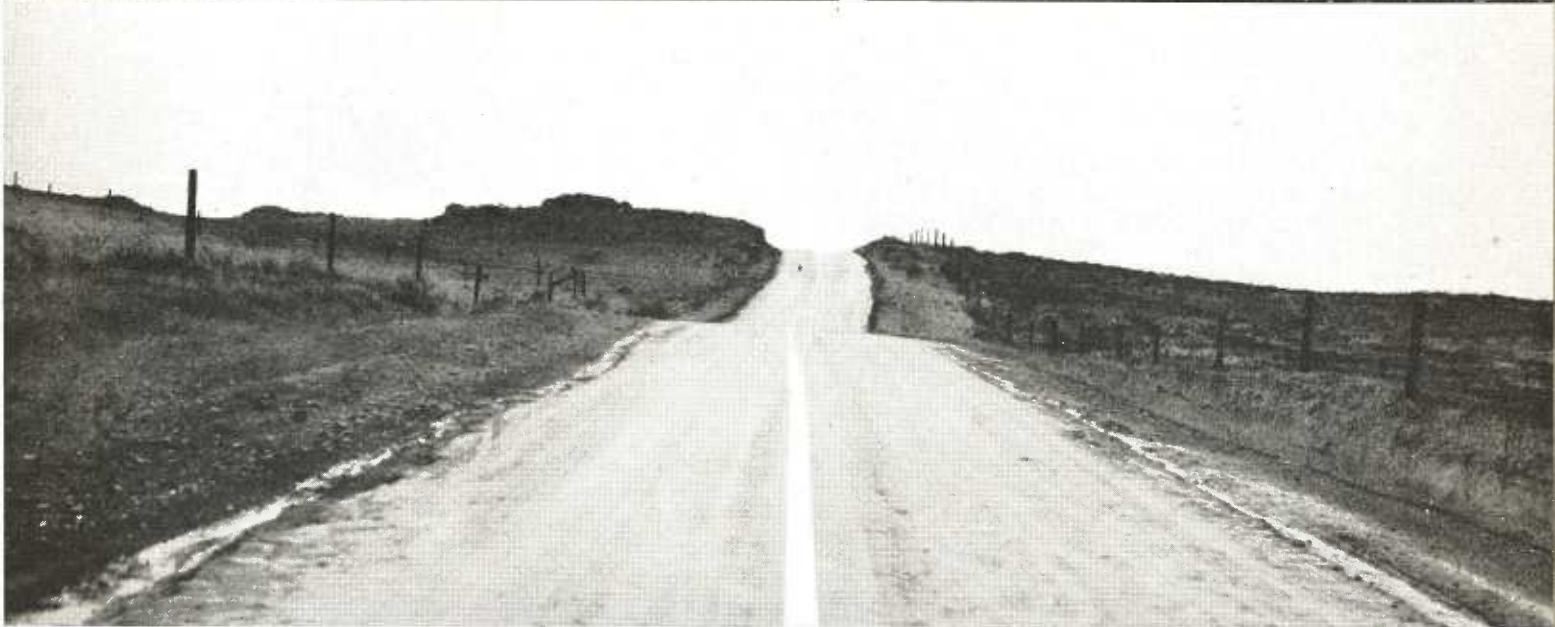
At top—Cottonwood Creek bridge on new Madera-Friant highway. Center—Long, straight stretches with perfect visibility are typical of the new highway. At bottom—Narrow road before reconstruction was a series of sharp vertical curves
