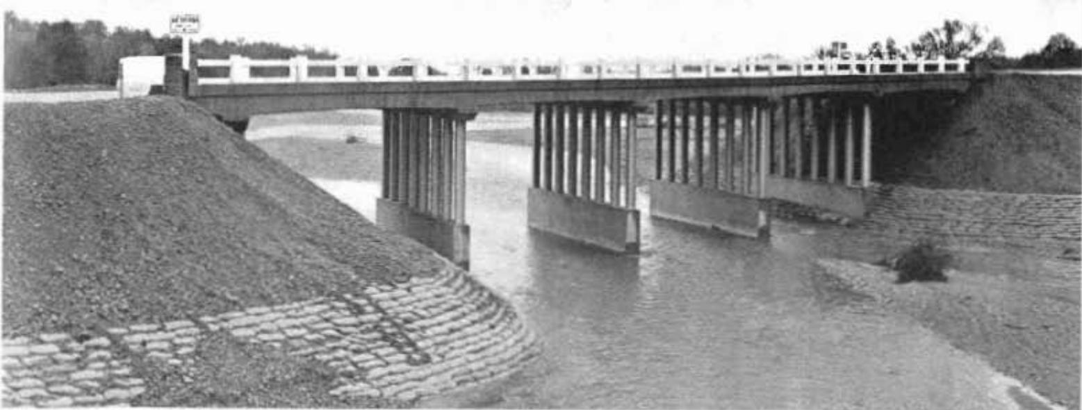
Six mile relocation of U. S. 99 north of Red Bluff just completed includes a 160-foot concrete slab bridge on steel piles across Dibble Creek and a 135-foot bridge of same type across Blue Tent Creek shown in top and bottom photos
