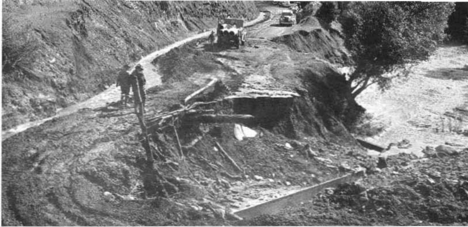
Washout on U. S. 299 West of Redding caused by February storms. Large sections of pavement were destroyed by undermining waters
