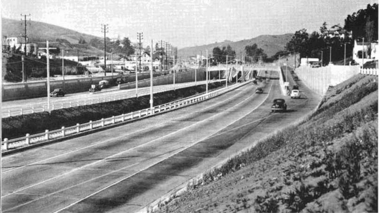
New section of Cahuenga Pass looking north toward Barham overpass, showing two 4-lane highways separated by railroad tracks with ramps to service roads
