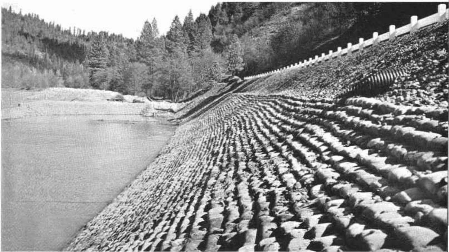
The above pictures show portions of 25 acres of sacked concrete slope paving placed on the banks of Trinity River for protection of the highway at flood stages. A total of 148,029 sacks was laid, approximately one sack per square foot.
