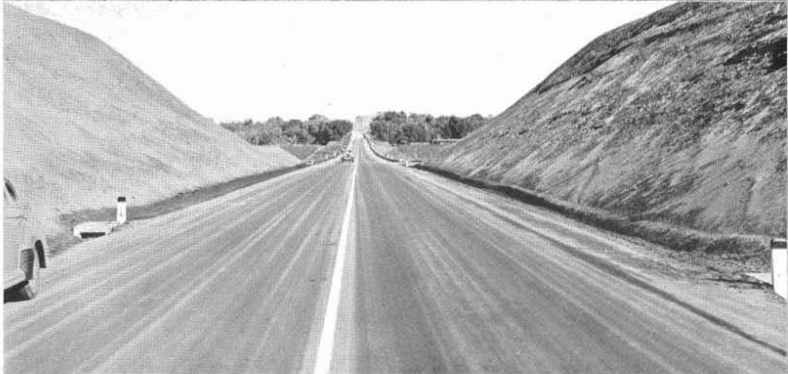
Top and bottom pictures show sections of revised alignment on State Highway between Fresno and Yosemite Valley. Center—Reinforced concrete bridge over San Joaquin overflow connected with Lanes Bridge by 255-foot fill. The bridge is 200 feet long
