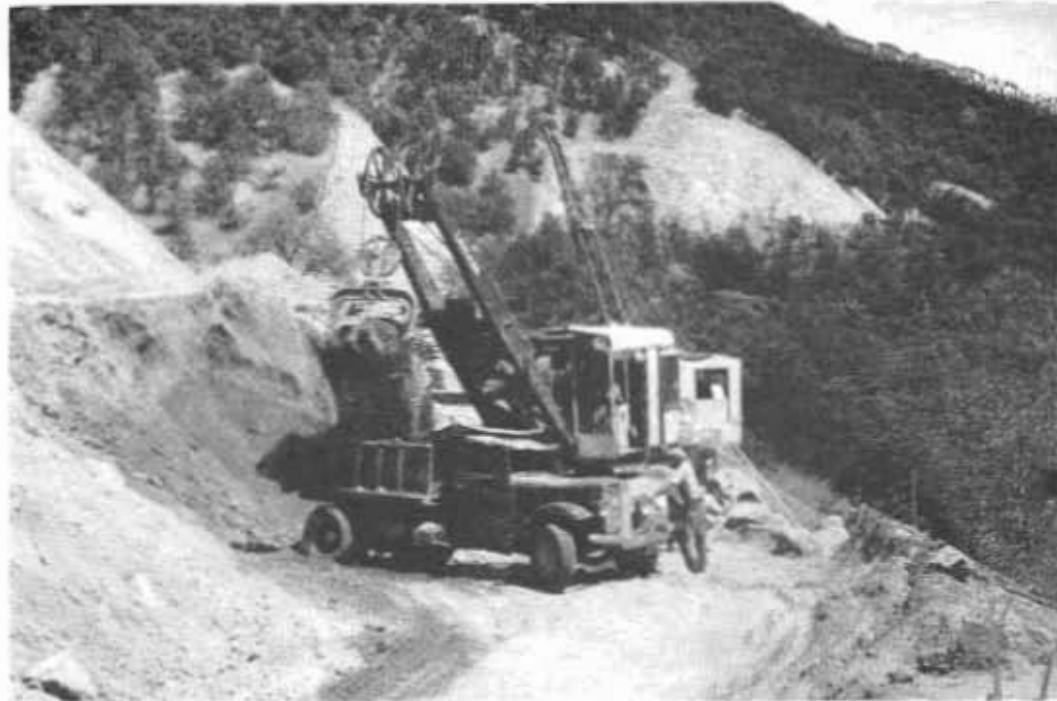
Shovel and trucks completing construction on Kings River Canyon unit
