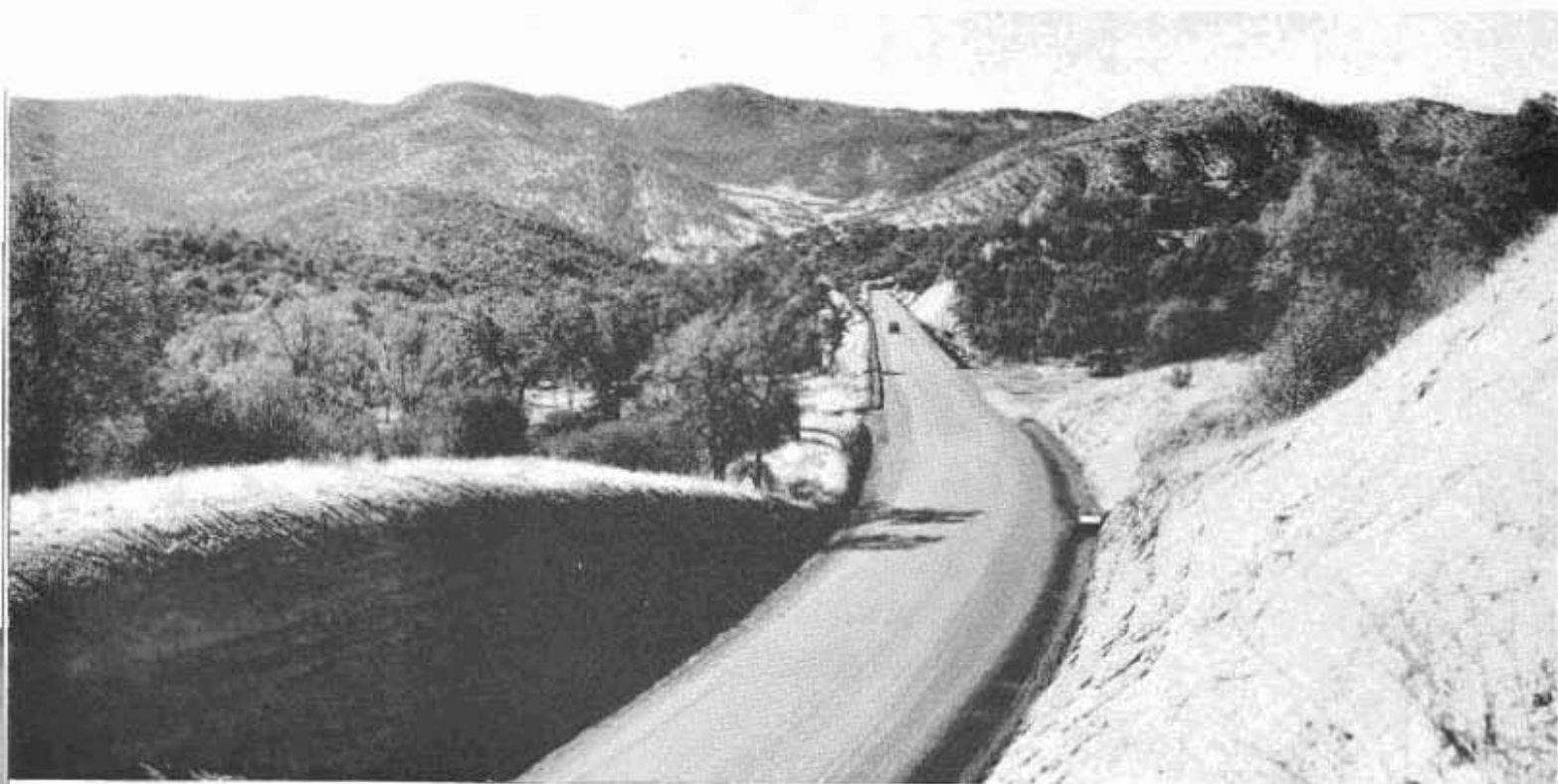
Modern type mountain road in Squaw Valley area has 26-foot bituminous surfaced roadway
