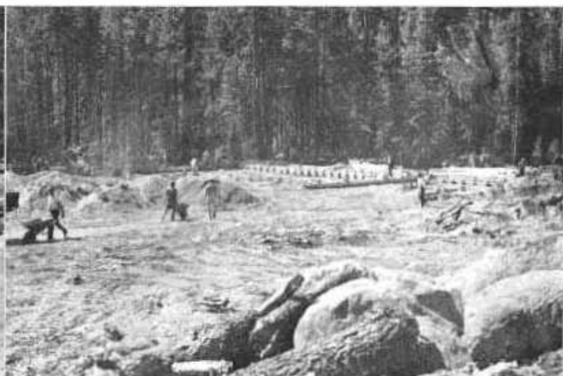
General view, with truck shed forms in background, Sept. 19
