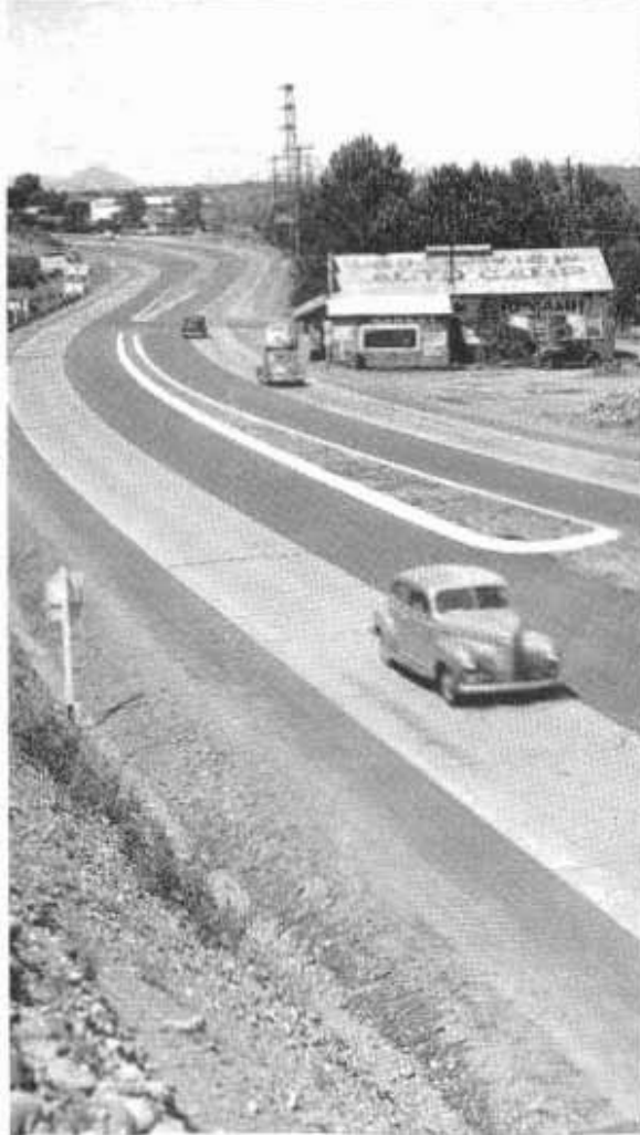
Views of channelization project recently completed on U. S. 99 near Redding that converted the existing 2-lane road into a 4-lane divided highway. At the 3-way intersection with Route 20 and the highway to Volcanic National Park, opposing traffic is separated by irregular shaped division strip areas partially bounded by concrete curbs.
