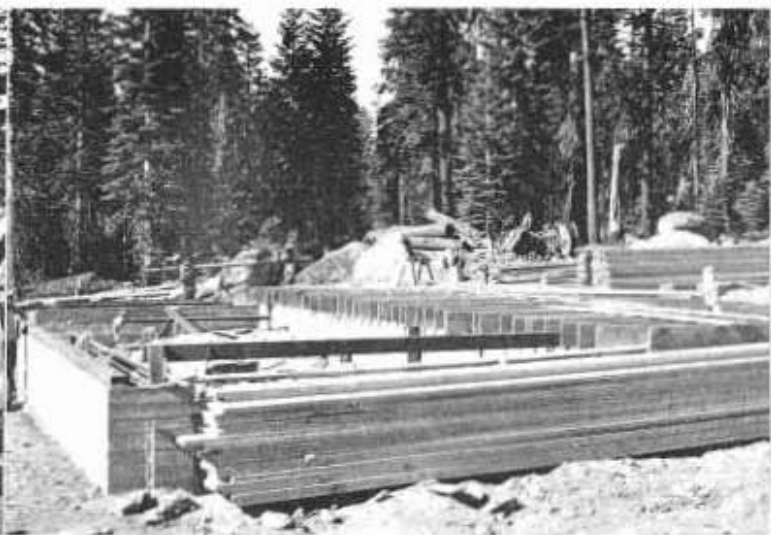
Floor joists on bunkhouse foundation, Sept. 30
