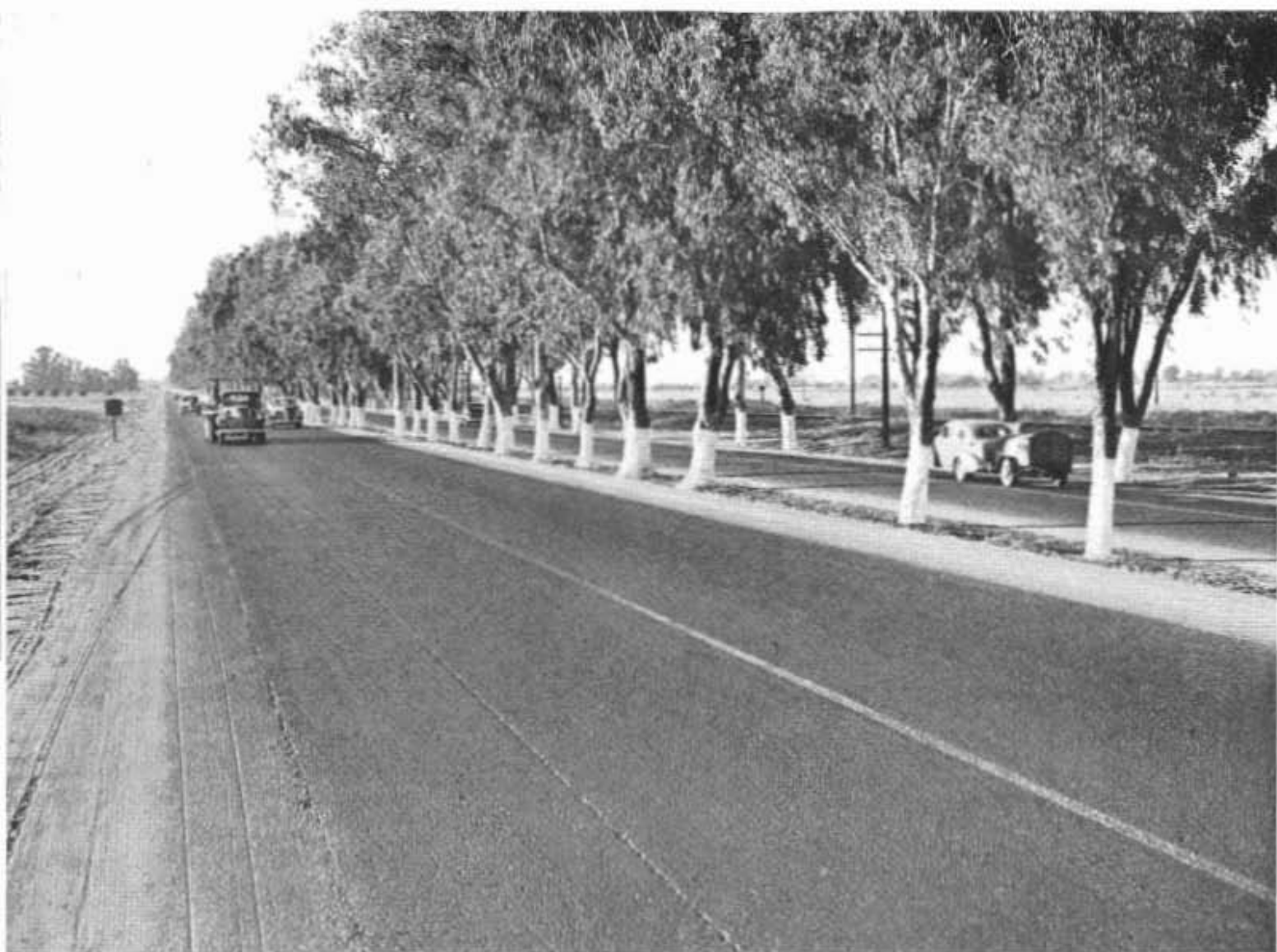
Newly completed divided highway south of Madera. Roadside trees of old road preserved as screen on division strip
