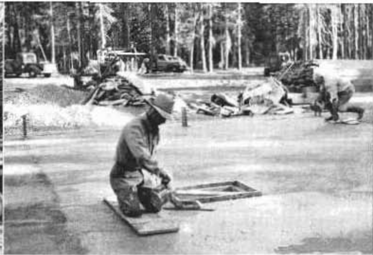
Finishing floor of truck shed on Sept. 26
