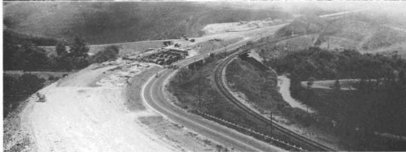
Views of reconstruction on Coast Highway west of Santa Barbara. Top and bottom scenes show Canada del Refugio bridge under construction. Here a 4-lane realignment on a fill eliminates a long dip and narrow old structure with restricted sight distance
