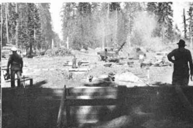
General view of work operations on Sept. 15
