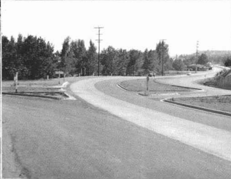
Views of channelization project recently completed on U. S. 99 near Redding that converted the existing 2-lane road into a 4-lane divided highway. At the 3-way intersection with Route 20 and the highway to Volcanic National Park, opposing traffic is separated by irregular shaped division strip areas partially bounded by concrete curbs.
