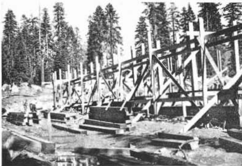
Truck shed framing being erected, Sept. 30
