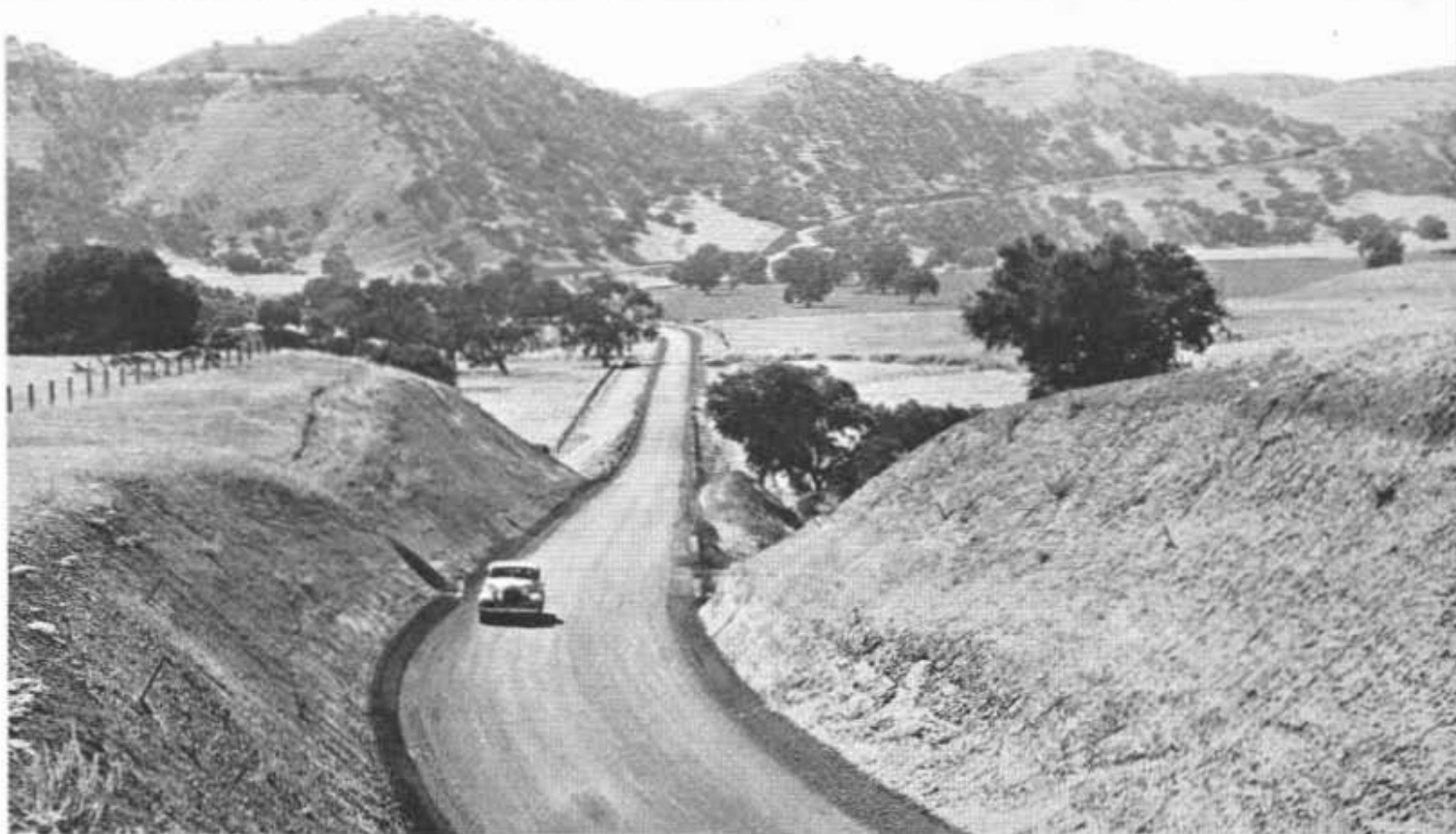
Two views of improved sections of realigned Mustang Ridge route through mountains separating San Joaquin and Salinas Valleys where a narrow old road with 123 sharp curves in 6.3 miles has been replaced by a 21 foot highway with 23 easy curves
