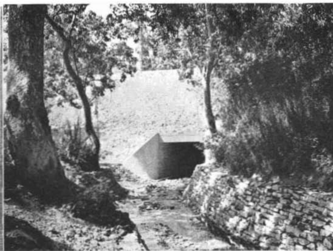
A reinforced concrete box culvert carries Tecolote Creek under highway
