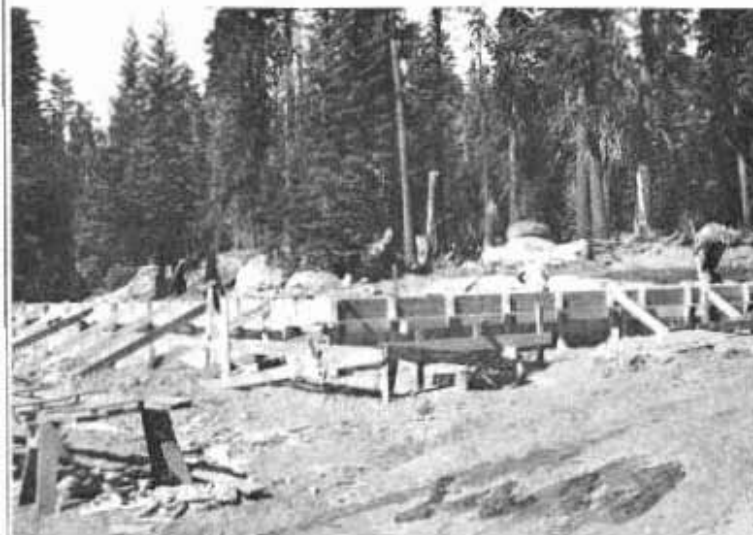
Bunkhouse foundation forms in place, Sept. 18
