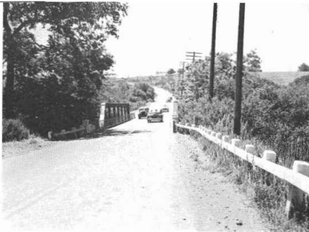
Old narrow bridge across Dos Pueblos Creek was replaced by modern structure
