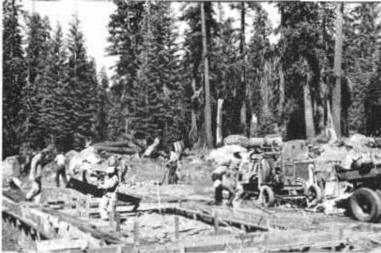
Pouring concrete on bunkhouse foundations, Sept. 23
