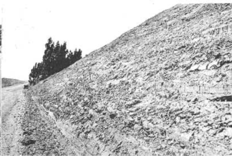
A sandy highly erodable slope left in good condition to retain top soil protective cover
