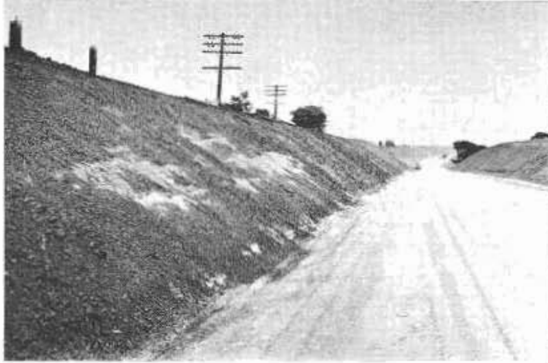
Lumps or granular particles can not be expected to stick to a 1½:1 smooth surface. Roughening is necessary
