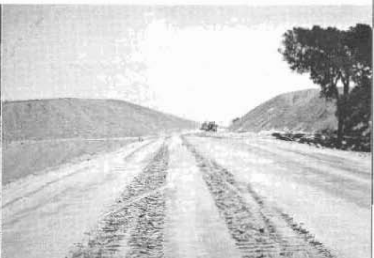
Cut slopes with transition at the ends of cuts and protected with top soil present a natural appearance
