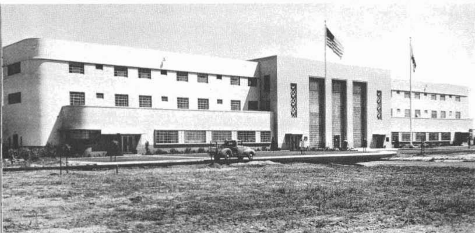
Administration Building, a 3-story reinforced concrete structure housing Warden's office, clerical staff, visitors' section and Board rooms
