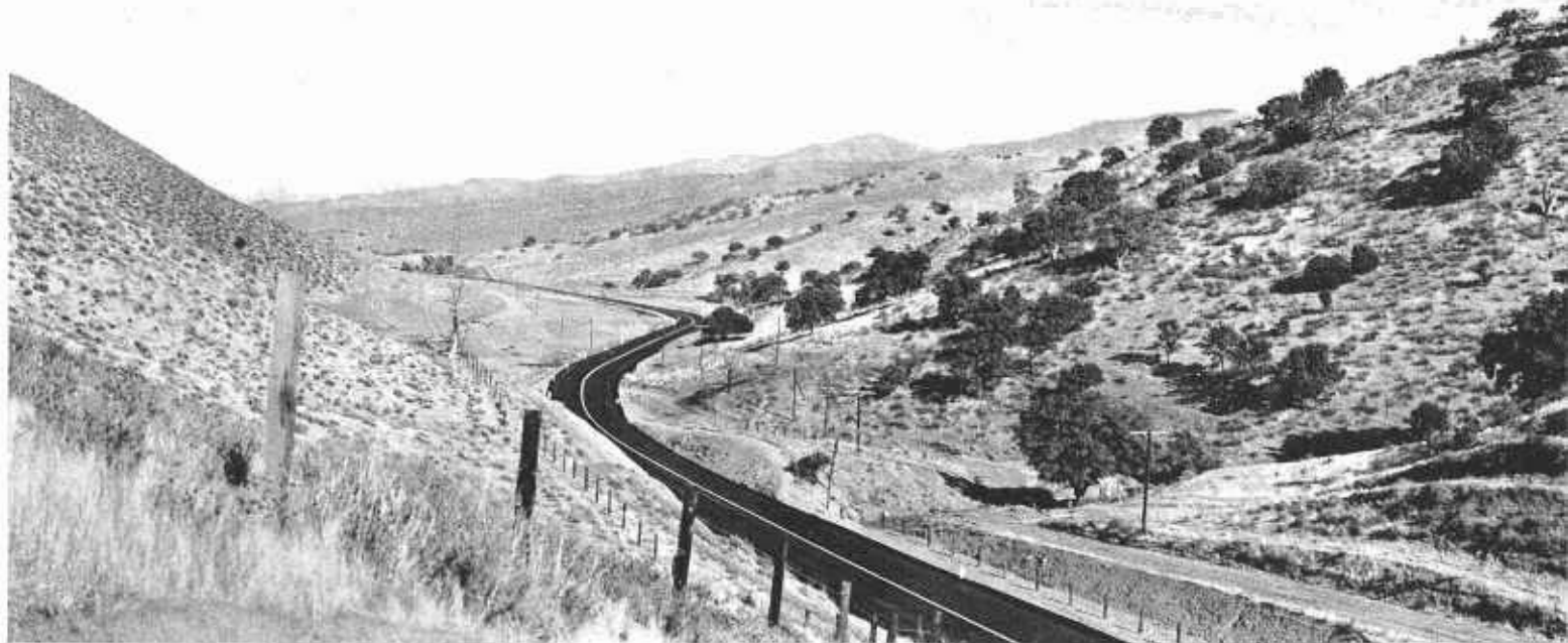
View of realigned State Sign Route 41 that connects Yosemite Park and San Joaquin Valley with the coast at Cambria
