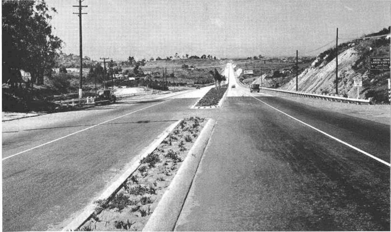
The four-lane divided highway cut-off recently completed in San Diego County between La Mesa and El Cajon includes practically all features of modern design such as grade separations, opposing traffic separations by reflectorized curbs, profile separations and channelization islands.
