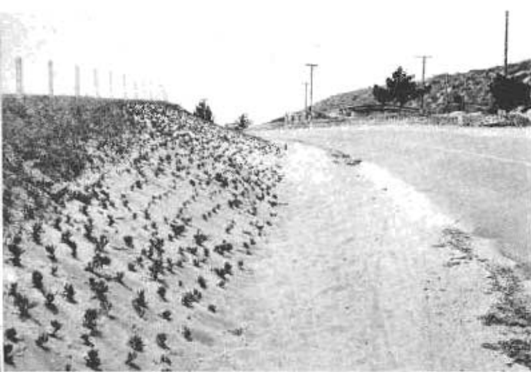
Ground cover plantings have proved unsatisfactory protection when planted on sterile slopes
