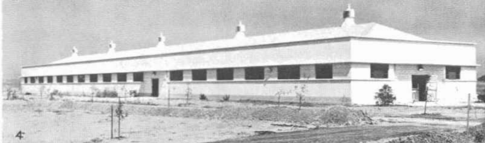
Chino institution buildings. No. 1—Observation cell block, a two-story building with 52 single rooms on first floor and 4 dormitories on second floor housing 44 beds each. 2—Mess hall, a reinforced concrete structure seating 1,200 inmates. Also contains kitchens and storerooms. 3—Westerly dormitory, a 2-story structure housing 136 men in single rooms and recreation rooms on each floor. 4—Barber shop, laundry and bath house containing shower rooms, dressing rooms and 12 barber chairs
