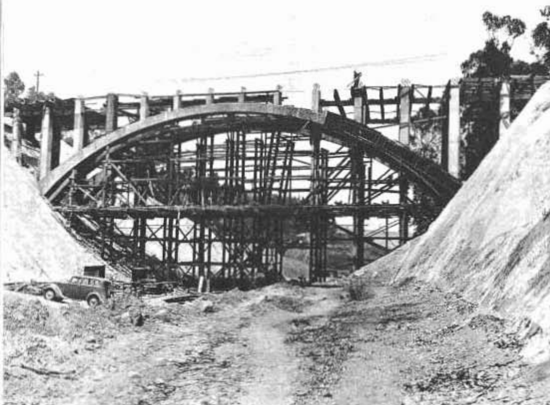
Close up view of Park Lane grade separation under construction
