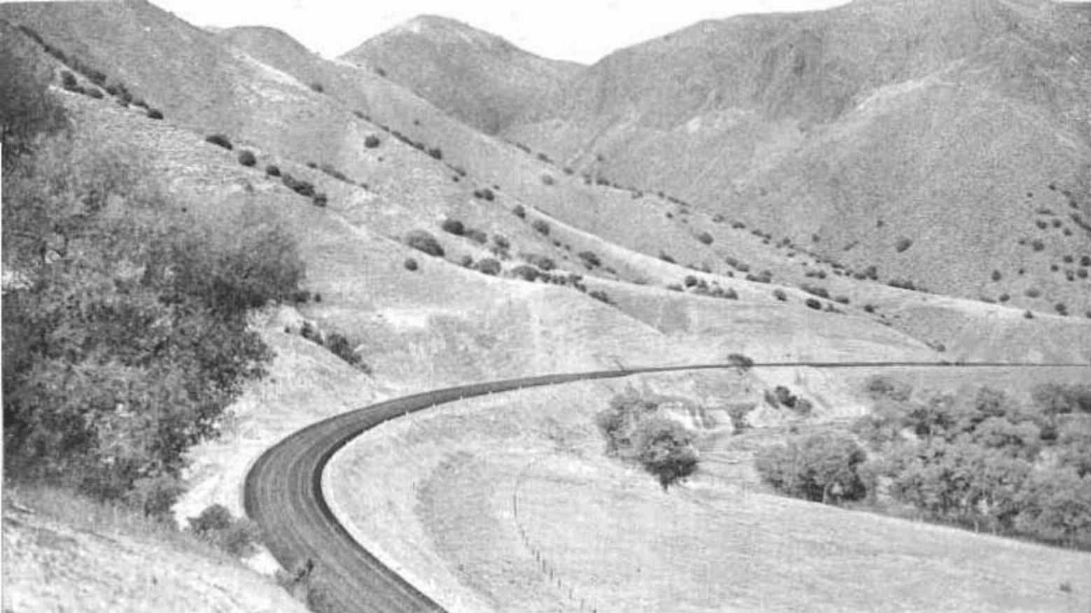
New surfaced road through Warthan Canyon swings high above creek bed avoiding a dangerous crossing of ravaging stream
