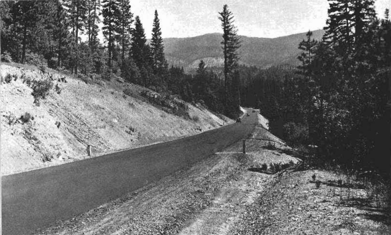
View of completed surface on the Feather River Highway in scenic region between Howells and Keddie
