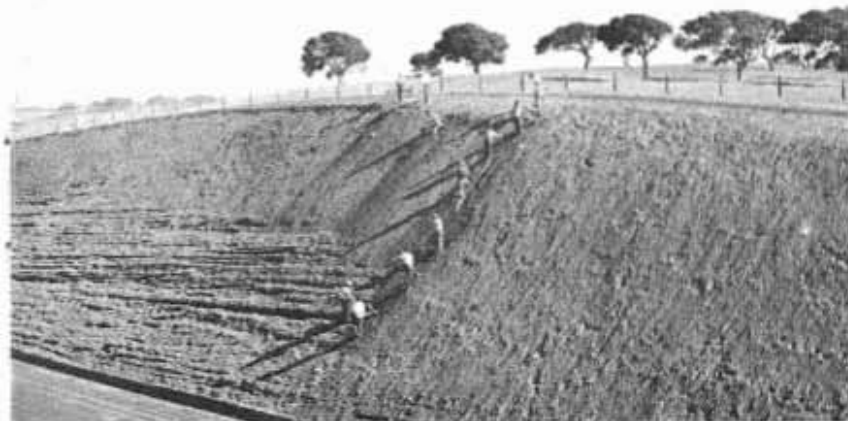
Raking top soil down—Improved appearance of cuts after covering would justify this method if no other factors were involved
