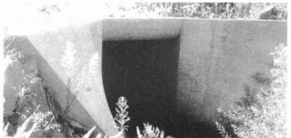
FIG. 22. Warped wing headwall with rounded-lip crown at entrance to concrete box culvert
