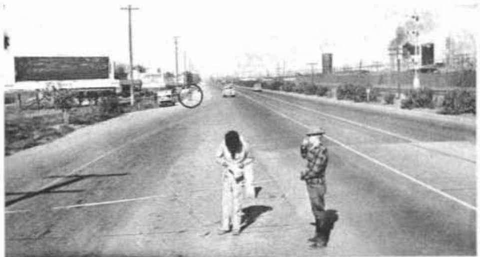
Recorder and chainman in foreground with levelman in distance
