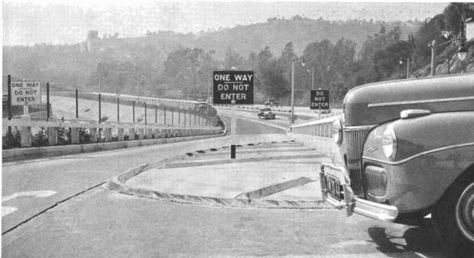
Traffic hazards created by drivers entering Arroyo Seco Parkway by way of an exit ramp will be greatly reduced by treatment pictured above
