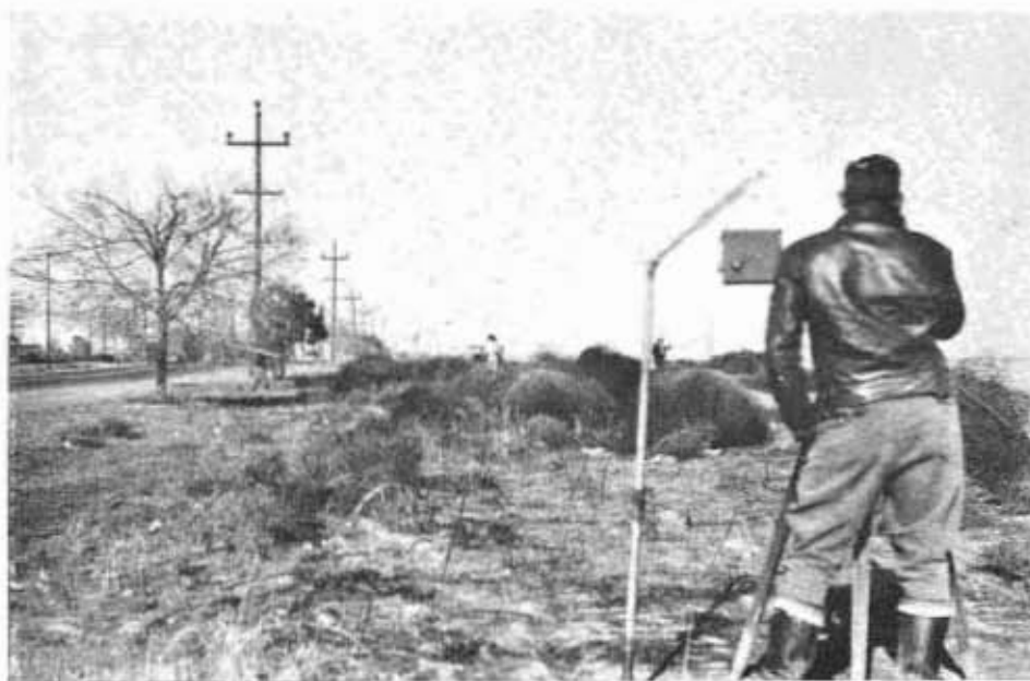
"Listening aid" suspended from flag standard to receive levelman's calls
