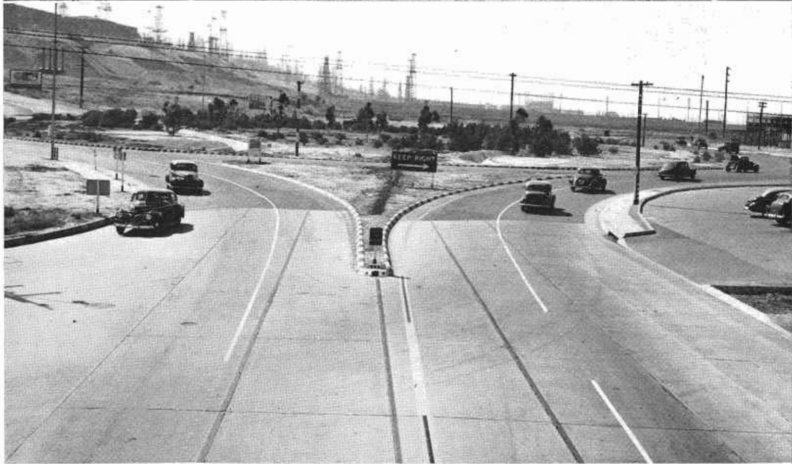
Views of reconstructed traffic circle at intersections of State Street, Lakewood Boulevard and Hathaway Avenue in Long Beach which now consists of a circle within a circle. At top—channelization at State Street entrance. Below—Hathaway Avenue approach
