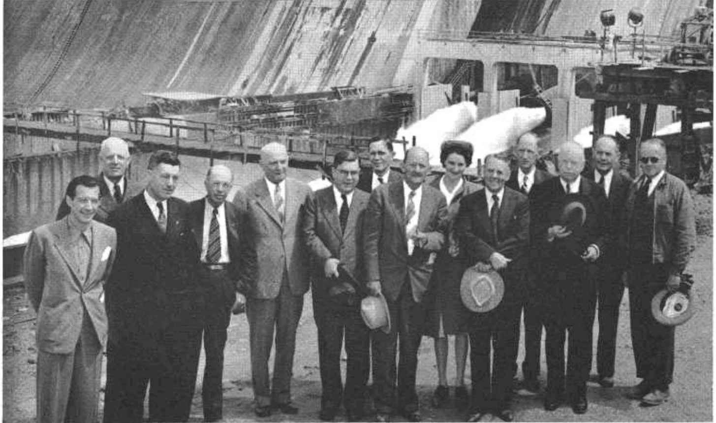
The Joint Legislative Interim Committee on Water Problems is shown here at Friant Dam, which is nearly complete. From left to right are: Executive Secretary Frank Reed; Senator Fletcher, San Diego; Assemblymen Millington, Gridley, and Watson, Orange; Senators Myhand, Merced, and Kenny, Los Angeles; State Engineer Edward Hyatt; Senator Crittenden, Stockton, Chairman; Mrs. Elizabeth Eyre, Secretary; Assemblyman Turner, Delano, Vice Chairman; Senators Cunningham, Hanford, and Deuel, Chico; R. S. Calland, District Engineer, U. S. Bureau of Reclamation and R. B. Williams, Construction Engineer.
