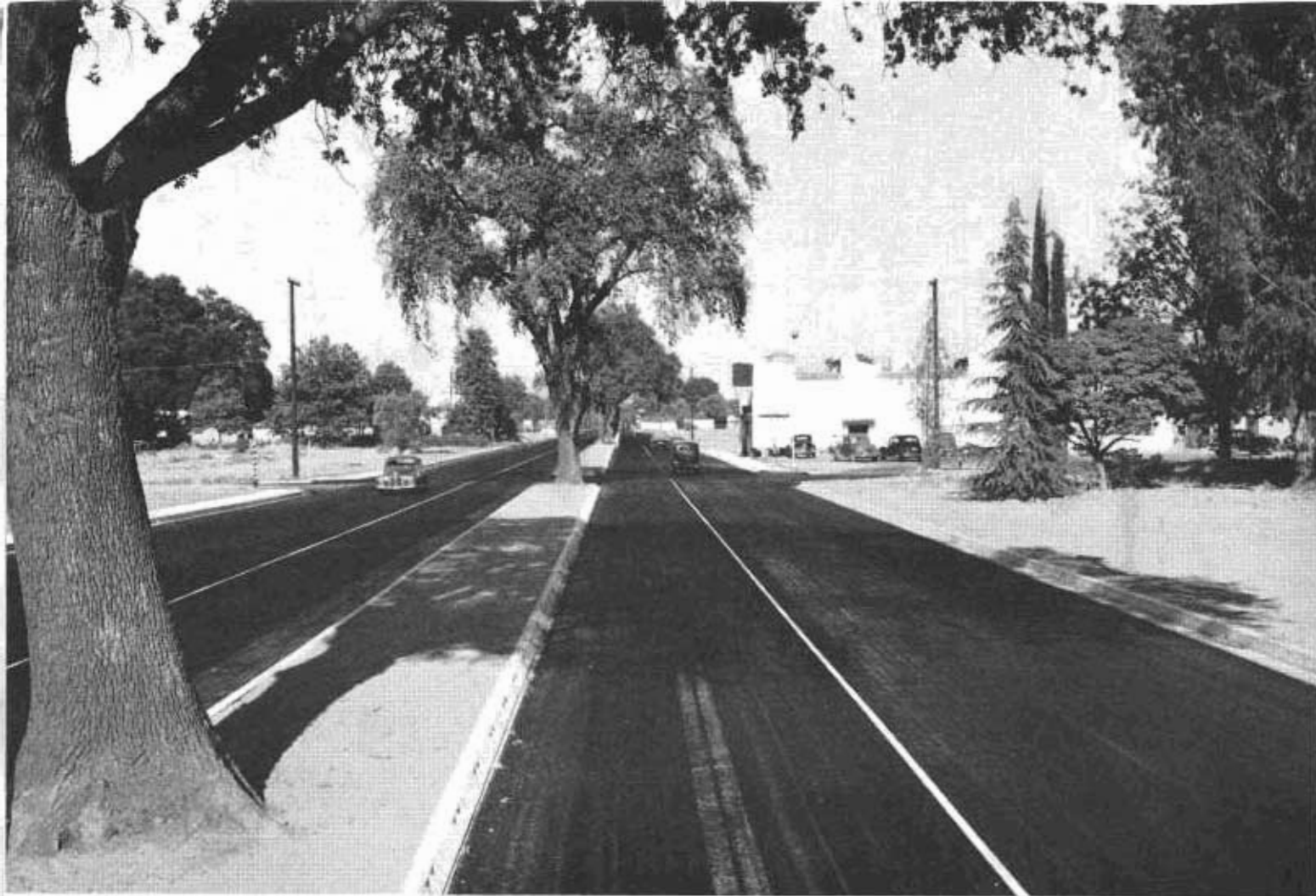
Many large, beautiful trees were saved in construction of the division strip on new 4-lane highway section through Visalia
