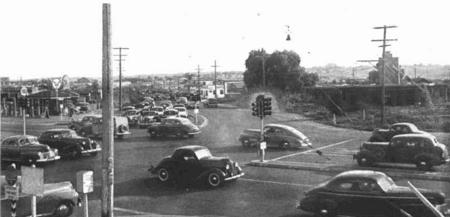
Scene at a San Diego intersection where a single automatic signal keeps four streams of traffic rolling
