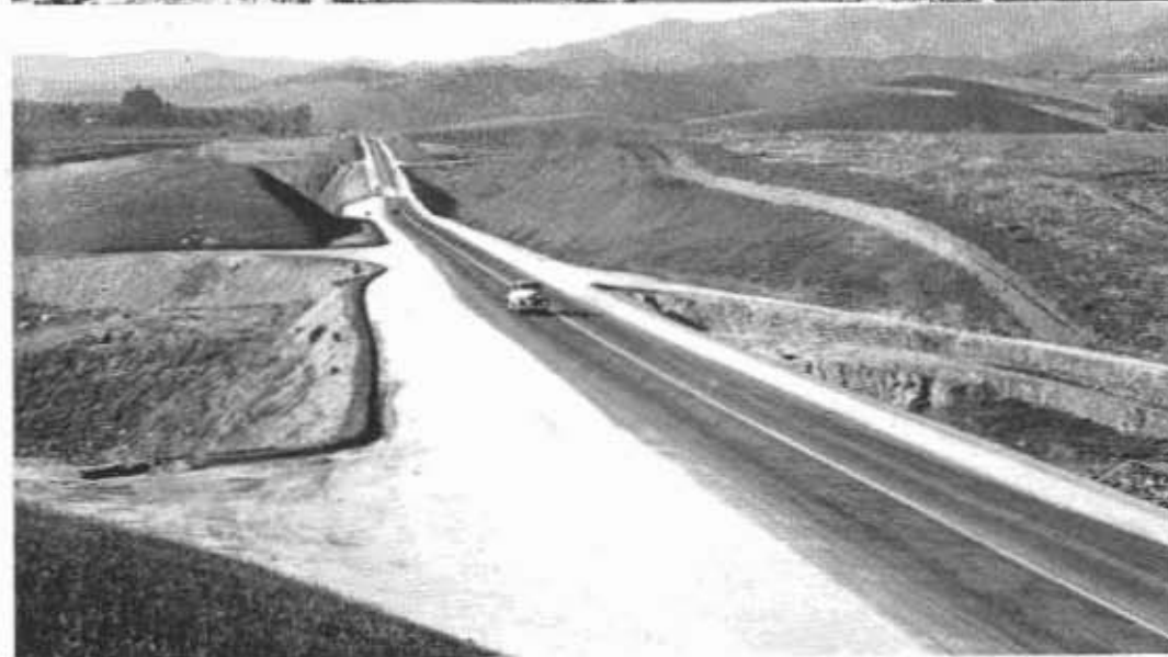
After pictures of improvements that remedied bad traffic conditions shown on adjoining page
