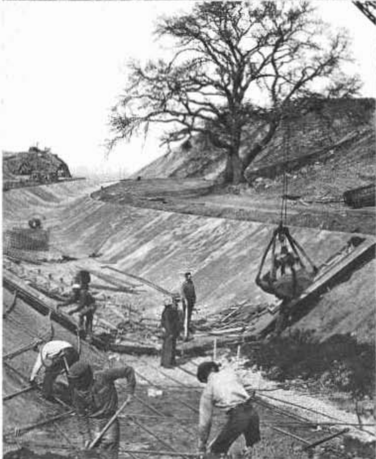
Top picture shows completed portion of flume, paralleling Grapevine Grade highway, for carrying creek waters past slide area. Lower pictures show work on reinforced concrete lining of flume and the special spillway construction at its lower end
