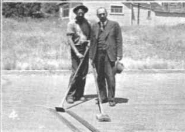
1—Durable, raised bars of asphalt concrete instead of plant-mixed bars placed in advance of safety zones adjacent to street-car tracks by use of plywood forms that rendered unnecessary the building of barricades needed to protect plant mix bars while curing. 2—Shaping iron on tracks in form. 3—Tamping iron for shape in ends of bars. 4—City Engineer Klassen of Daly City, who devised method, and equipment operator Cafferreta
