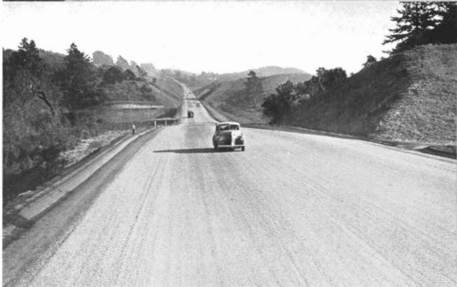
Two views of three-lane highway between Watsonville and Rob Roy Junction which replaces old two-lane road and relieves traffic congestion in Pajaro Valley. Highway ultimately will extend to Santa Cruz.
