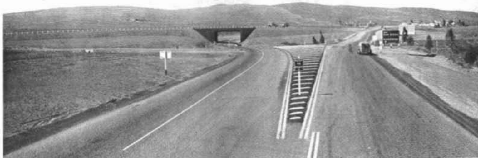
Top—View west. Pepper trees previously bordered old two-lane road. One row now in dividing strip. Center—Dual roadway sections each paved 23 feet in width. Dividing strip is 30 feet wide between near edges of pavement. Bottom—View west. Island between traffic channels constructed of bars made of plant-mixed surfacing and painted white. Grade separation structure in center.
