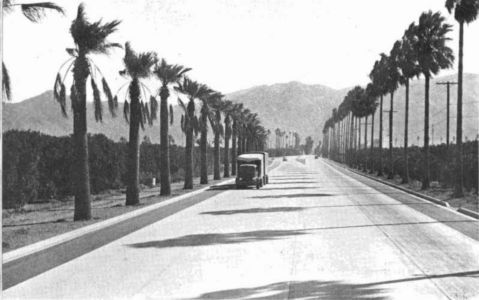
Palm trees on right were moved and reset outside of curb line. Palms on left were left in place.
