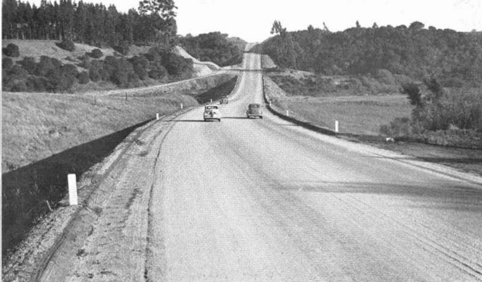
This stretch of new Watsonville-Rob Roy highway shows easy grade alignment and sight distance advantages.
