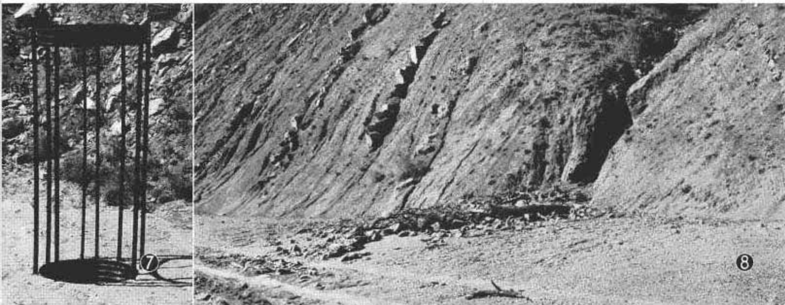
FIGURE 7. Metal debris riser placed over culvert entrance in debris basin. Note provision for extension when debris basin has filled to such an extent as to cause deposition of most of the detritus before it reaches the riser
