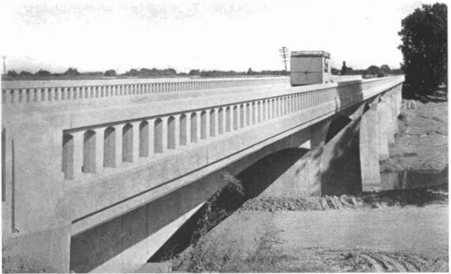
One of two one-way bridges on Davis-Dixon cut-off. Each one carries two lanes of traffic across Putah Creek.
