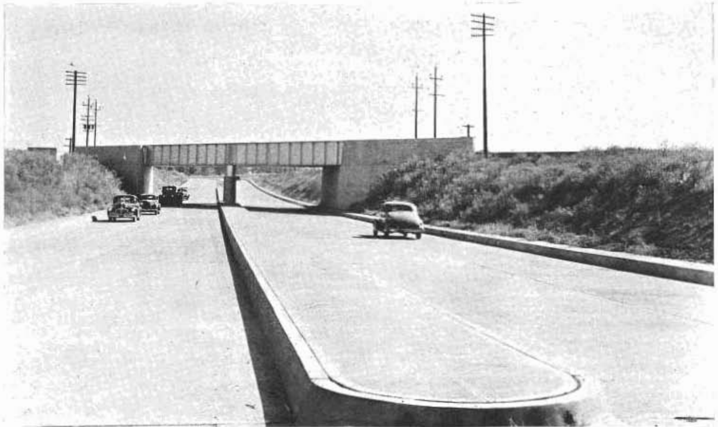
Four-lane divided underpass on Davis-Dixon cut-off where the Southern Pacific Railroad crosses the highway. This structure is one of the modern features which permit a saving of 150,000 vehicle hours annually
