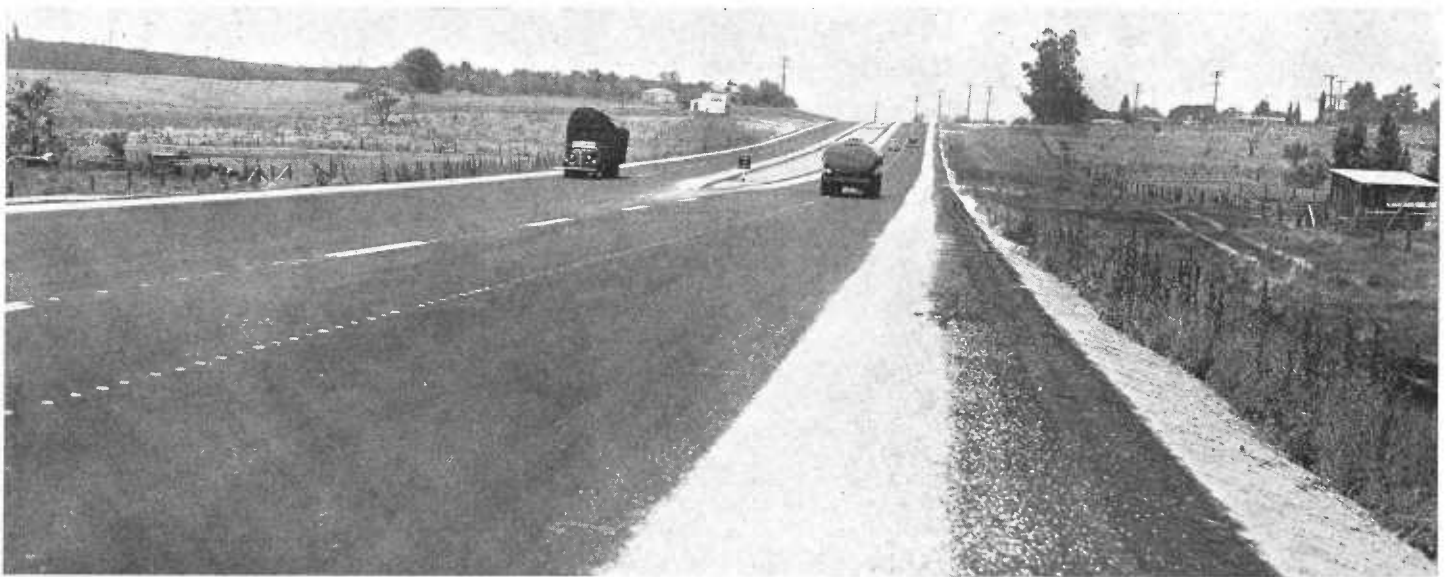
View showing transition section where divided highway merges into two-lane existing highway ahead at end of project
