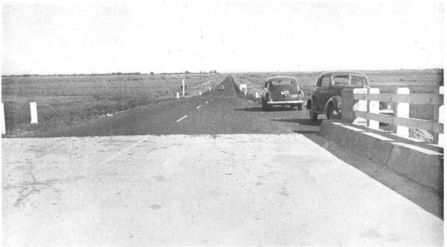
New Lodi-Rio Vista cut-off highway looking East from the timber trestle approach to Mokelumne River Bridge
