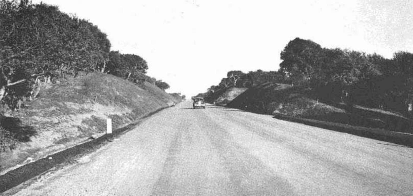
View of unfinished realigned section of Prunedale-Castroville road showing straight tangent eliminating many curves and grades
