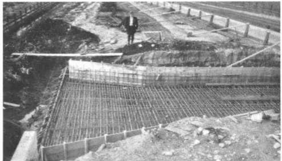
Fig. 43. Vallejo Creek. Construction of flare-siphon culvert
