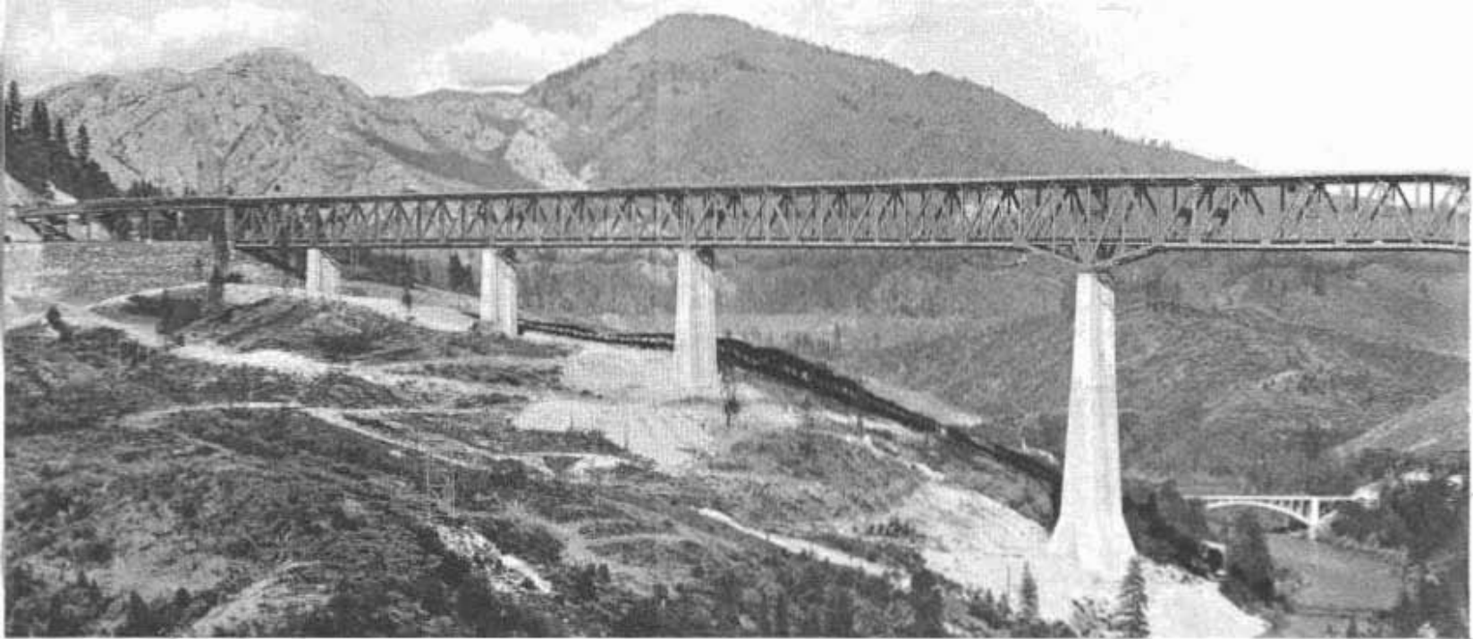
Photograph of Pit River Bridge, a double-decked structure carrying a railroad on the lower deck and the highway on top 350 feet. The existing
