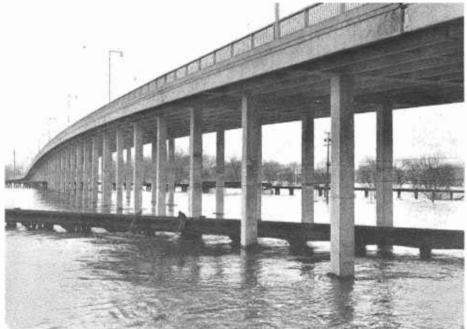
Tracks of Sacramento Northern and Western Pacific railroads just escape submergence
