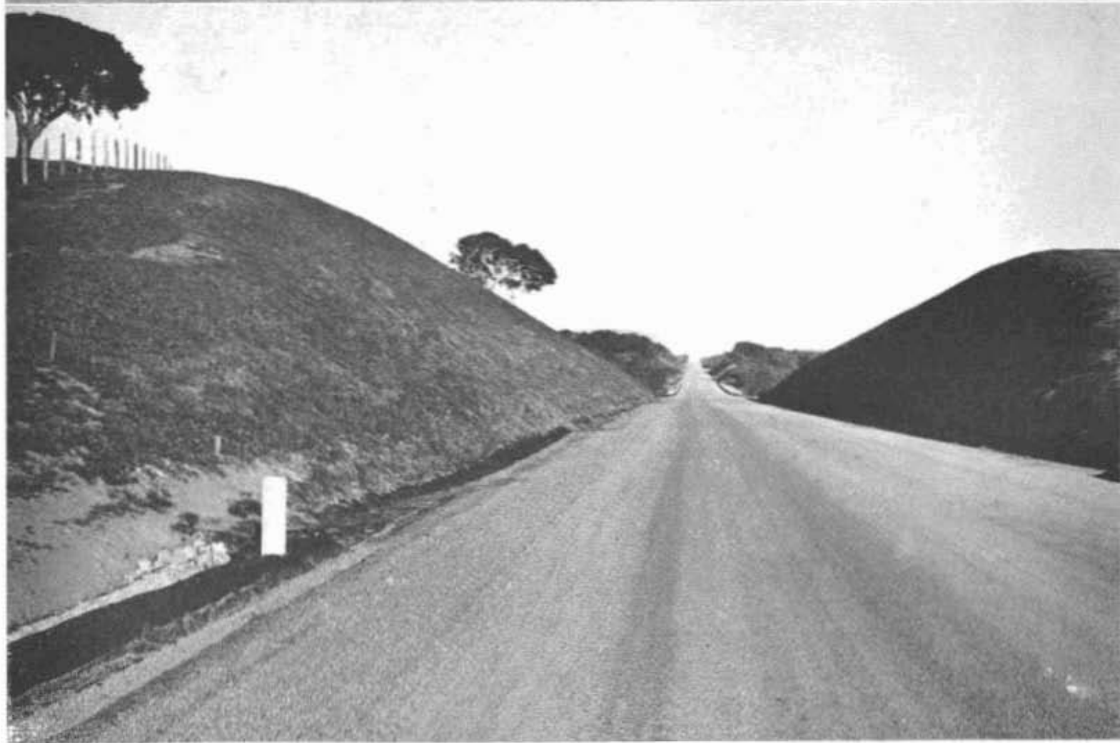
Two views of realigned and regraded sections of cut-off between U. S. 101 and coast taken before road was opened. Alignment is of high standard containing but 4 curves which have a minimum radius of 2500 feet. The 36 foot roadbed has a 22 foot plant mixed surfacing on a crusher run base and 7 foot shoulders, bituminous surface treated.
