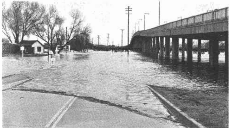
Viaduct 50 feet above ground level, crosses channel and two railroads
