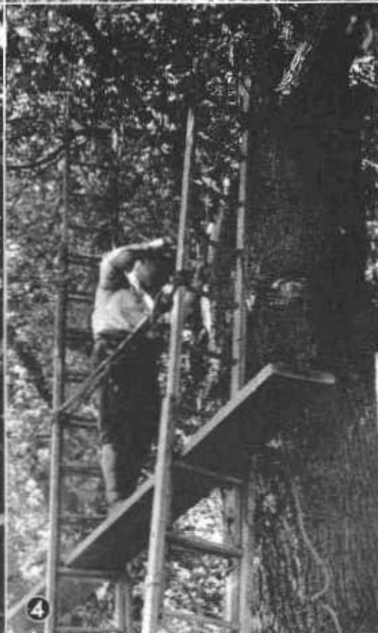
Tree doctors and their work. 1 and 2—Before and after views of elm tree trunk showing decayed heart wood in an old cut, and completed cavity, lip bolts and drain tube in place, ready for sectional concrete filling. 3—Tree Foreman A. E. Burnell, operating an electrically powered chisel for removal of decayed and infected heart wood. 4—Tree Trimmer Leo Simoni shaping a cavity with hand chisel and mallet.
