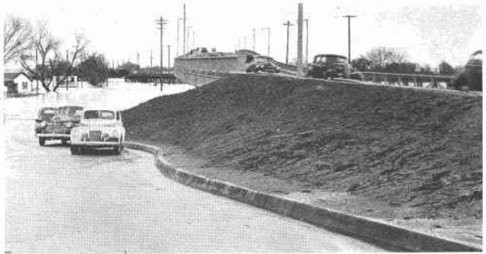
Old section of U. S. 40 across American River overflow was flooded but 16th Street Viaduct opened Sept. 14, 1942, carried all traffic
