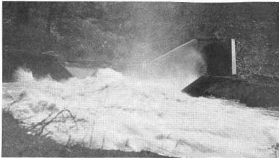
FIG. 35a. Bucket outlet deflects Salt Creek through angle of 70°
