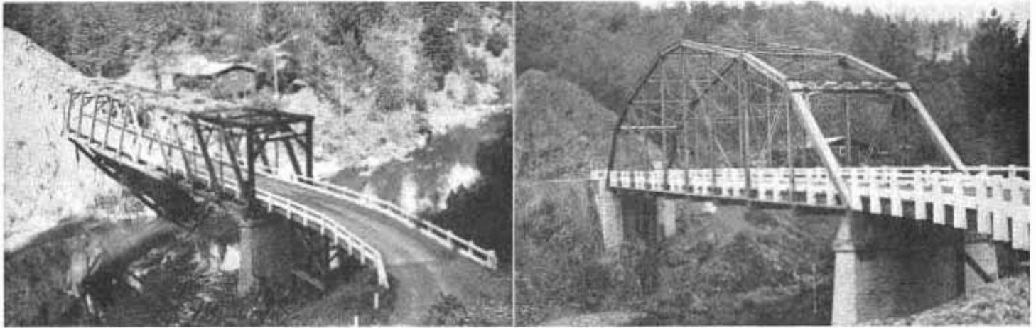
At left, old Salmon River Bridge at Somesbar, Siskiyou County. At right, how it looks rebuilt with steel salvaged from Eel River bridge at Scotia.
