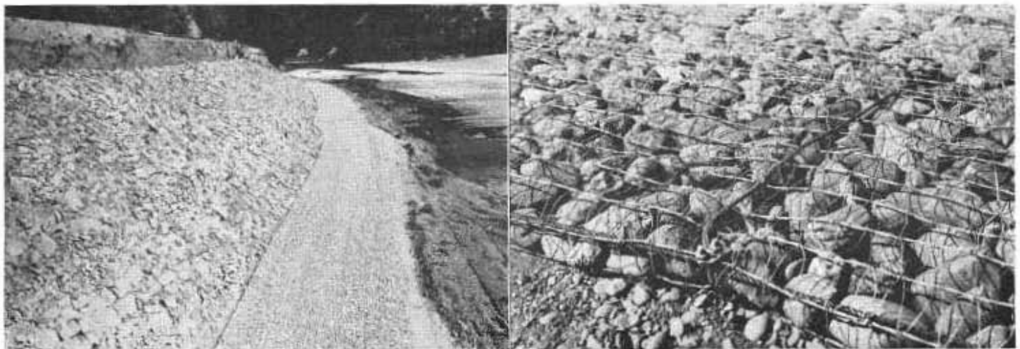
Rock riprap and wire mattress protection of left bank of Eel River below Dyerville. Left: general view, looking downstream. Right: detail of mattress and cable tie.
