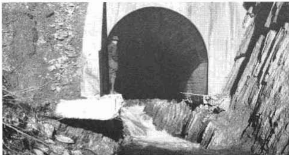
FIG. 31b. Soft bed rock has been scoured rapidly by accelerated boulder-laden flow
