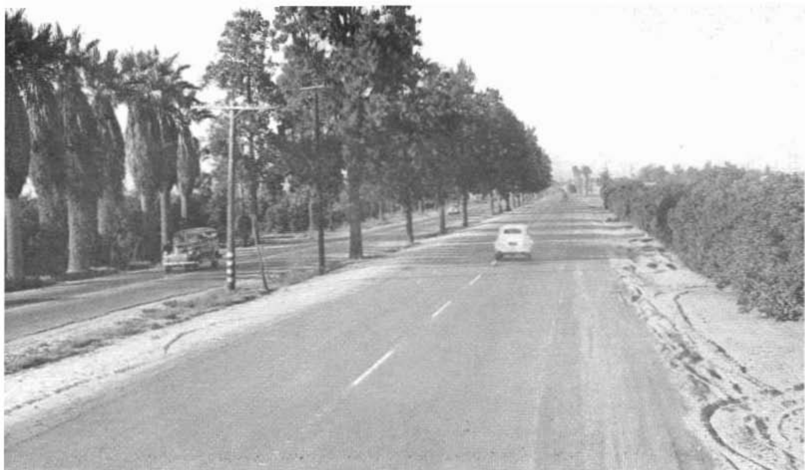
Section of 4-lane divided highway through Buena Park on State Highway 171 in Orange County.
