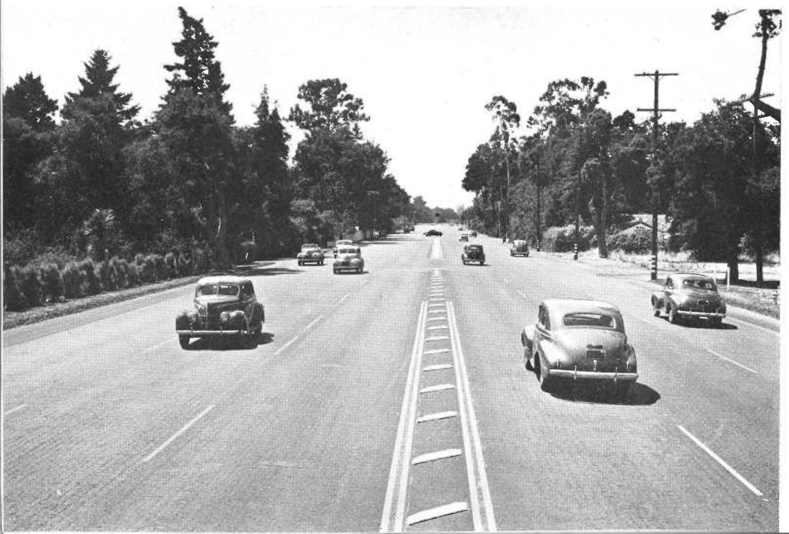
Typical view of widened section of U. S. 101 near Atherton providing a 6-lane divided highway
