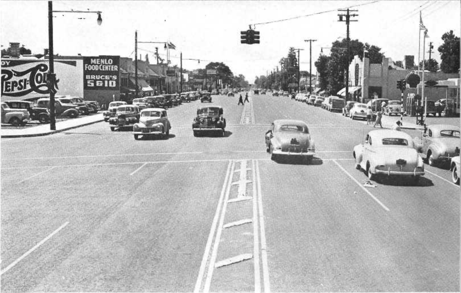
Top, improved section of U. S. 101 showing channelized division strip approaching Atherton. Below, widened avenue through Menlo Park
