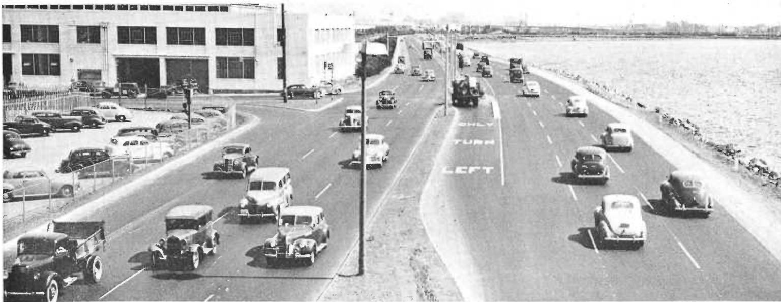
Indentation of the median strip provides a waiting or storage lane for vehicles turning left and avoids holding up through traffic
