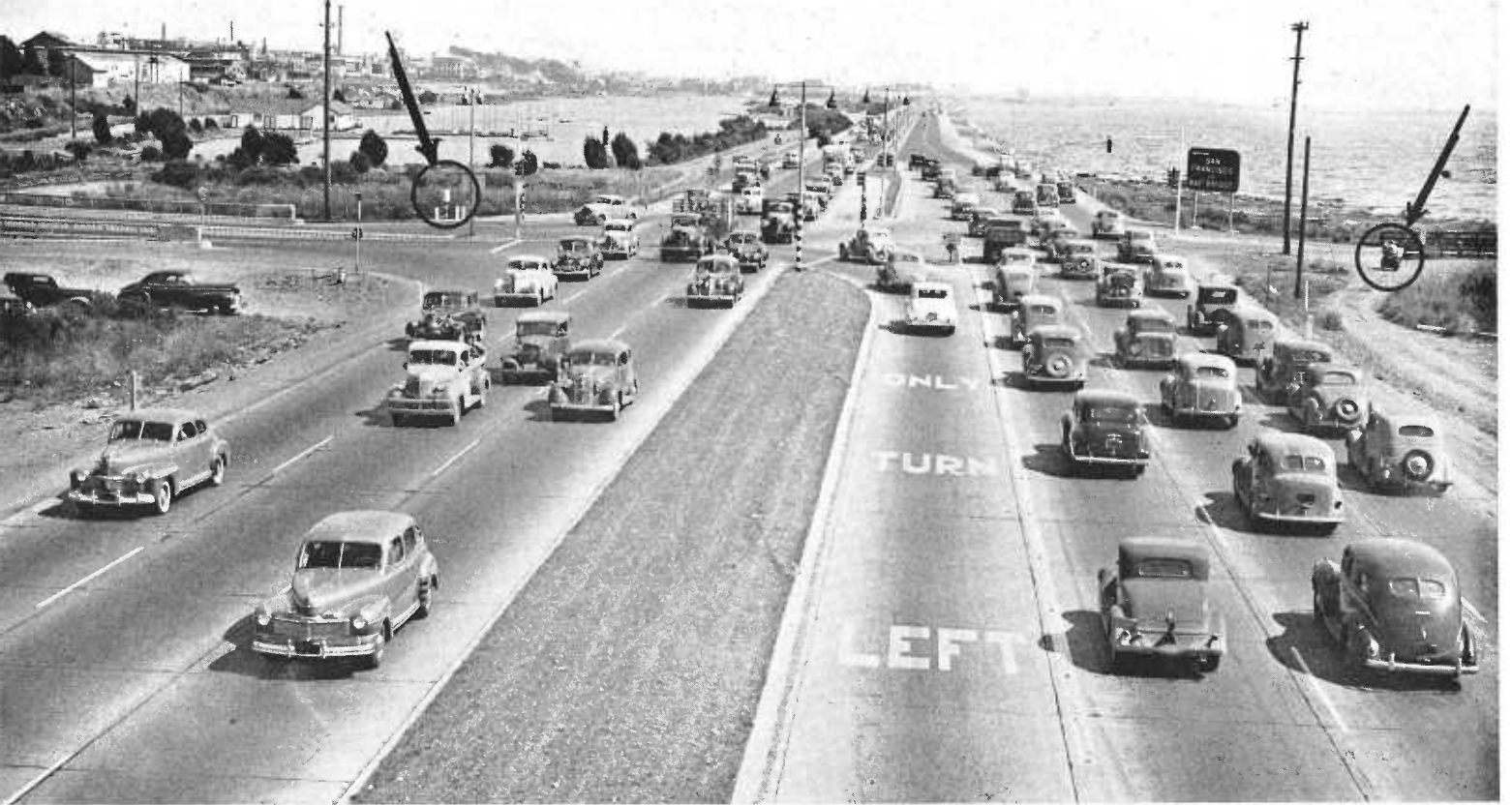
Scene at intersection on East Shore Highway, Contra Costa County, where an electric monitor (in circle at left) governs through and turning movements on six lanes of heavy traffic watched by officer on bike shown in circle at right
