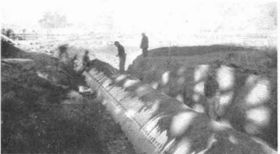
Below—Fig. 50. Crusher run backfill placed and jetted by contractor in lieu of compaction backfill
