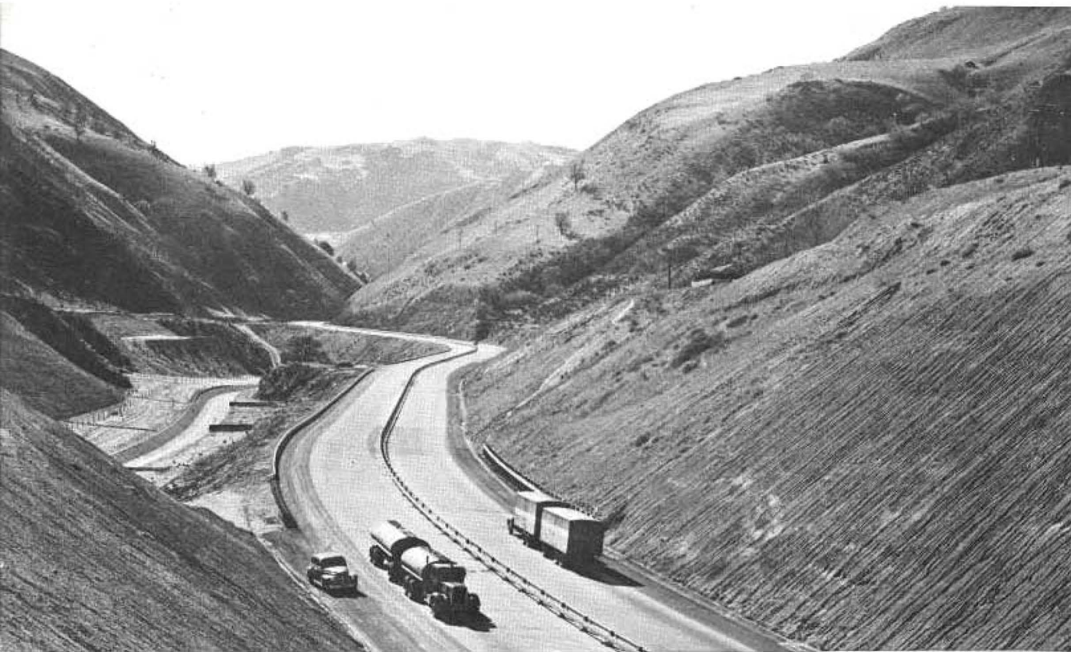
Section of new 4-lane divided highway in Grapevine Canyon, showing metal plate road divider and concrete flume for creek at left.
