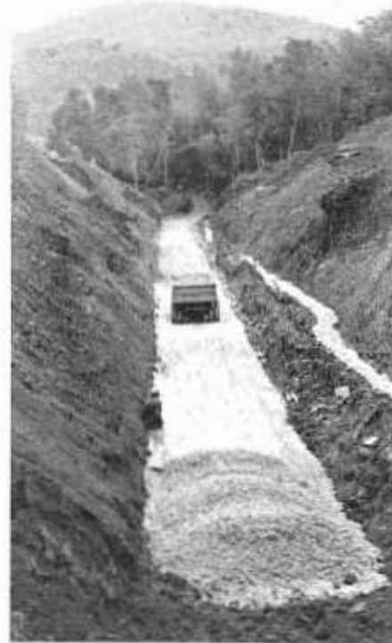
Fig. 47 (i, j). Right and wrong way of installing culverts in sidehill location
