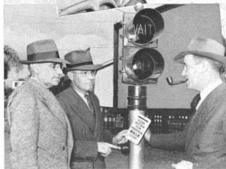
Scenes at automatic traffic signal in San Diego. Top left—Electric brain that receives messages from magnetic traffic detectors and operates signals. Top right—Pedestrians on safety island awaiting effect of push button signal. Center—Market and Pacific intersection. Bottom left—Pedestrian "Wait-Walk" signal. Bottom right—Left turn signal and magnetic detector coil buried in pavement
