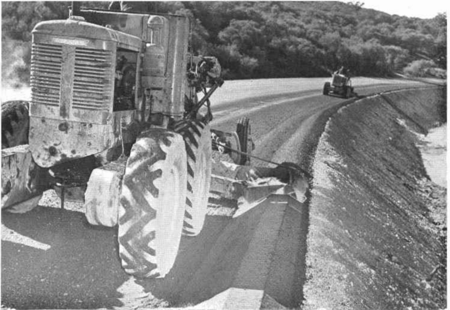
Picture of dozer spreader with spreader-box blade attachment constructing plant-mixed berm and gutter
