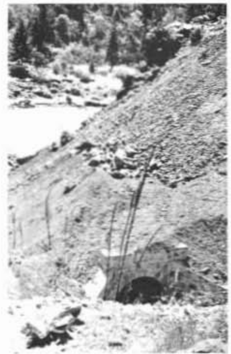
Fig. 52. Left—Masonry arch culvert under construction. Right—Same culvert unequally loaded by end-dumped material on one side (material to be rehandled to a lower level for compaction).
