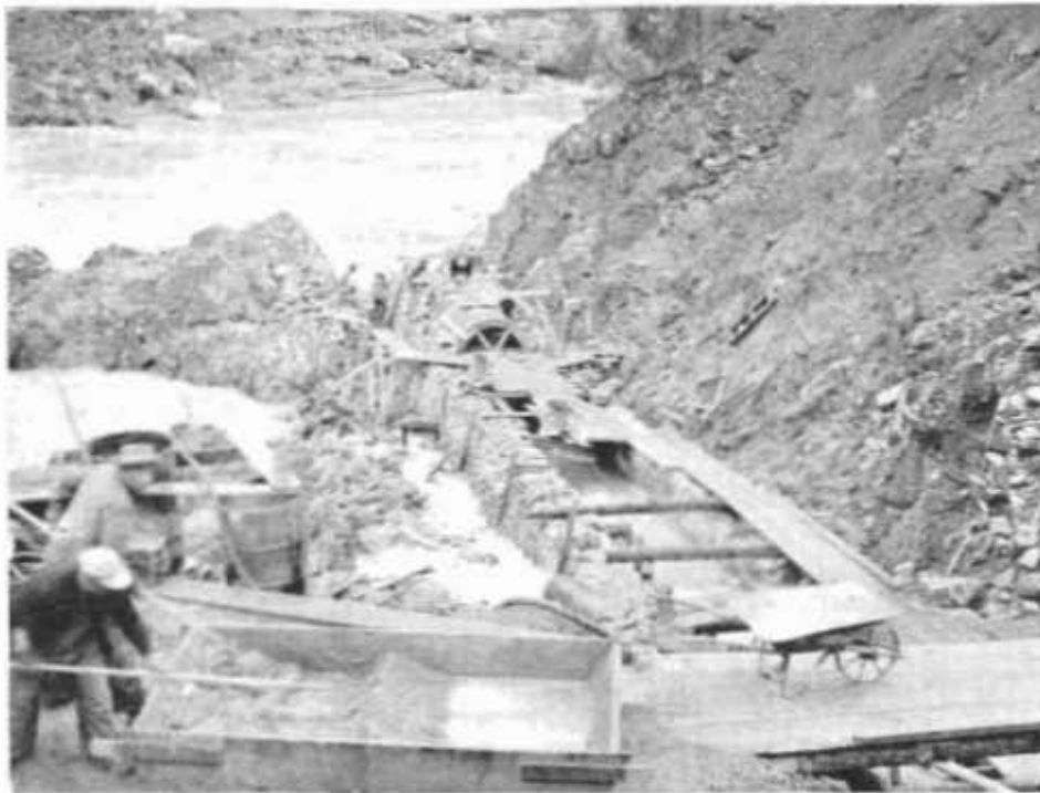
Fig. 52. Left—Masonry arch culvert under construction. Right—Same culvert unequally loaded by end-dumped material on one side (material to be rehandled to a lower level for compaction).
