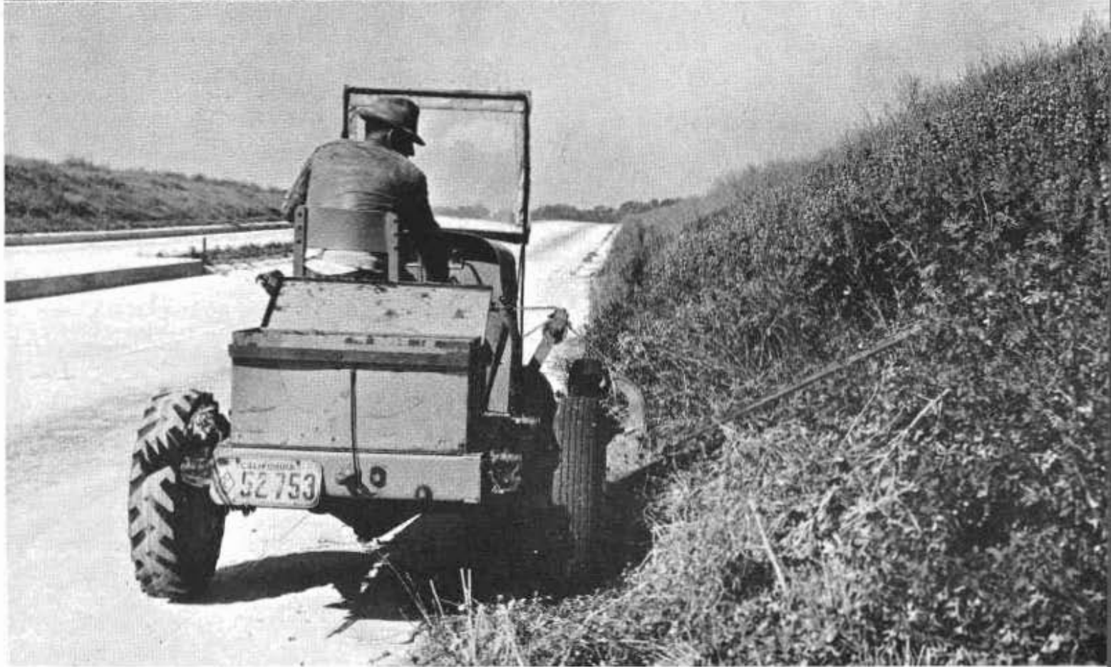
At top—Spraying roadside slope with diesel oil preparatory to burning. Simplified adjustable boom equipment is operated by one man from front of tank truck. Bottom—Mowing tall dry growth reducing fire hazard
