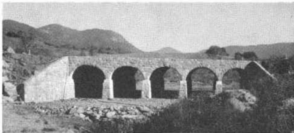
FIG. 57. Quintuple culvert of rubble masonry and metal arches, Moosa Canyon on State Highway in San Diego County
