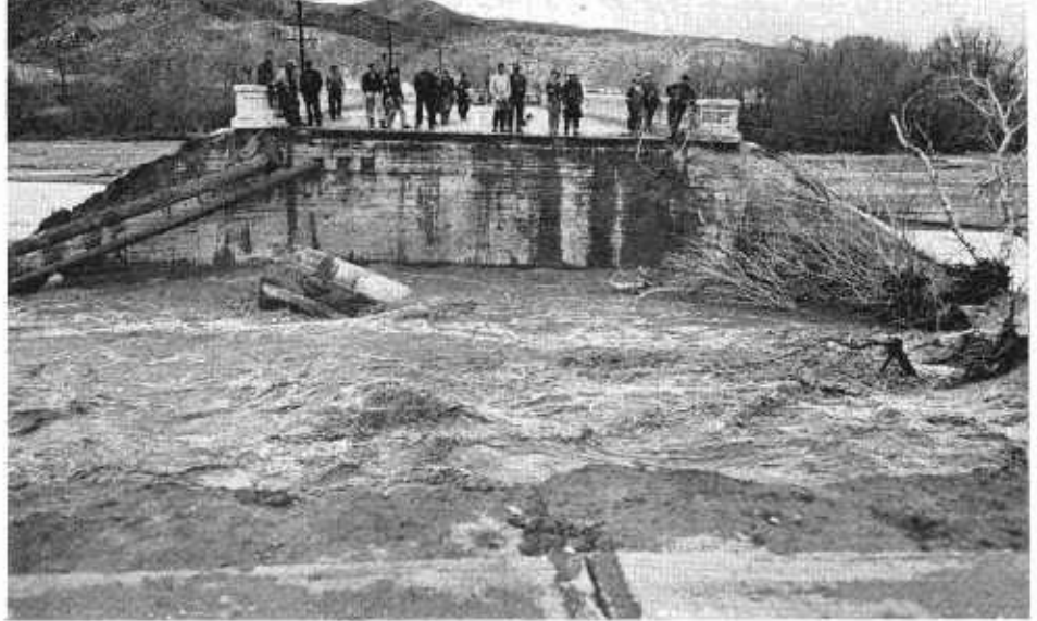
Approach to Castaic Creek Bridge on U. S. 99 in Los Angeles County washed away
