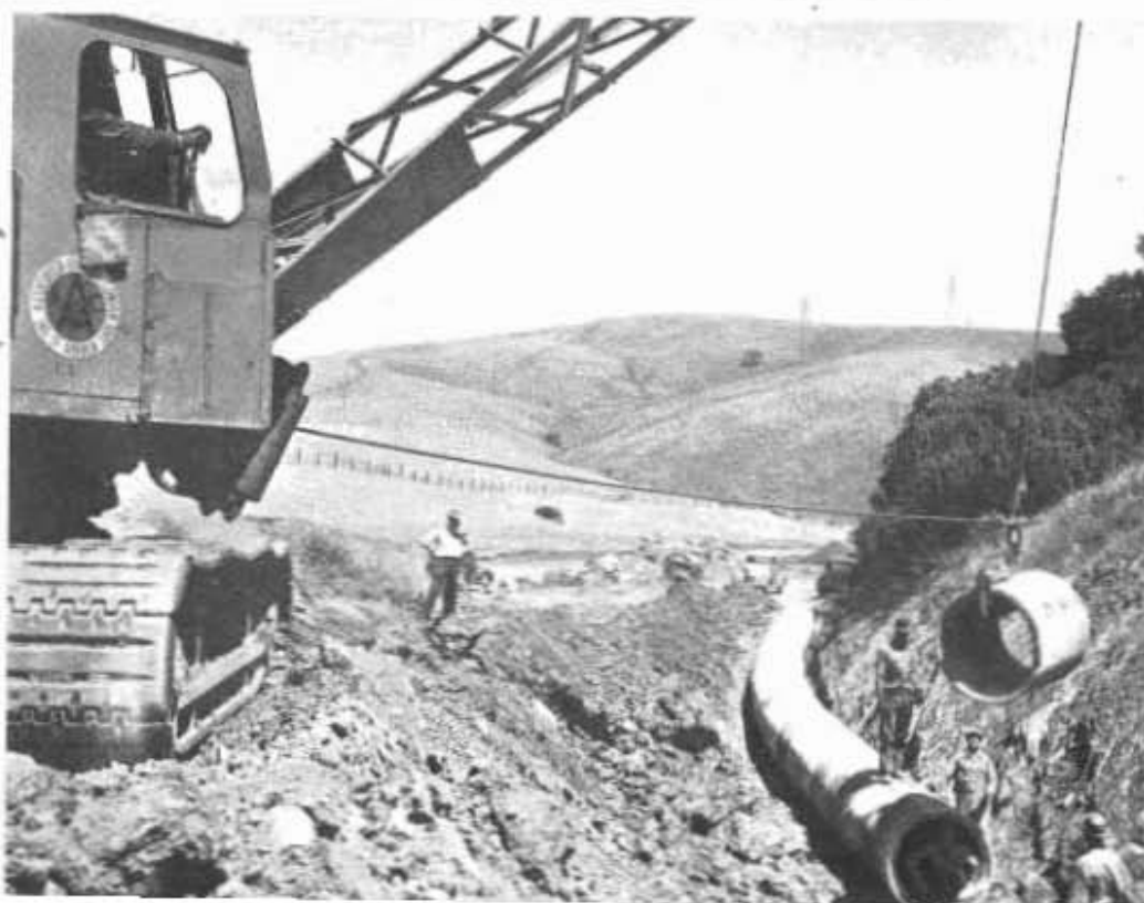
Dragline placing 36-inch reinforced concrete drainage pipe
