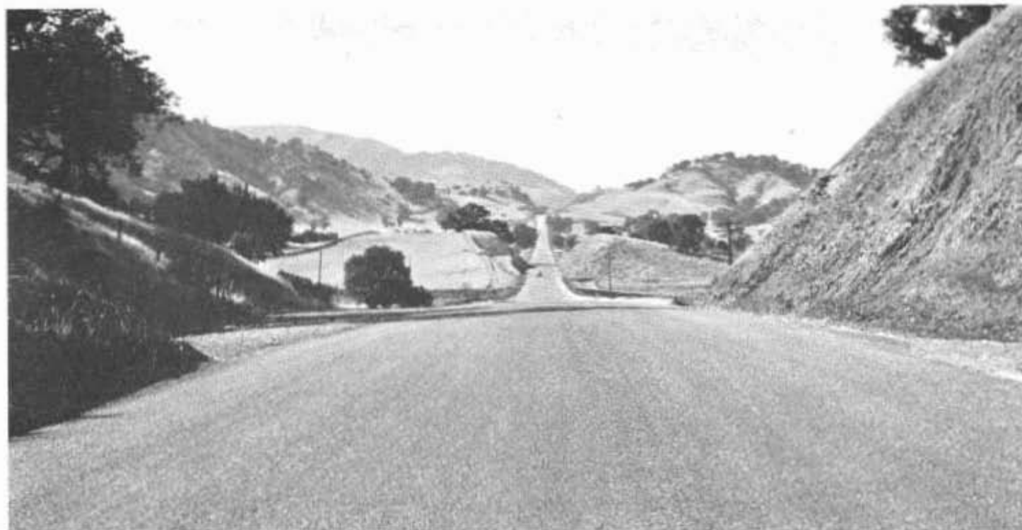
Redwood Highway improvement north of Hopland involved several long deep cuts on new direct routing
