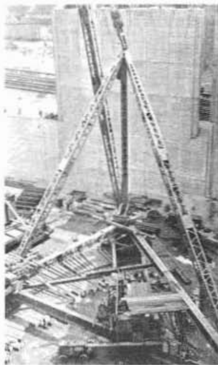
Stiff leg derrick did the work
