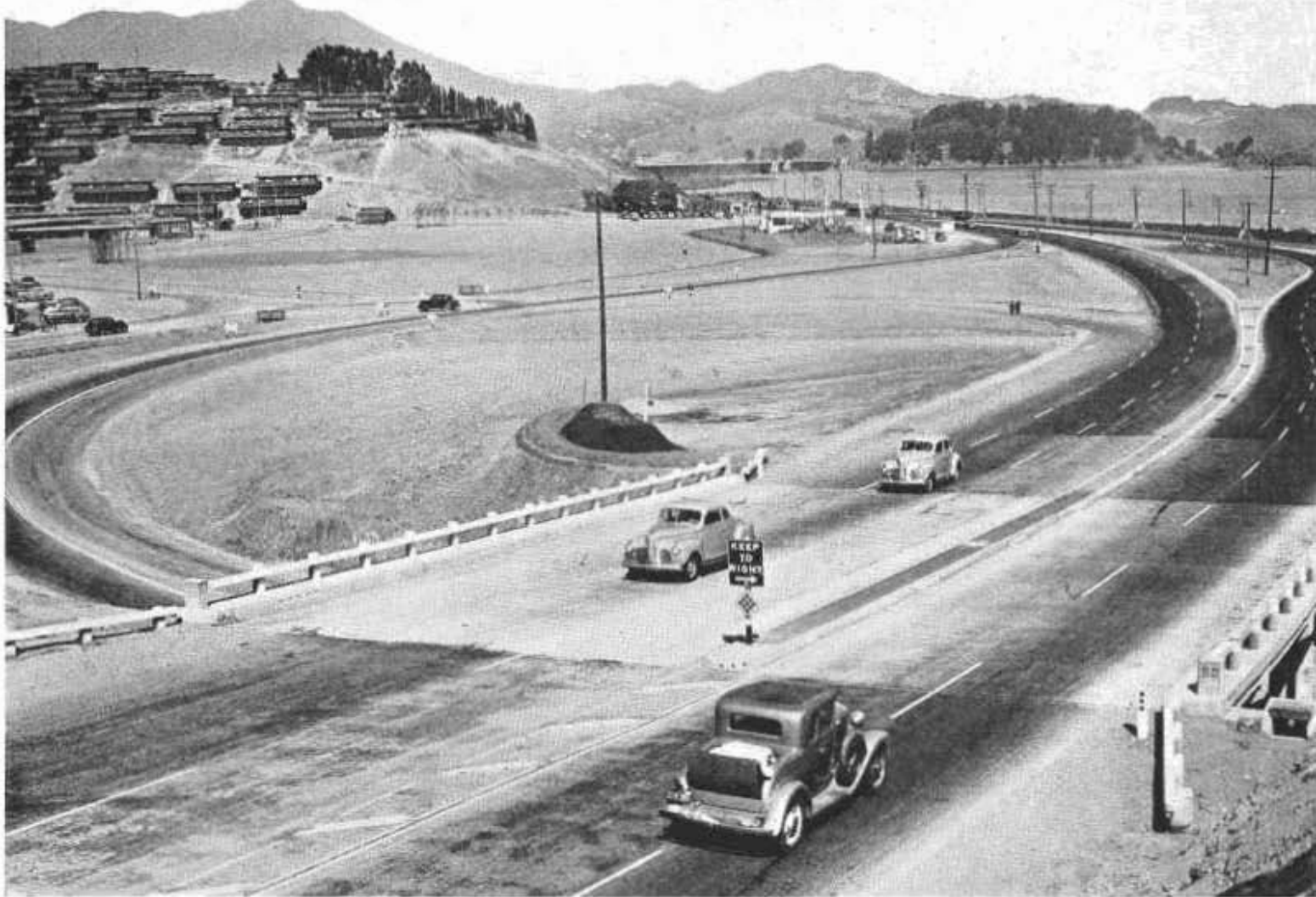
View of Waldo grade separation of U. S. 101 and Marin City road. Bridge structure carries 5-lane divided highway
