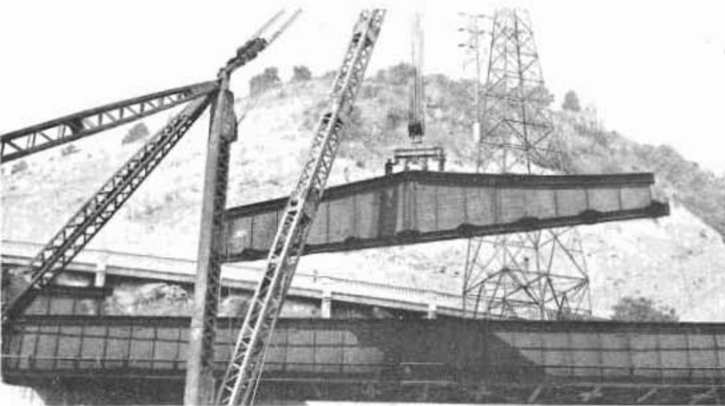
This 70 ton member had to be swung 100 feet in the air
