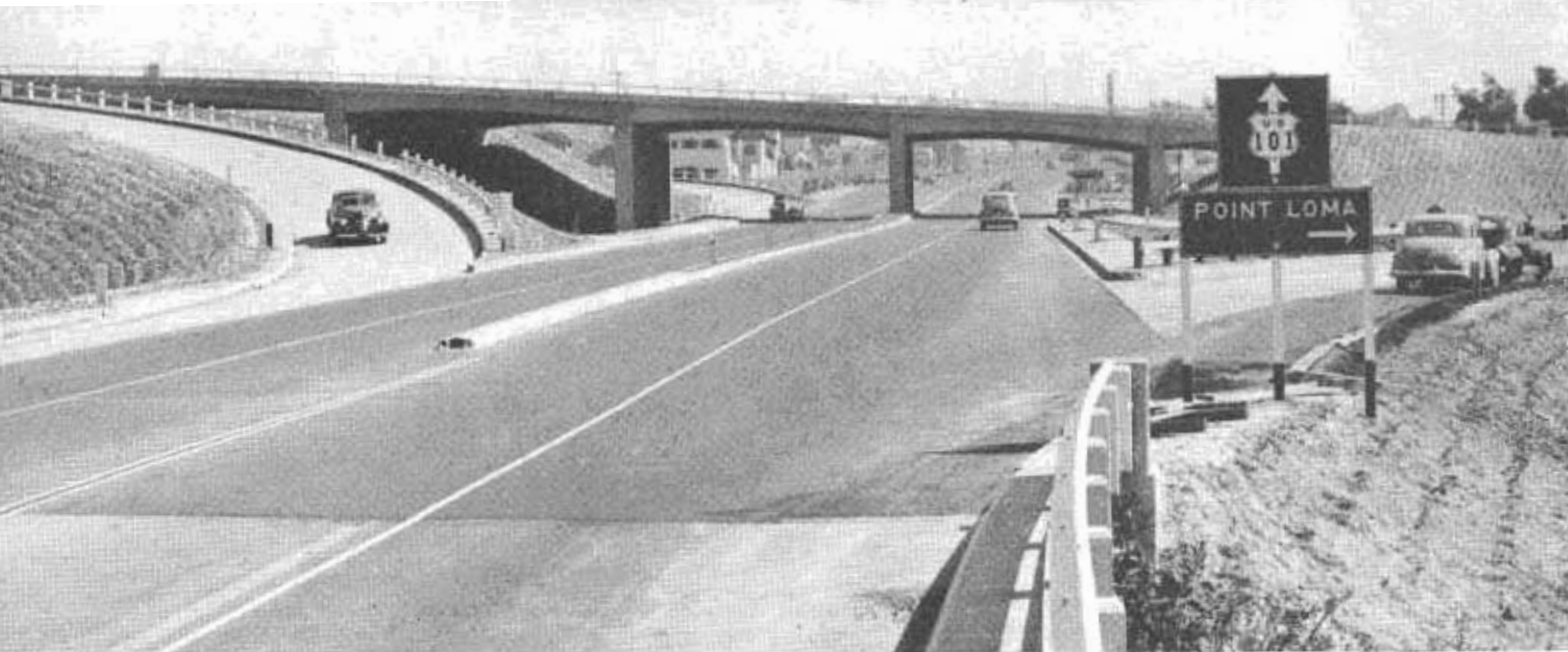
Overpass structure at cloverleaf grade separation of U. S. 101 and Mission Valley highways in San Diego
