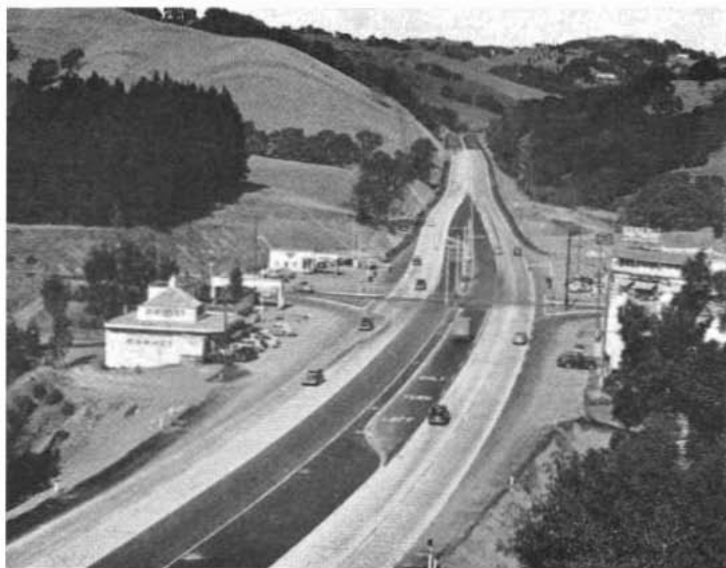
Orinda Junction on Sign Route 24, Oakland-Walnut Creek arterial, has full traffic signal control and channelization
