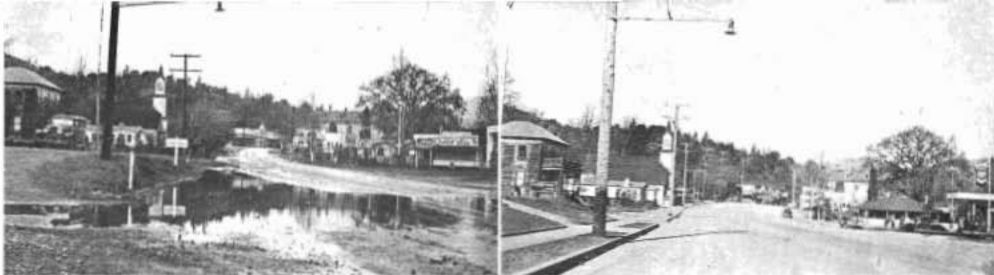
Before and after views on recently improved section of Redwood Highway in the city of Hopland
