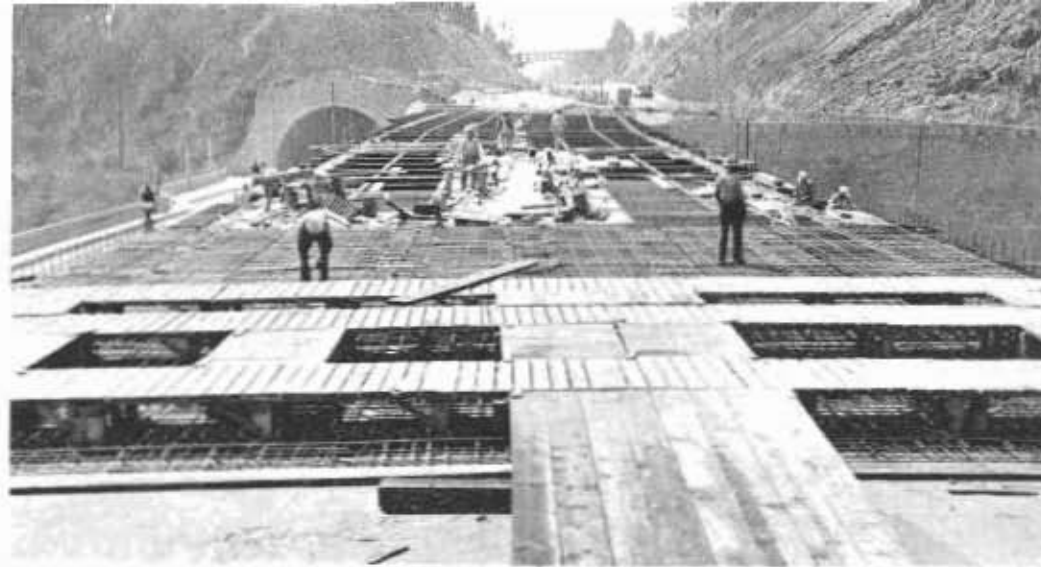
Steel construction on bridge section fast approaching completion
