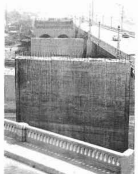
New bridge parallels existing structure
