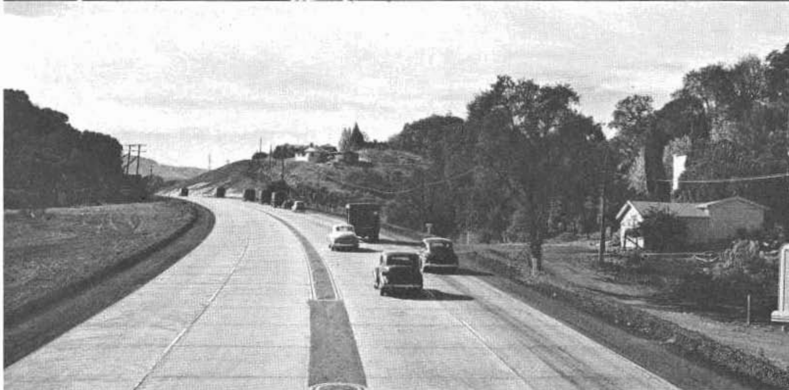
At top, slide section of State Sign Route 24 rebuilt as 4-lane asphalt concrete highway with hydrauger pipe drainage and 3-inch median bars. Below, section over Charles Hill with two 23-foot lanes of Portland cement concrete and 4-foot asphalt concrete dividing strip
