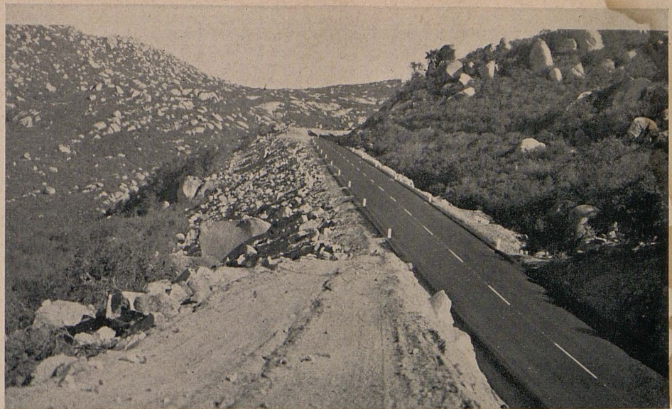
Mile and a half stretch of 7 per cent grade on new highway through boulder covered hills
