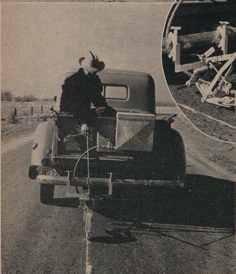
Top picture shows pointer assembly attached to front bumper of truck enabling operator to follow straight line. Center inset shows marking wheel attached to rear bumper and below workman controlling paint valves and wheel lifting lever
