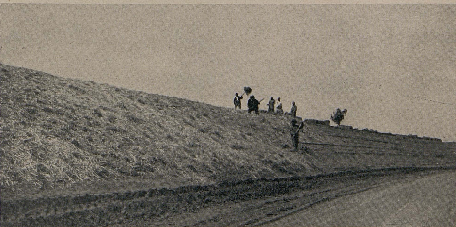
Spreading straw over top soiled slope to provide a mulch
