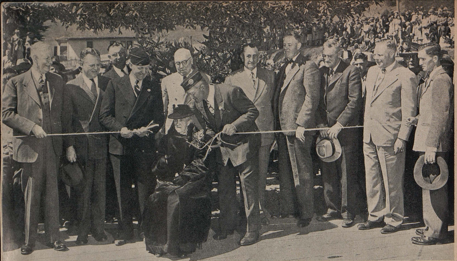
Pioneer of Mendocino County, Mrs. Marian A. Haarby, severs hempen cord, signaling opening to traffic of new Albion River bridge. Left to right, Highway Commissioners James Guthrie and Harrison R. Baker; Lyle Kirkpatrick, Chairman Lake County Board of Supervisors; Martin Haarby; C. H. Purcell, Director of Public Works and Chairman of the Highway Commission; Albert Haarby; Commissioners Homer P. Brown and Chester H. Warlow; State Highway Engineer George T. McCoy; Commissioner Walter Sandelin and Supervisor James Tocher of Lake County
