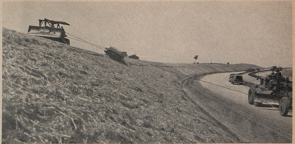
Punching in straw with sheepsfoot roller cabled between two tractors
