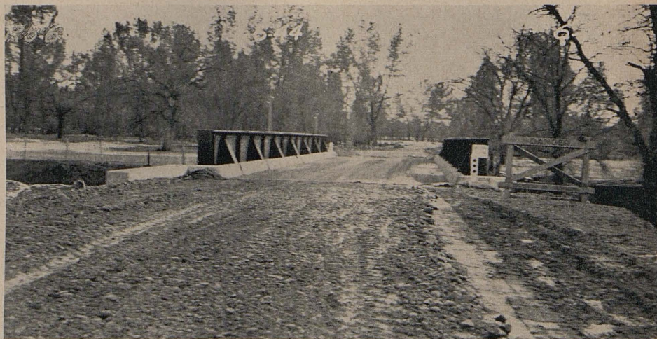
Eighteen-foot solid paved roadway now carries highway across Oak Run Creek
