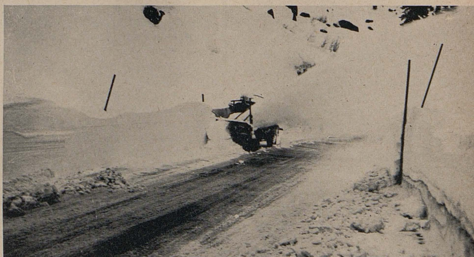
A powerful rotary plow hurls snow high over the Donner road to the opposite bank
