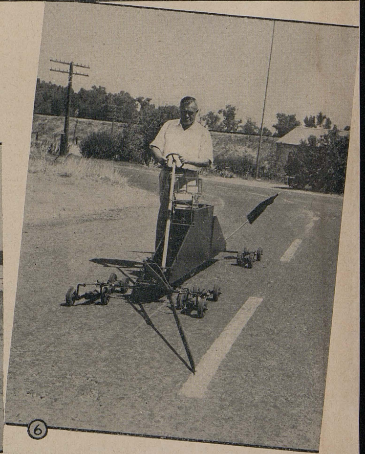
1. Units of profilograph machine for measuring pavement roughness. 2. Assembling the frame. 3. Close-up of recording mechanism. 4. Plan view of the machine. 5. Profilograph assembled, ready for use. 6. Profilograph in use
