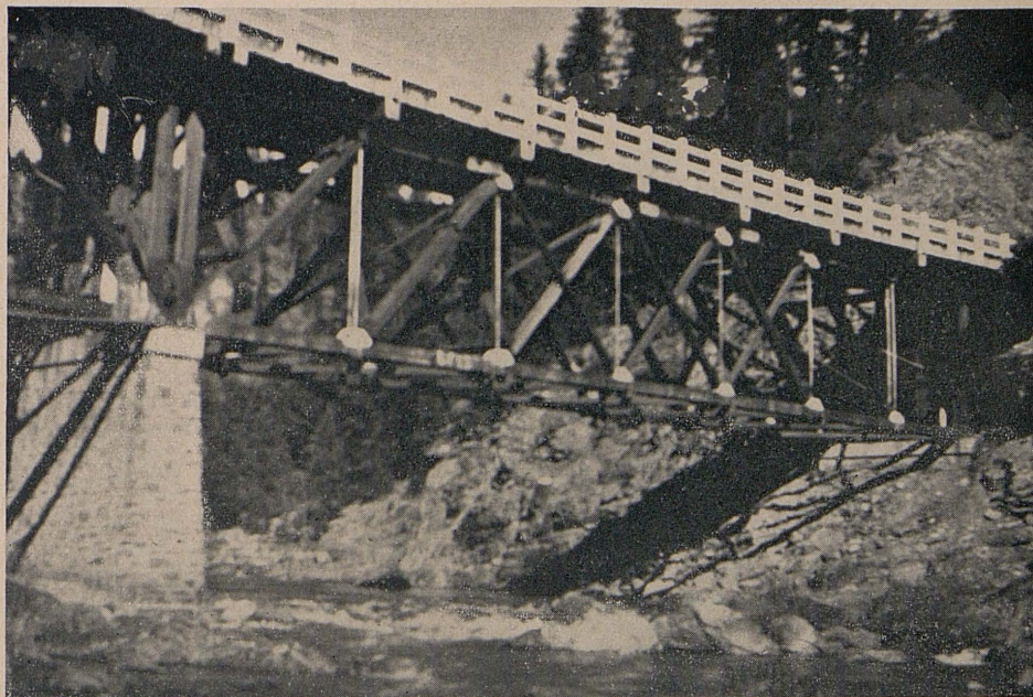
Timber bridge on Feather River Highway showing new concrete bearing blocks on truss members
