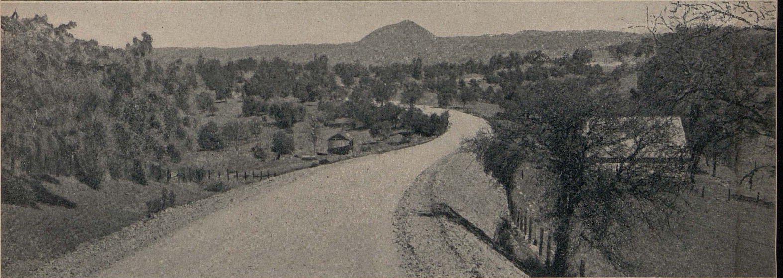
At top—lumber trucks hauling heavy loads over steep grades and sharp turns on old road east of Mokelumne Hill before realignment. Center—big load of logs tops summit of McFadden Hill on new, wide highway. Bottom—view east of Flume House Hill on State Highway 5 where 10 per cent adverse grade was regraded to 7 per cent
