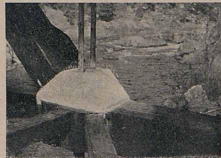
Reinforced concrete bearing block with 2 steel hanger rods through the center
