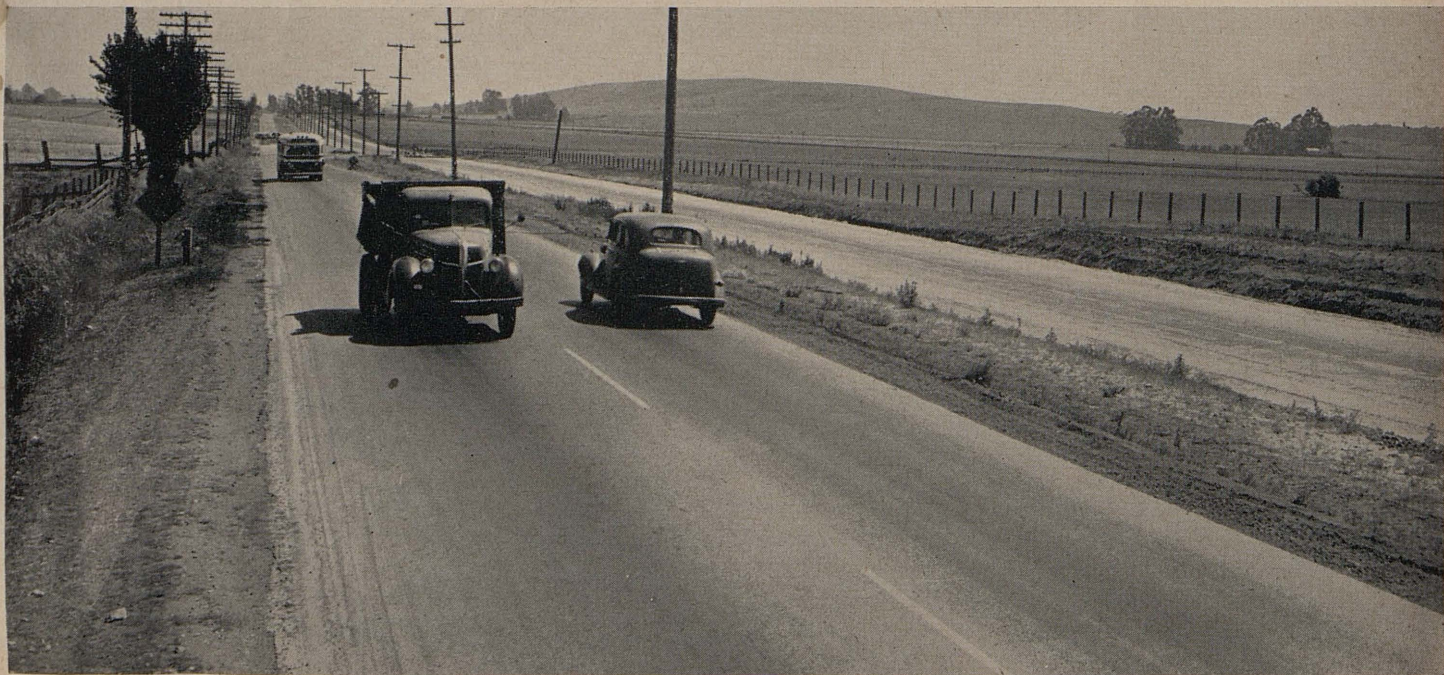
View of new four-lane highway between Napa Wye and Vallejo before paving operations. New lane is on right
