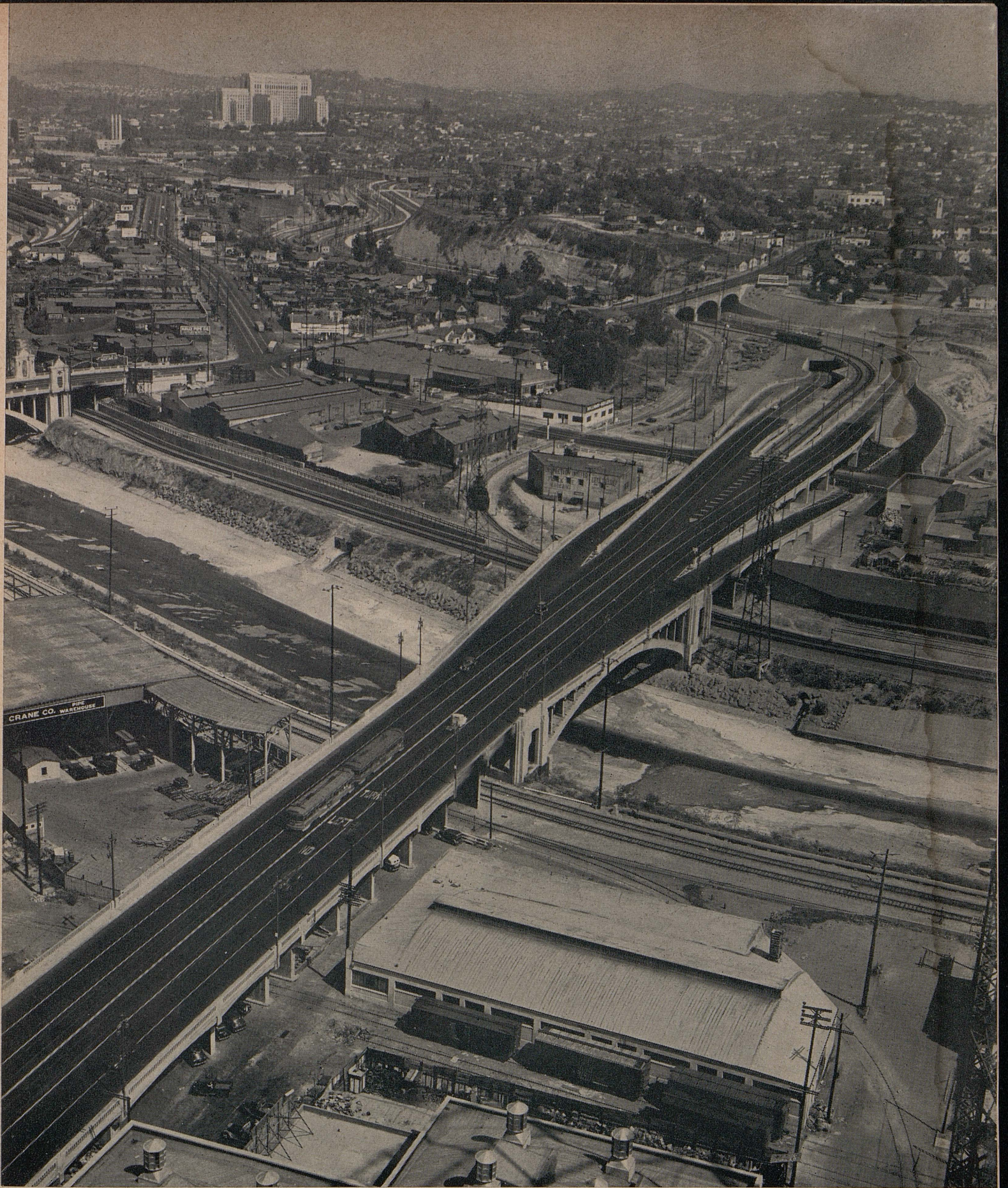
Recently completed $5,000,000 Aliso Street Viaduct across Los Angeles River in Los Angeles, showing connections with important freeways
