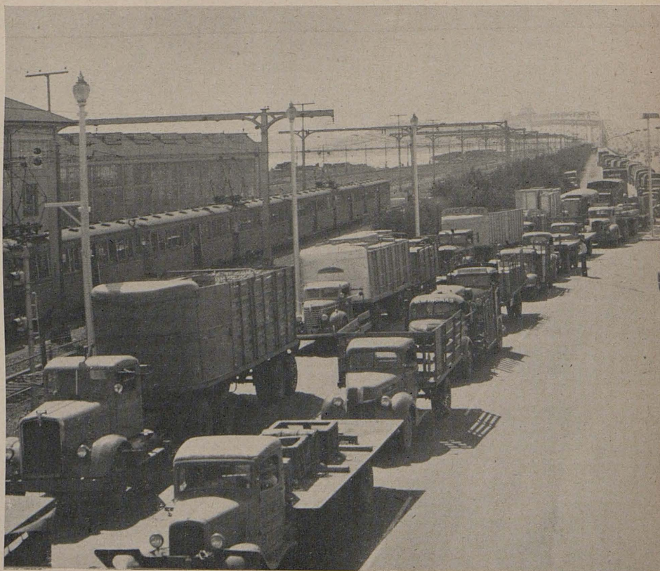
Before Improvement—Two lane lower deck roadway on Bay Bridge blocked by waiting trucks
