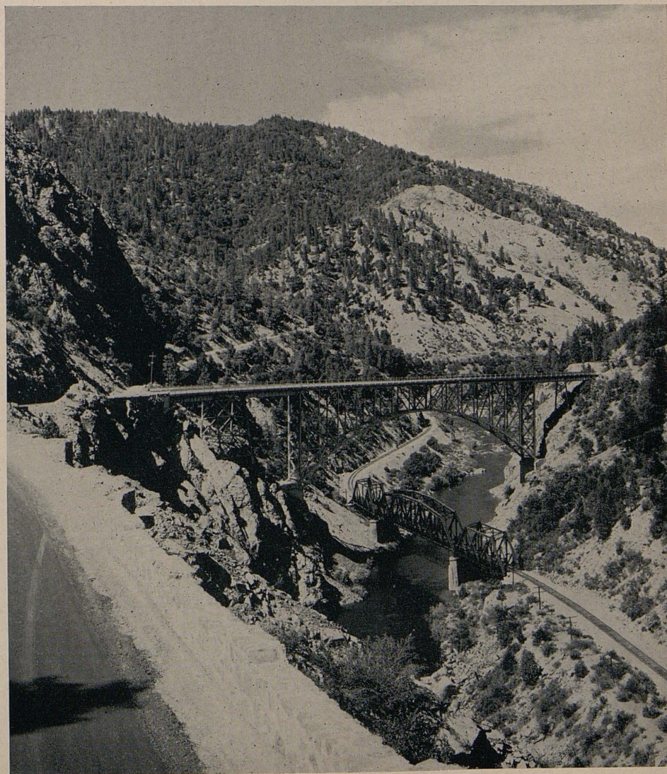
One of the unusual features on the Feather River Canyon Highway is the overcrossing by the State Highway Bridge of the Western Pacific Railroad Bridge at Pulga
