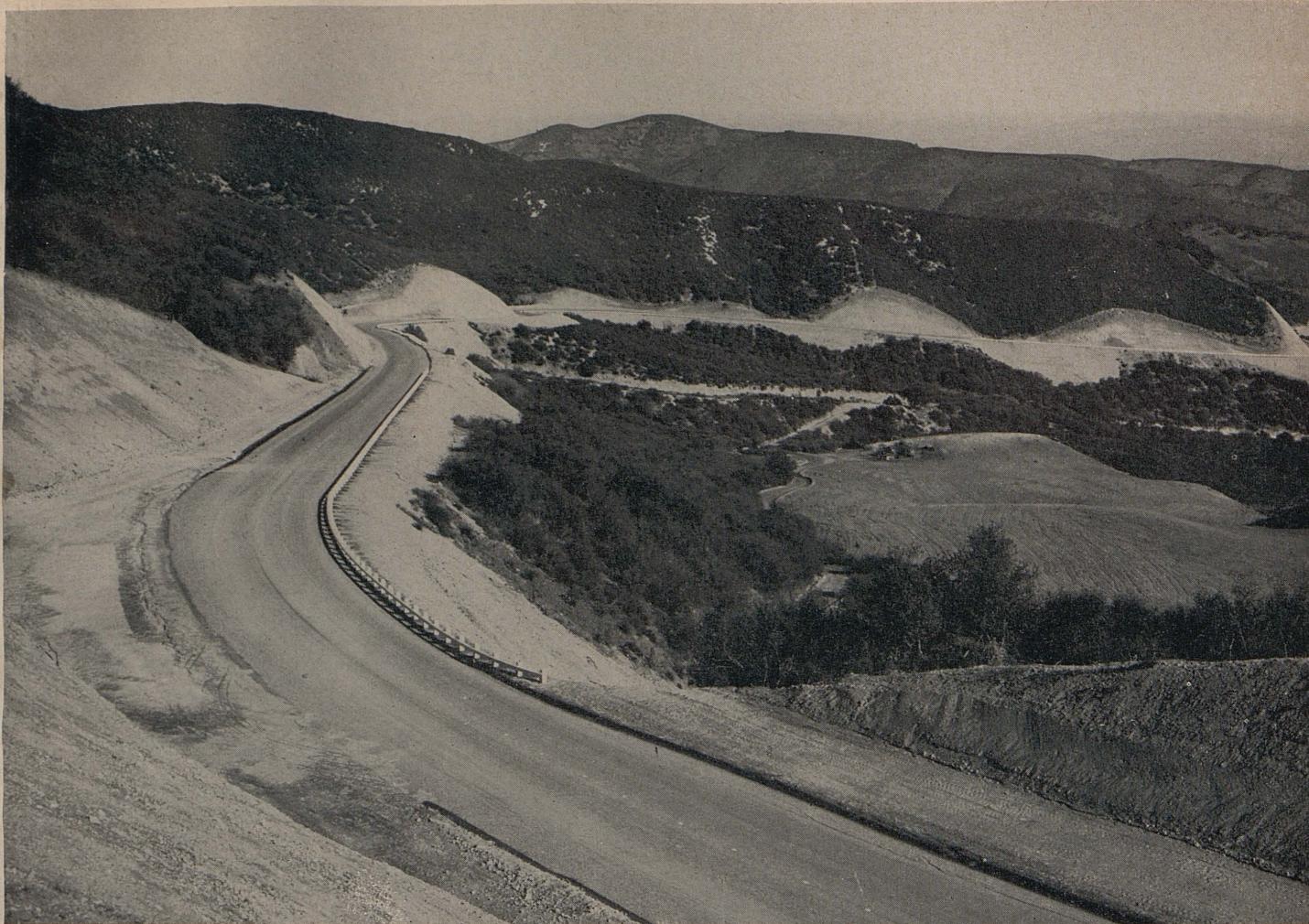
Casmalia-Santa Maria Access Road. On the horizon at the right may be seen the big cut which is 100 ft. deep and contained 240,000 cu. yds. of excavation
