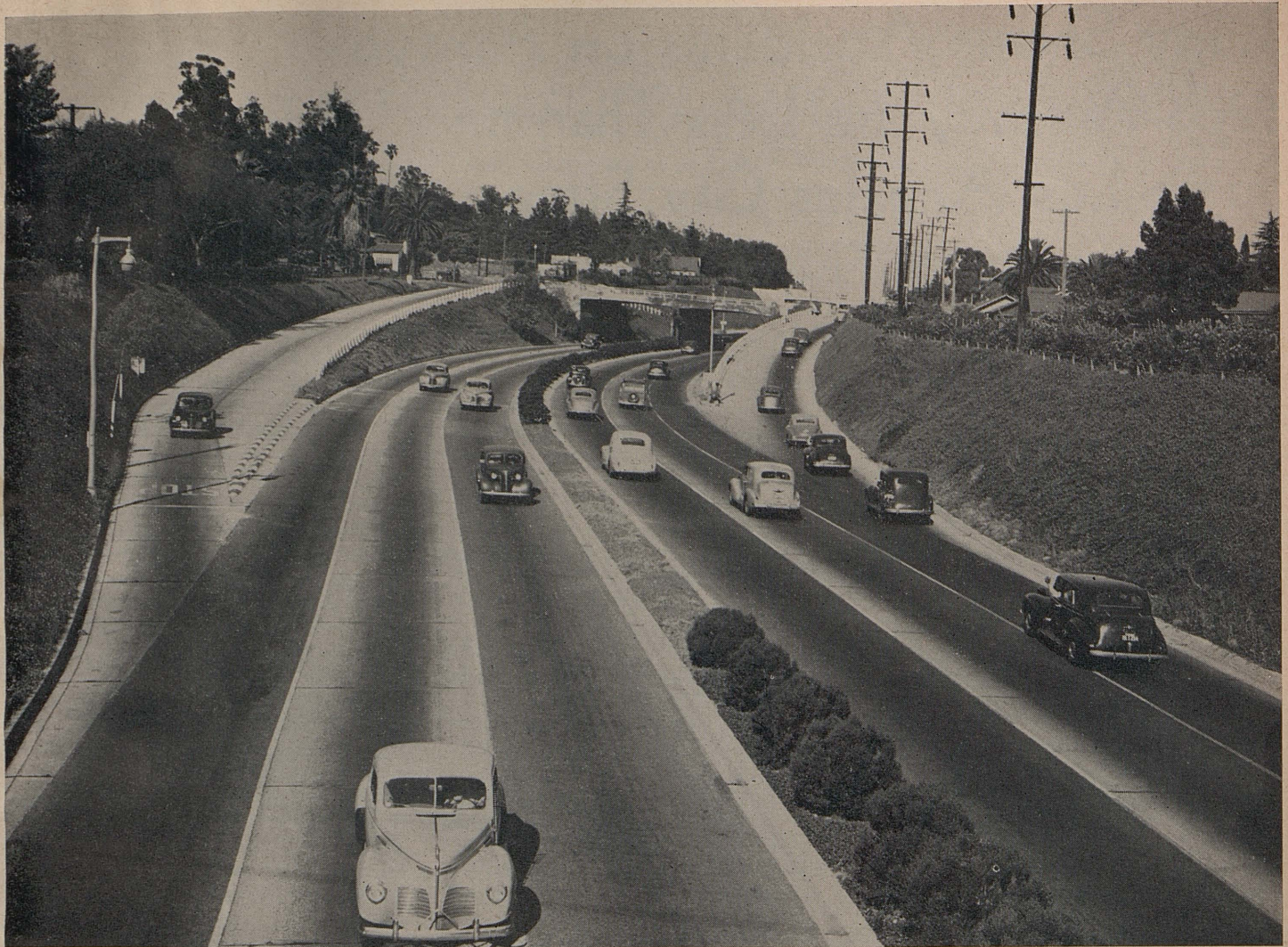
Traffic is safely handled on Arroyo Seco Parkway with divided lanes, overheads and on and off ramps
