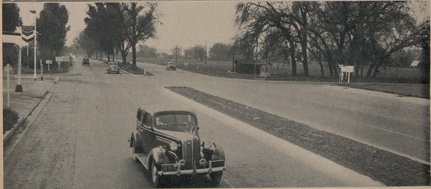
Upper—U. S. Highway through Tuggleville, southerly approach to city of Tulare, where uncontrolled vehicle movements cause many accidents. Center—Unsightly business development along major traffic artery south of Tulare, where accidents frequently occur. Lower—Looking westerly from west city limits of Visalia. This entrance to Visalia is almost entirely free of roadside developments.
