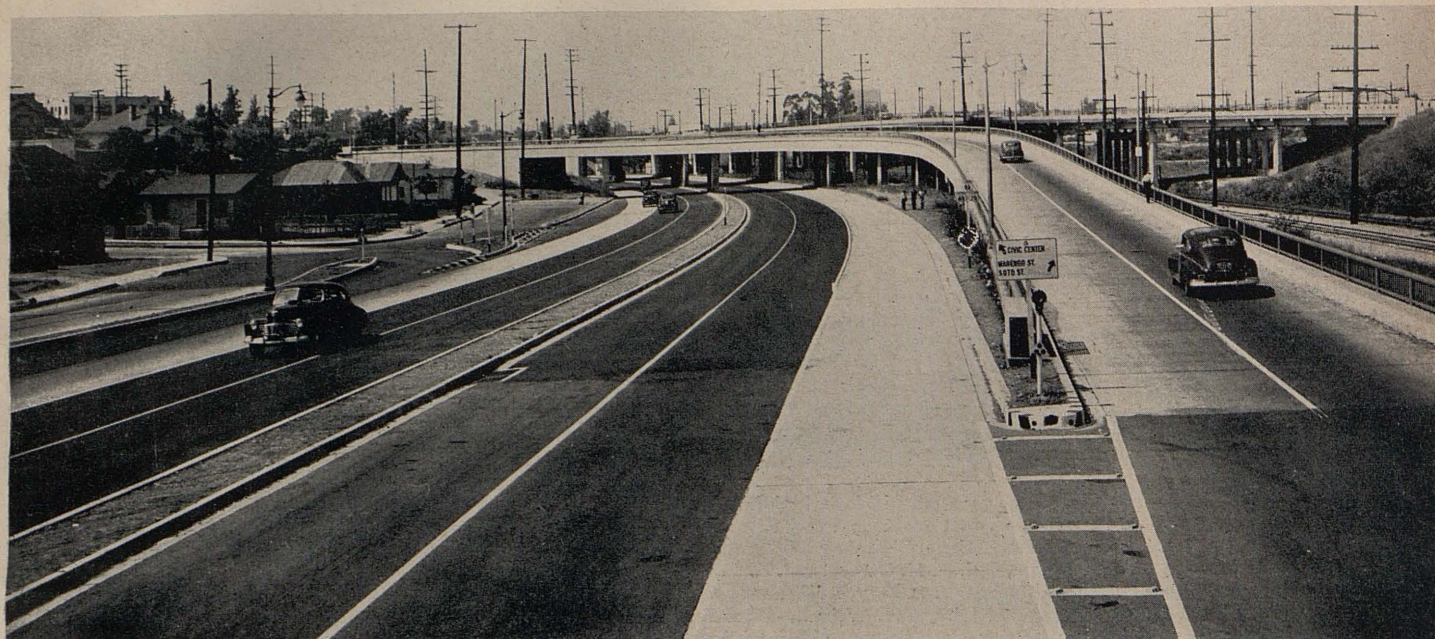
This photo shows Pomeroy Street Off-Ramp. The view is looking west on Ramona Freeway. The off-ramp to Soto Street starts on right and crosses freeway. Soto Street overhead crossing in background
