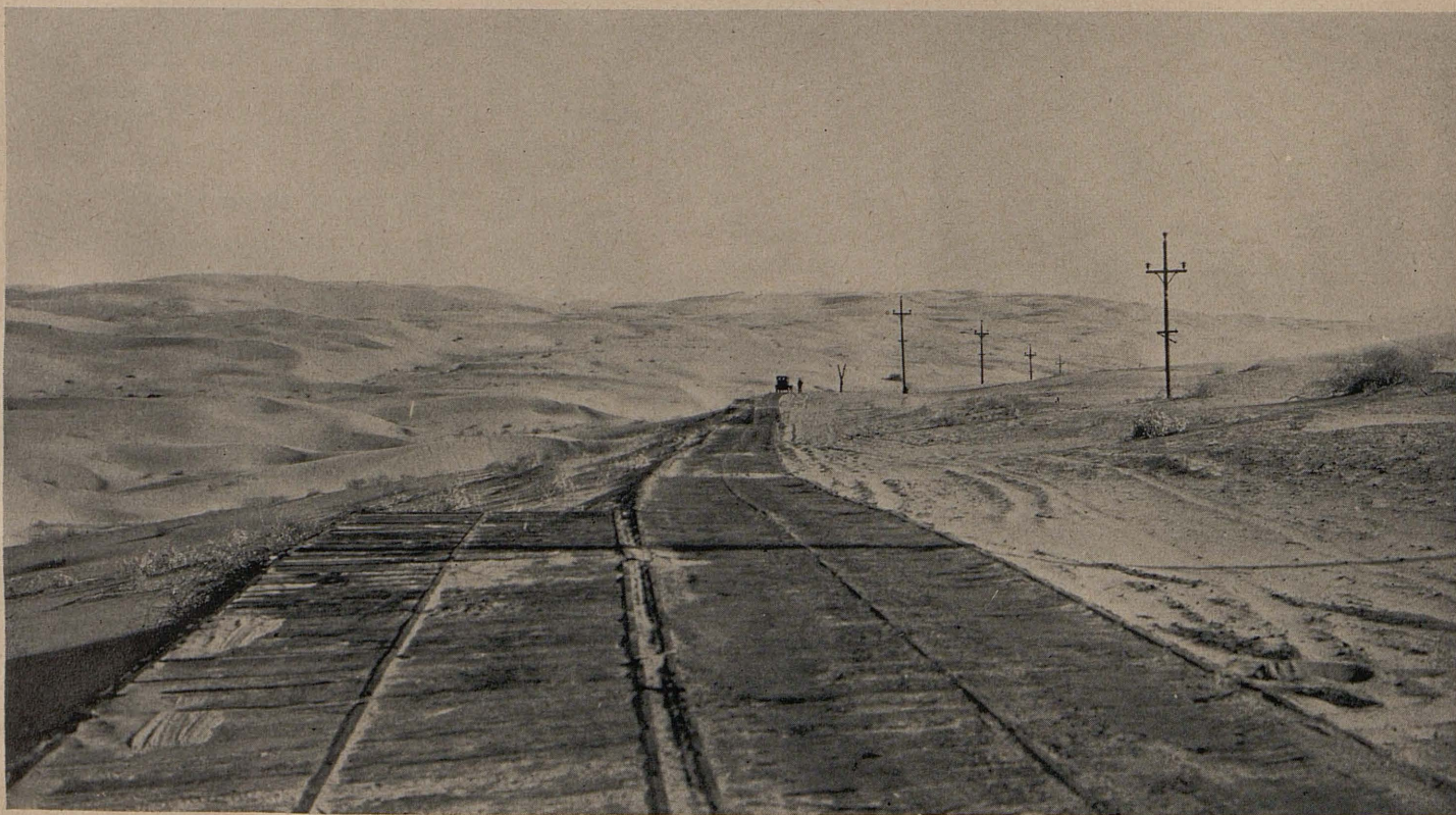
This corduroy road carried vehicular traffic across the Yuma sand dunes west of Open Valley in Imperial County for many years following its construction in 1915-16. Note plank turn-out for traffic on left
