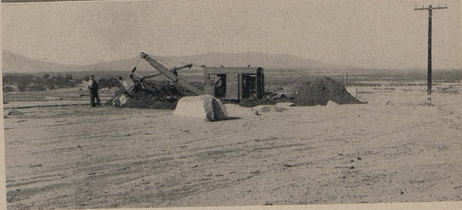
Top—This photo shows bus washed 1,000 feet from highway on State Route 23 in Inyo County. Center—Mud and boulders flowed over roadbed on State Route 23 in Kern County. Bottom—Shovel at work locating debris-covered roadway on State Route 23 in Kern County
