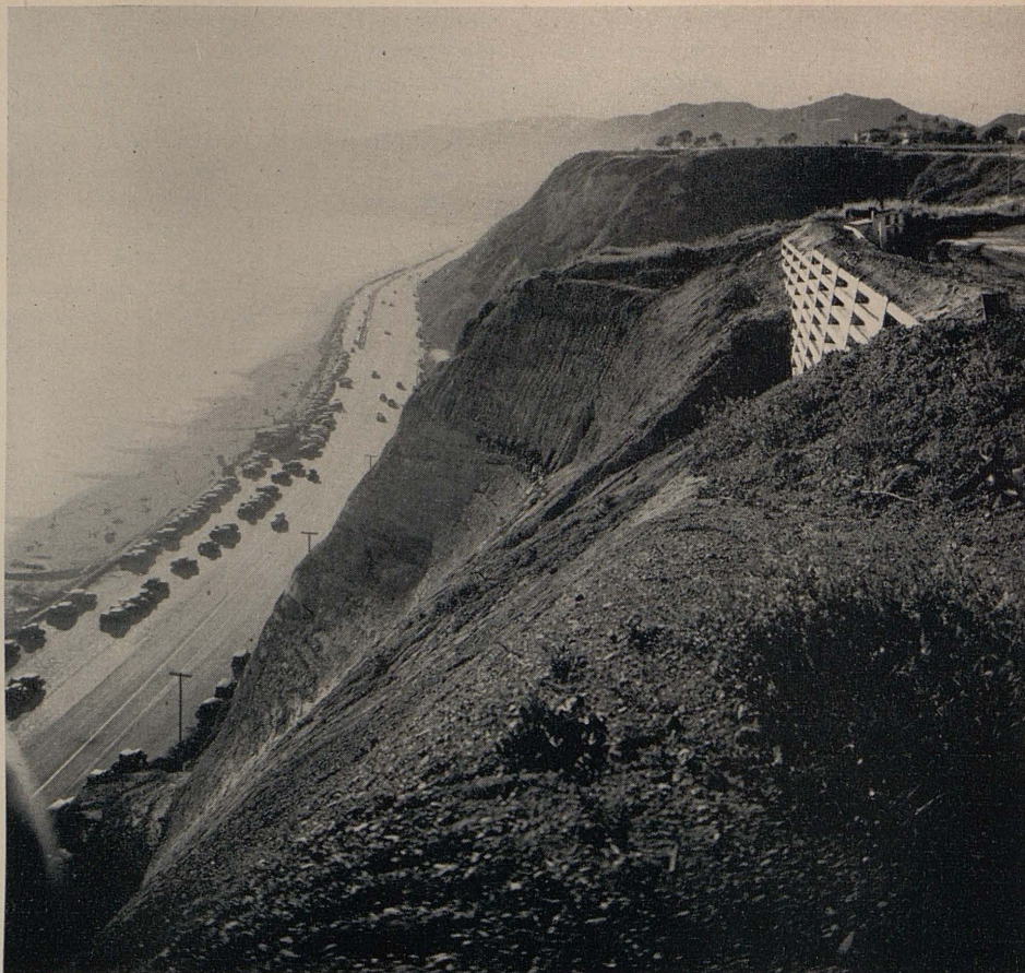
Scene on Santa Monica Highway showing precipitous bluffs which engineers had to overcome
