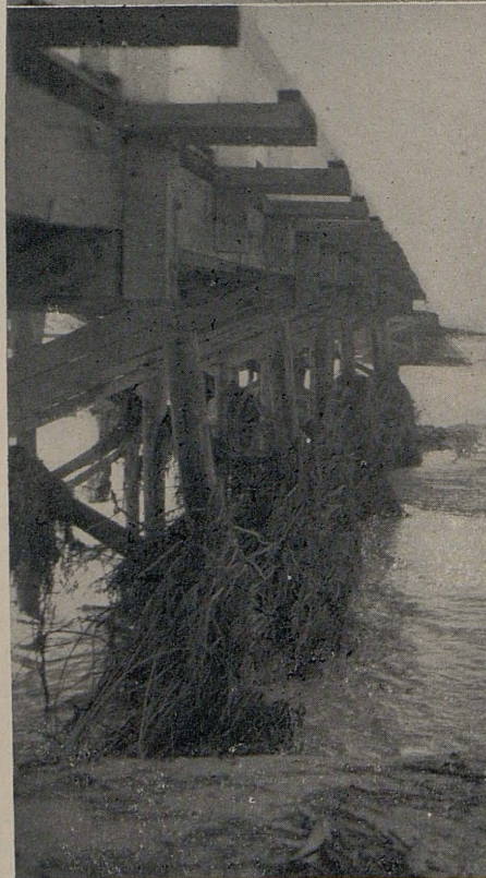
Upper—View of San Felipe Bridge showing washed out section after flood subsided. Lower—View of washout from upstream side showing debris accumulated on pile bents
