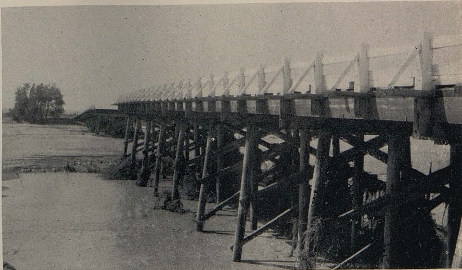
Upper—View of San Felipe Bridge showing washed out section after flood subsided. Lower—View of washout from upstream side showing debris accumulated on pile bents
