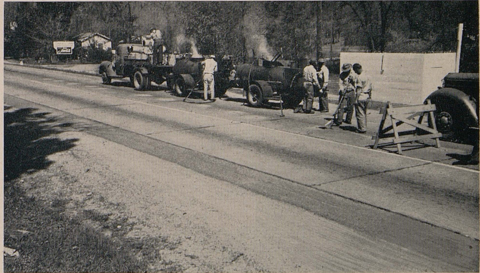
Here is a subsealing crew with equipment
