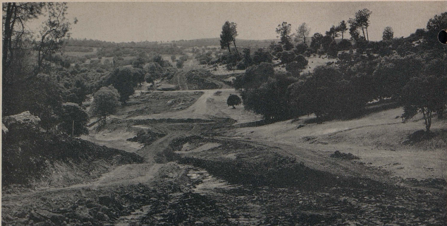
Looking from Windmill Hill toward Shingle Springs, showing clearing and old pioneer grading. Existing highway in middle ground
