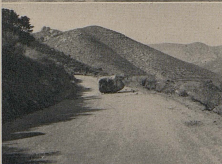
These photos show some of the larger rocks which blocked State Route 57 following earthquake jolts
