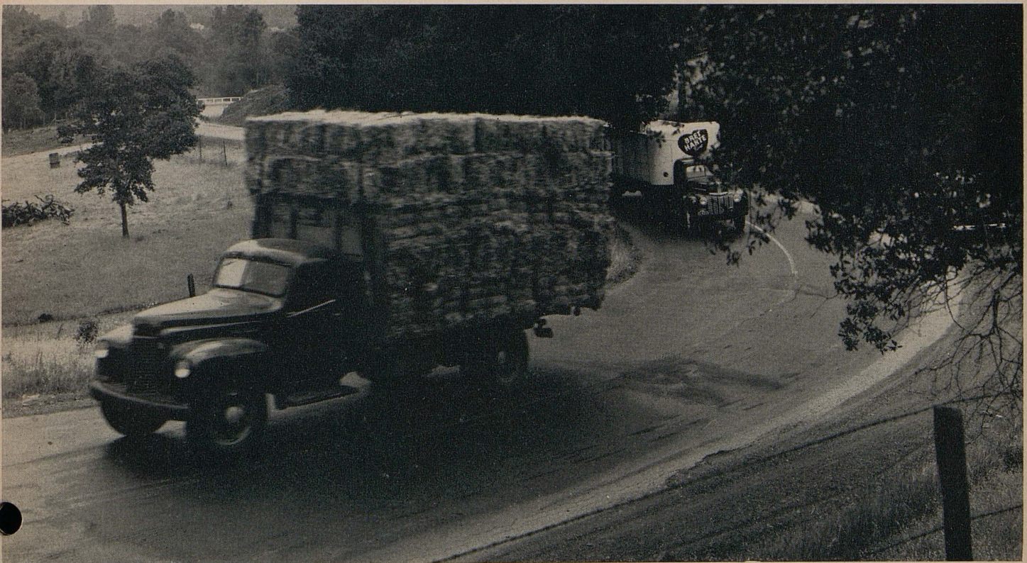
This hazardous curve is typical of many on U. S. 50 which will be eliminated by realignment
