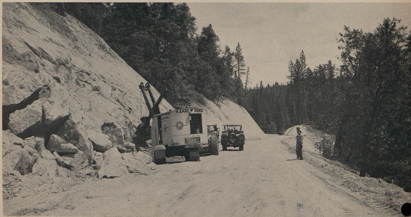
Heavy rock excavation in progress on realigned section of State Route 25
