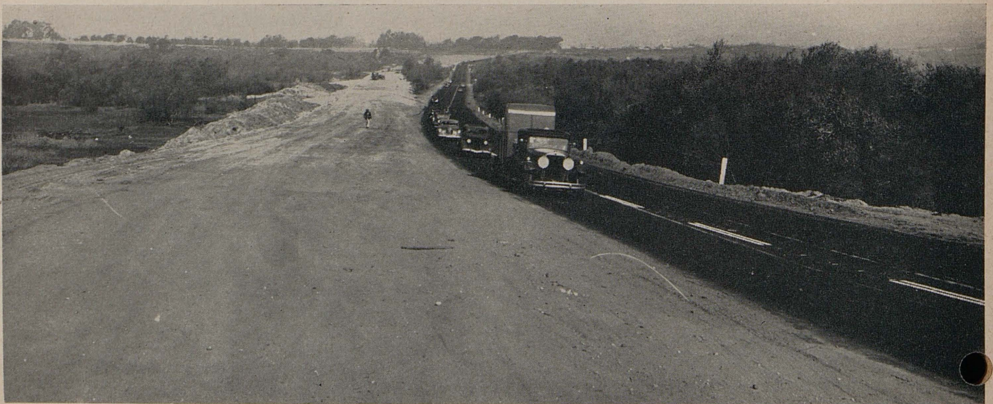
Realignment for southbound traffic across San Mateo Creek Valley
