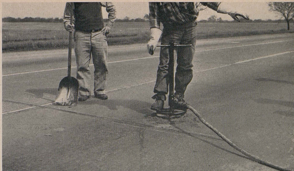
Type of expanding nozzle used for asphalt subsealing
