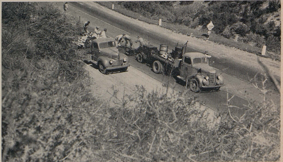
Asphalt subsealing crew of Division of Highways at work
