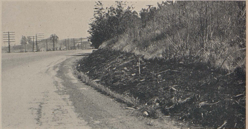
Burned firebreak on a cut slope from the gutter line up
