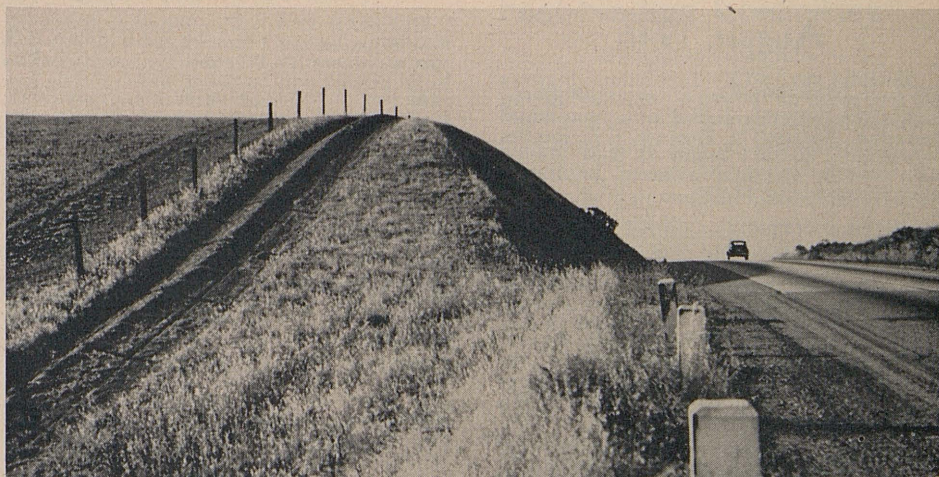
An improved control is provided by a burned firebreak placed from the gutter line up on cut slope
