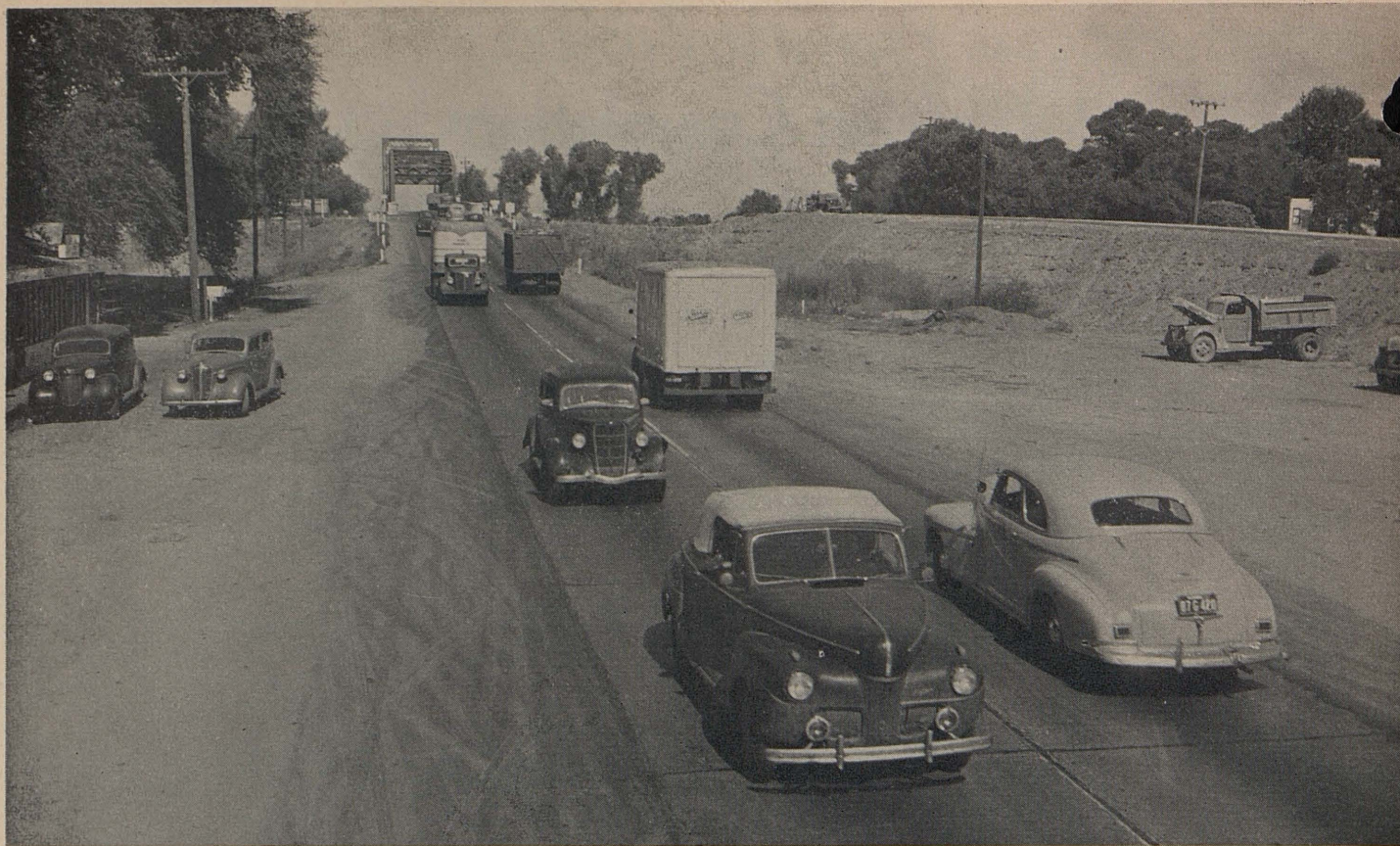
This sort of congestion will be relieved by new highway shown on elevation at right. View is on east end of project with traffic approaching Mossdale Bridge. A second bridge will be built for east-bound traffic
