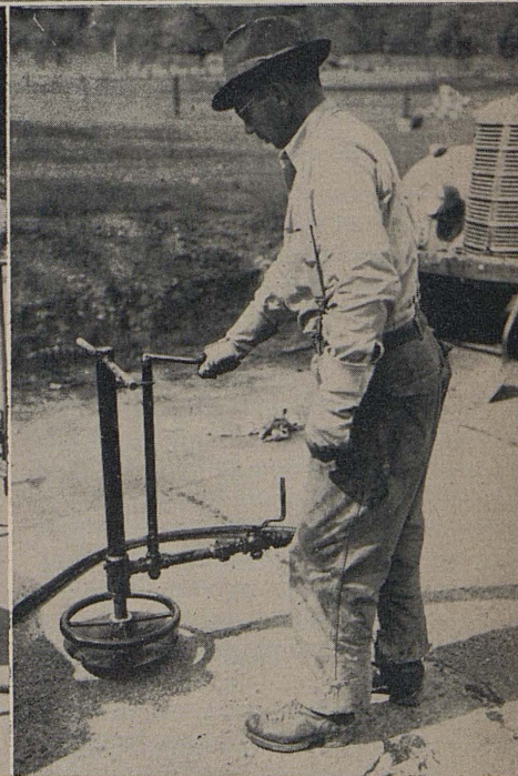
Three types of nozzles used in asphalt subsealing
