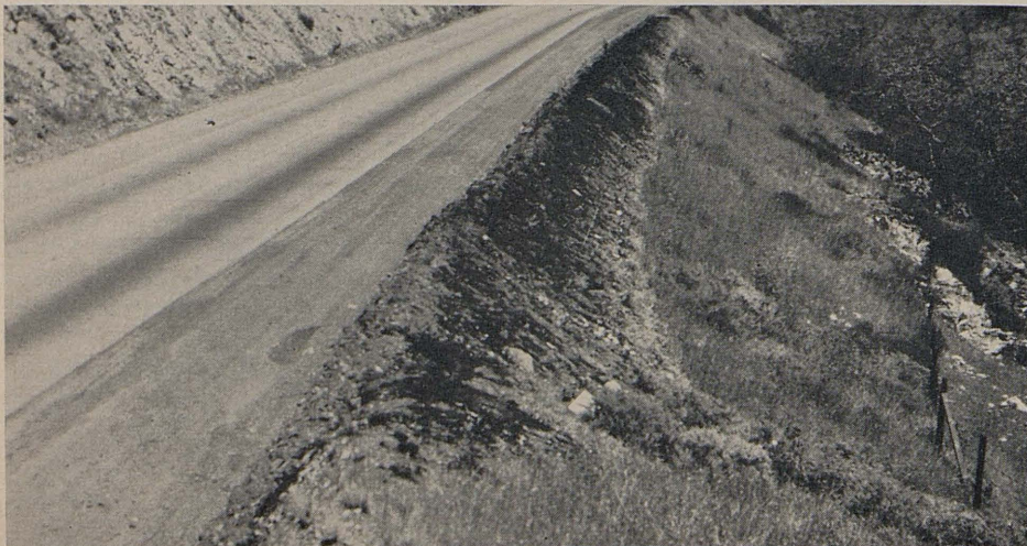
Burned firebreak on a fill slope from the top of the berm out and down
