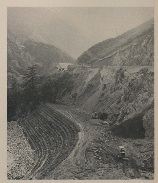
Above—This embankment on City Creek Road which is one-half completed will have an ultimate height of 110 feet. On opposite page, upper—Portion of 50-foot high embankment under construction, showing erosion protection features. Lower—Progressive work on sidehill excavation utilizing ramps within the roadway prism
