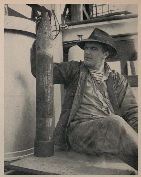
Close-up of jet nozzle. Four-inch pipe reduced to two inches
