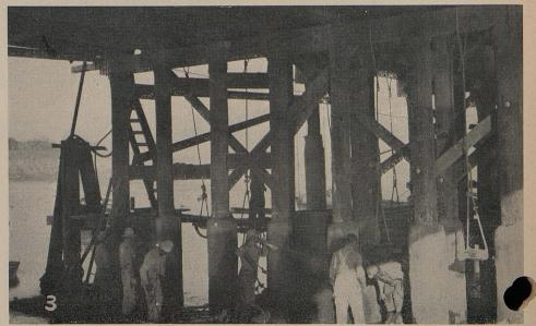
ments were completed. To stiffen the pile bents supporting the bulkhead, in foot "gunite" diaphragm walls built between groups of three four piles in these bents.
