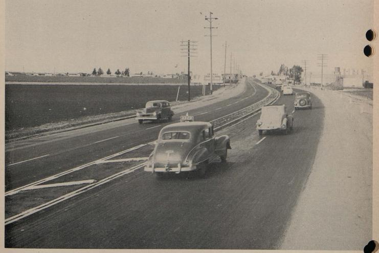
Raised bars in central division strip on transmission from two-lane to four-lane divided highway
