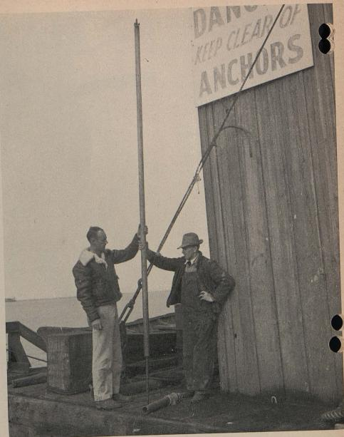
Sampler tube. This tube is weighted with lead to resist bouyancy
