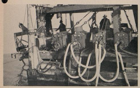
Pumps used to develop high water pressure for jetting
