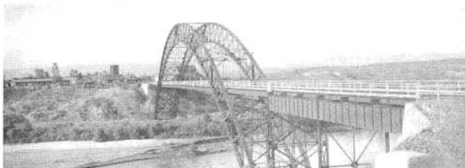
Old Trails Arch (Bridge 54-18) over Colorado River before Lake Havasu flooded the lower hinges. Topock, Arizona, in background
