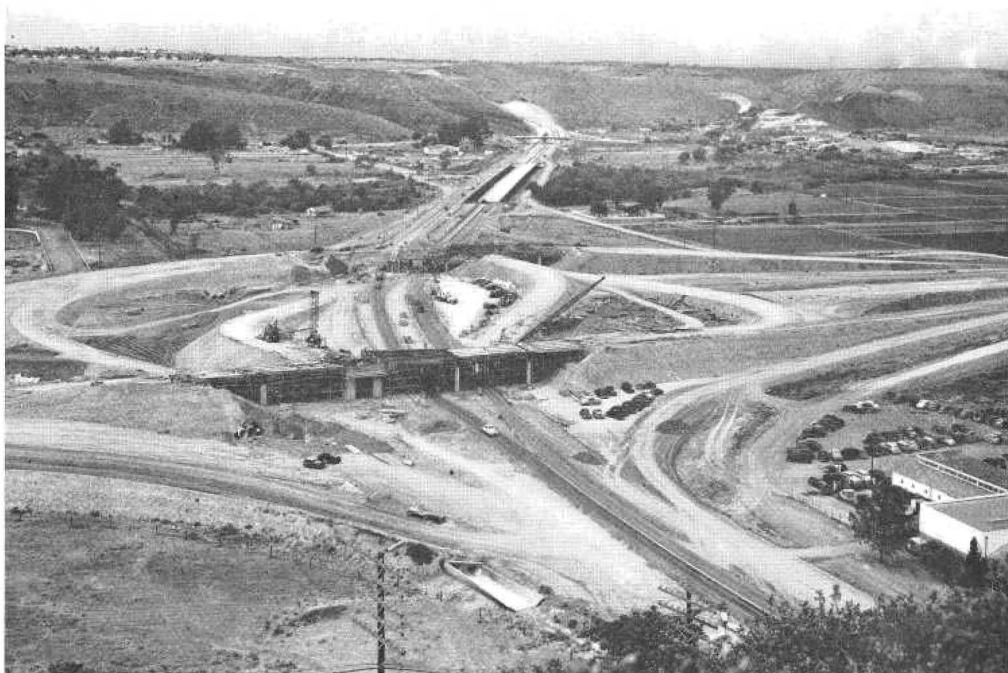
Looking north across Mission Valley and showing interchange and San Diego River bed
