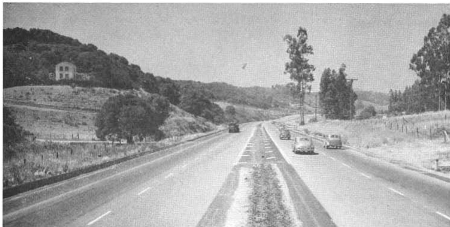
View of transitions on four-lane divided highway where existing concrete pavement changes from right to left set of lanes. Central dividing strip defined by traffic stripe and raised bars
