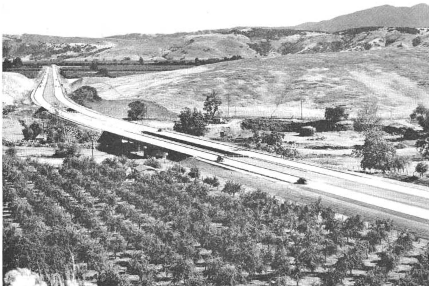
Near its southern end, where it joins El Camino Real at Ford Road seven miles south of San Jose's central business district, the New Bayshore Freeway Extension crosses Coyote Creek on a center-tiered span and then, at the far left, bridges Coyote Road
