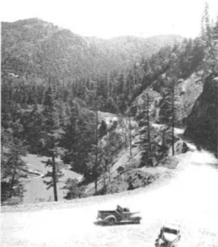
Upper left—Rough grading is nearing completion on this rocky section of the Trinity River highway east of Cedar Flat, where much drilling and blasting is necessary. Lower left—Improvement of U. S. 299 across Gray's Bluff is about complete, except for oiling. Upper right—This winding, narrow section of U. S. 299 along Trinity River, near Salyer, is scheduled for early realignment and widening. Lower right—Steep, rocky bluffs are encountered in grading operations along much of the Trinity River Route
