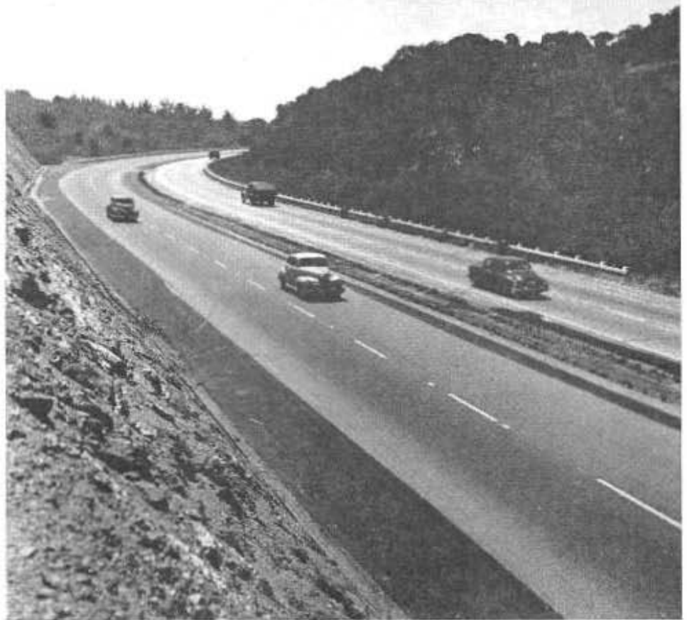
Upper—View showing erosion protection on embankment slope. Lower—Typical view of new four-lane divided highway developed from existing two-lane highway
