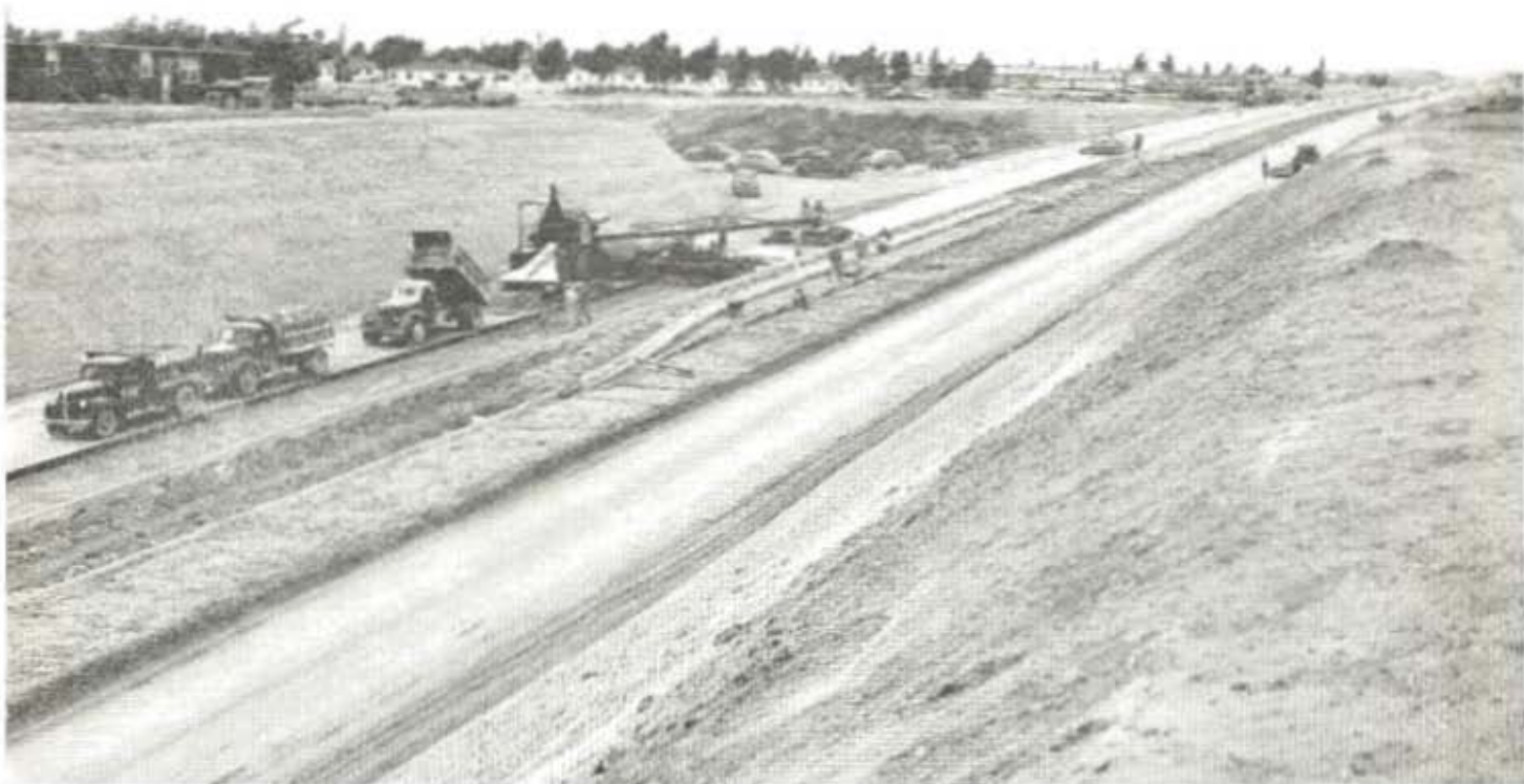
Lower—Concrete paving operations through Linda Vista
