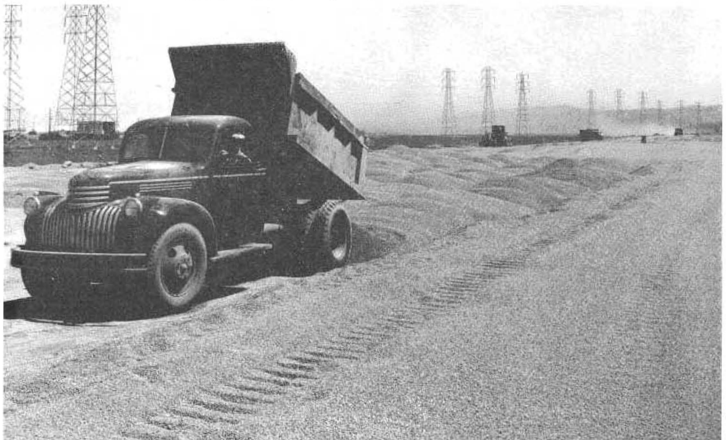
Here a five-yard truck is spreading sand blanket over sand drains
