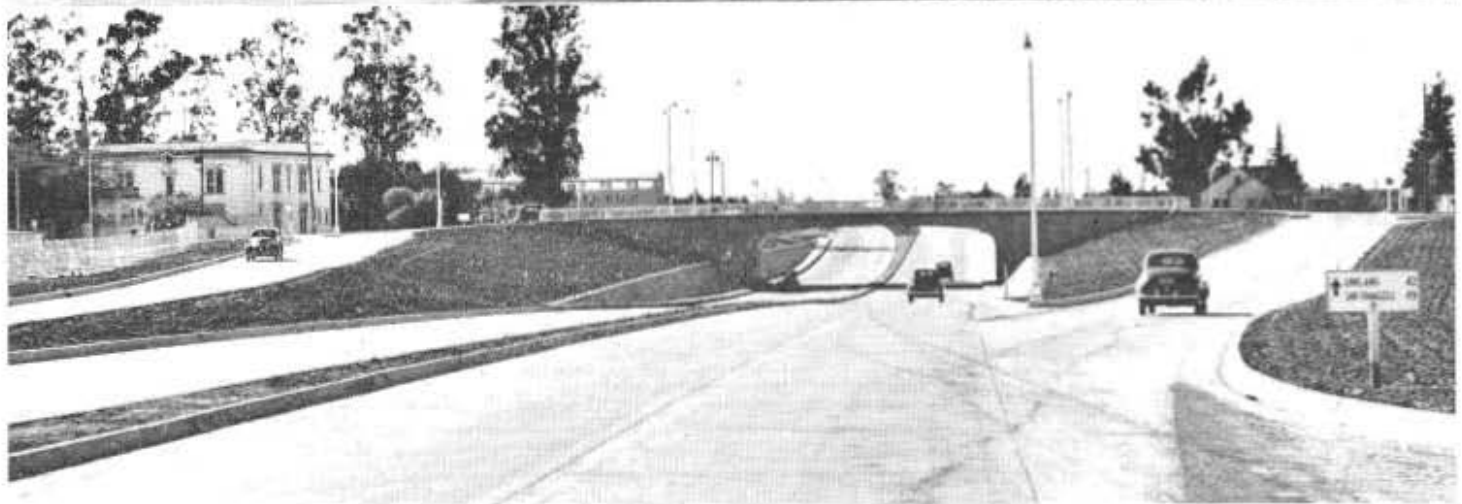
Upper—Northbound motorists approaching San Jose must enter the Ford Road Interchange at the southern terminus of the new Bayshore Freeway Extension, where it joins El Camino Real. Here they have the alternative of turning left, under the overhead structure, toward the business district of San Jose, or proceeding straight ahead along the freeway extension, which passes through the outskirts of San Jose on the way to San Francisco or Oakland. Center—Approximately midway in the new Bayshore Freeway Extension, passing through the outskirts of San Jose to connect Bayshore Highway with El Camino Real south of the city, is this gentle, 3,000-foot radius curve. Lower—Near its northern terminus the new Bayshore Freeway Extension, skirting San Jose in connecting Bayshore Highway with El Camino Real to the south of the city, passes through the Santa Clara Avenue interchange structure. In this view, looking north, the freeway leads straight ahead to San Francisco and Oakland, while the road to the right joins Santa Clara Avenue leading west to San Jose's business district or east to Alum Rock Park.
