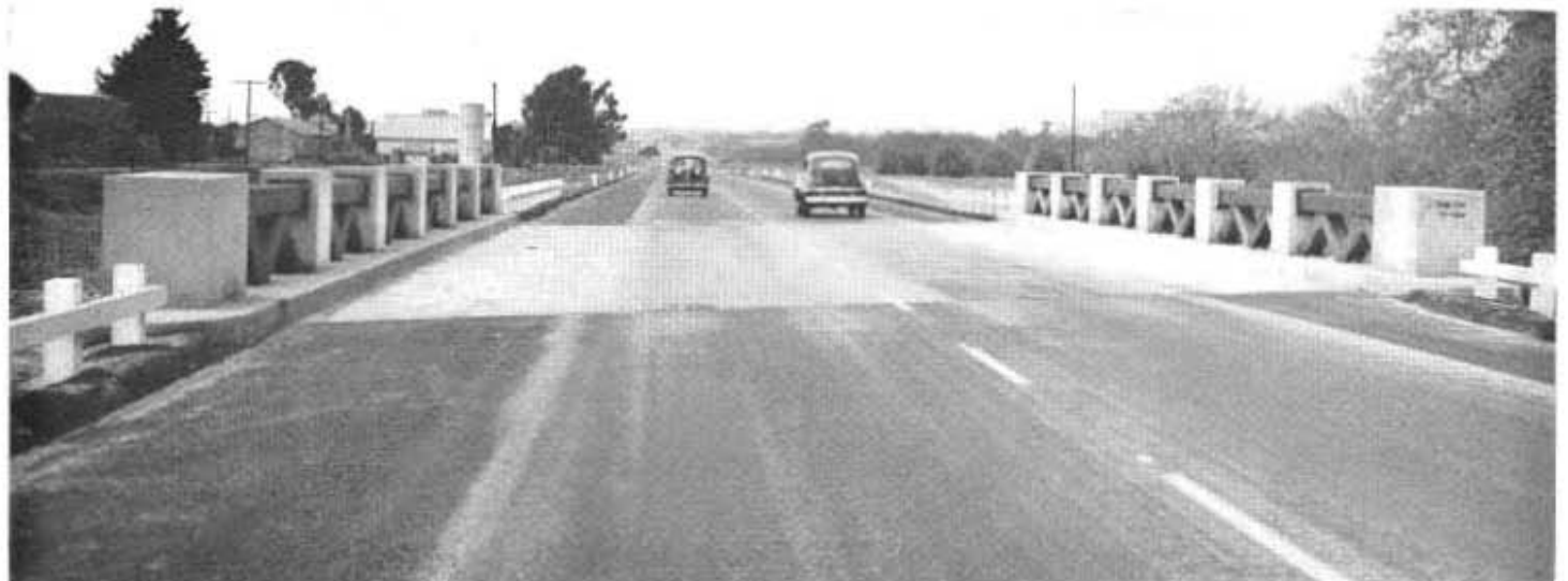
This view is looking northerly along the new location from San Jose Creek Bridge
