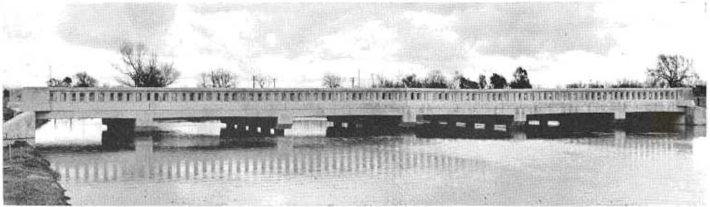
Laguna Creek Bridge. This structure is just north of Elk Grove in Sacramento County and is the first bridge to be completed under the present program. It is a modern reinforced concrete slab structure with a 30-foot roadway and was designed by the county
