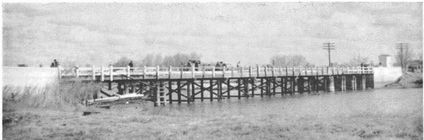
Looking northeast at White's Bridge following record reconstruction
