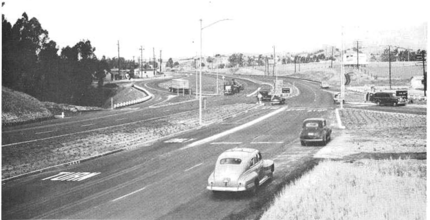
Channelization of Hollister Avenue intersection with signal installation in progress
