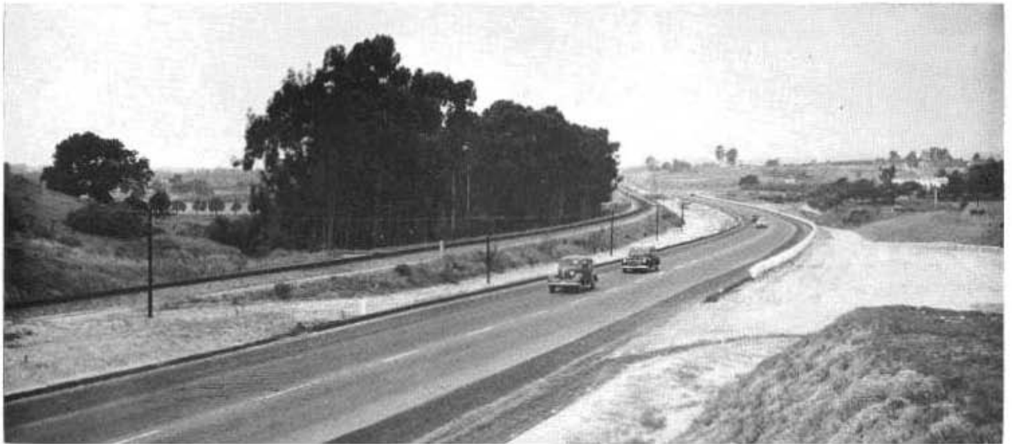
Looking northerly along completed relocation of U.S. 101 in Santa Barbara County
