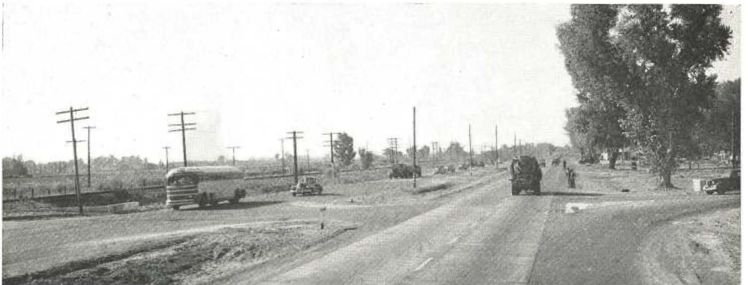
Divided four-lane highway at Buhach, Merced County, showing county road intersection channelization with raised bar island and cross-over between traffic lanes
