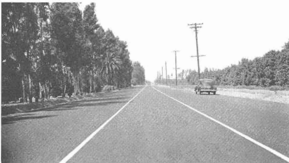
This is another view looking north to 800-foot radius curve
