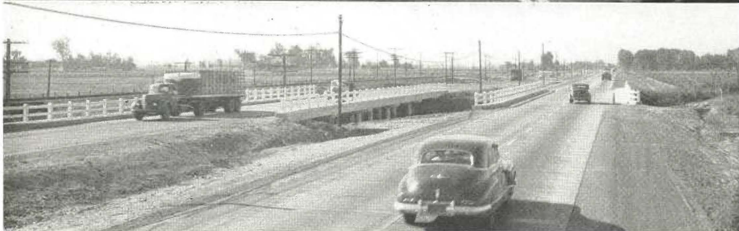
Upper—Traffic using two-lane bridge across Stanislaus River between Salida and Ripon, San Joaquin County. Bridge for additional two lanes to provide four-lane divided highway shown under construction on right. Lower—Twin bridges on four-lane divided highway north of Merced
