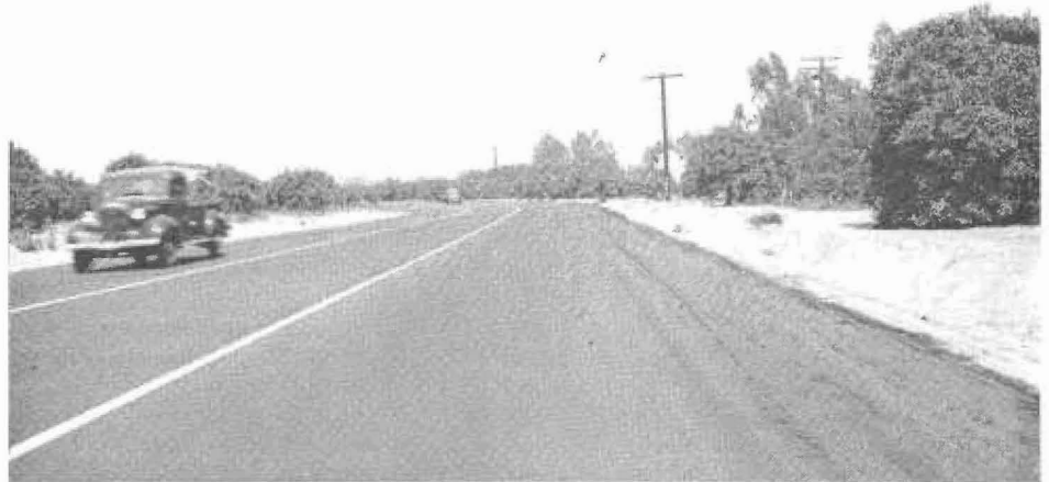
Looking northeast to 800-foot radius curve
