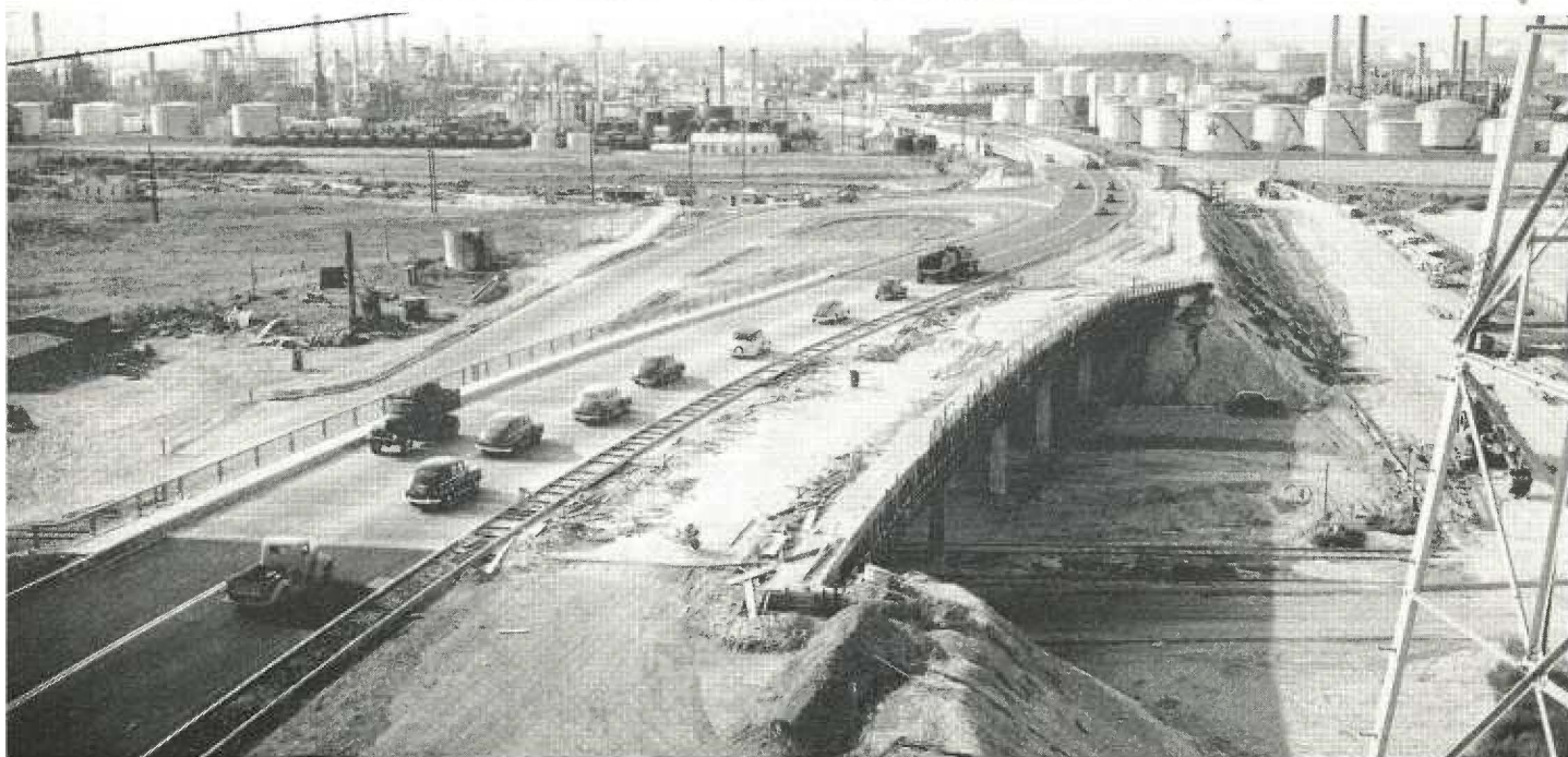
View of Classification Yard overhead. Dominguez Channel bridge in distance
