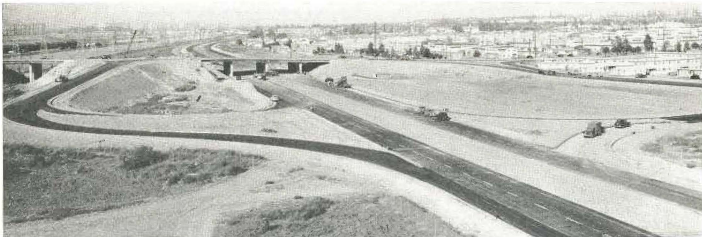
Looking along Terminal Island Freeway toward Los Angeles and Terminal Island Freeway undercrossing
