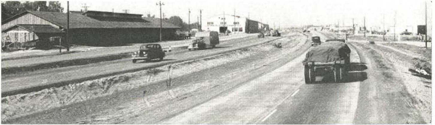
Four-lane divided highway and outer highway on left approaching Salida from south. Note wheel tracks of illegal crossing of divisional strip. Concrete barrier posts will be erected at this location
