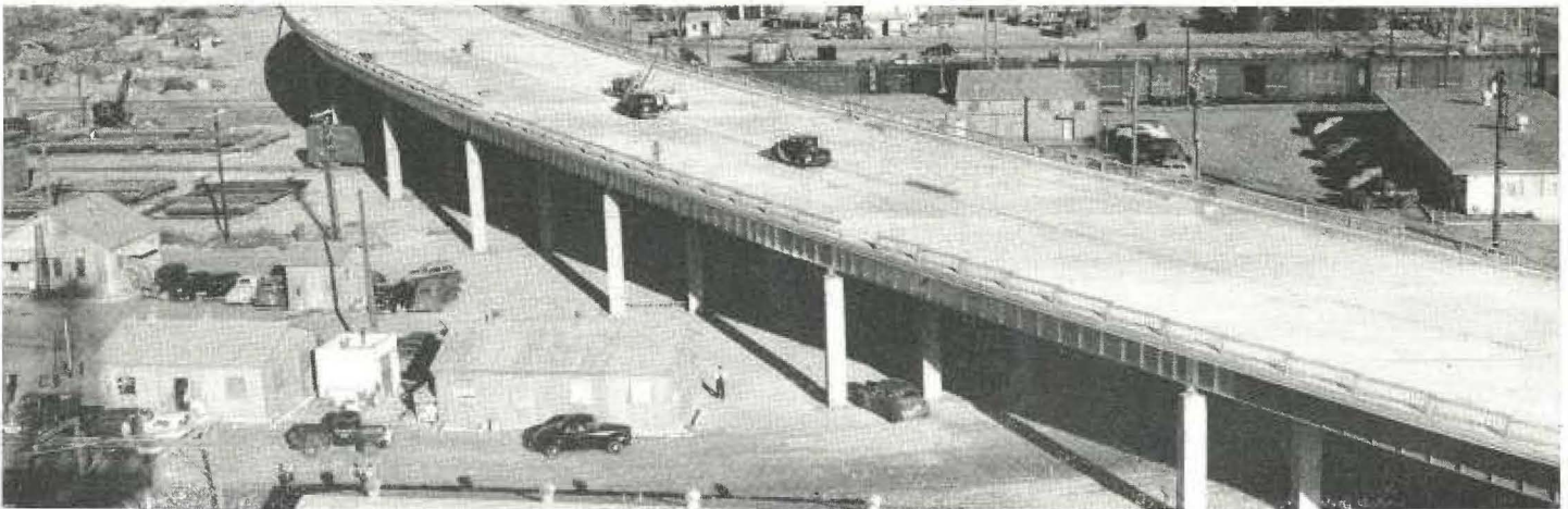
Union Pacific Overcrossing on Terminal Island Freeway
