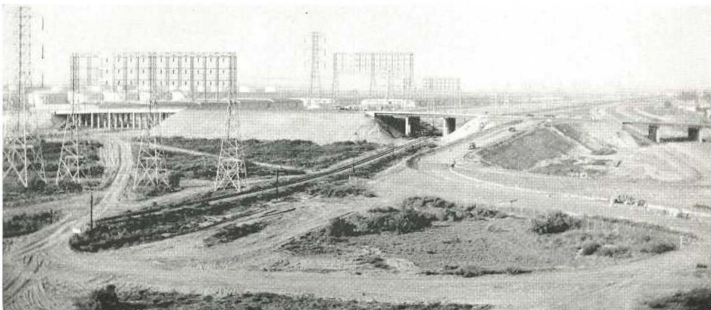
Looking north toward Classification Yard overhead which is on left. Hobson Avenue overhead is in center foreground and Terminal Island Freeway undercrossing on right
