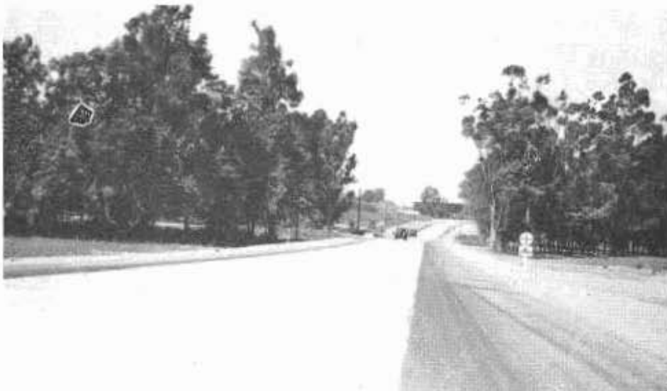
Looking northerly toward grade crossing of Union Pacific Railroad's Crestmore branch. Old road on left
