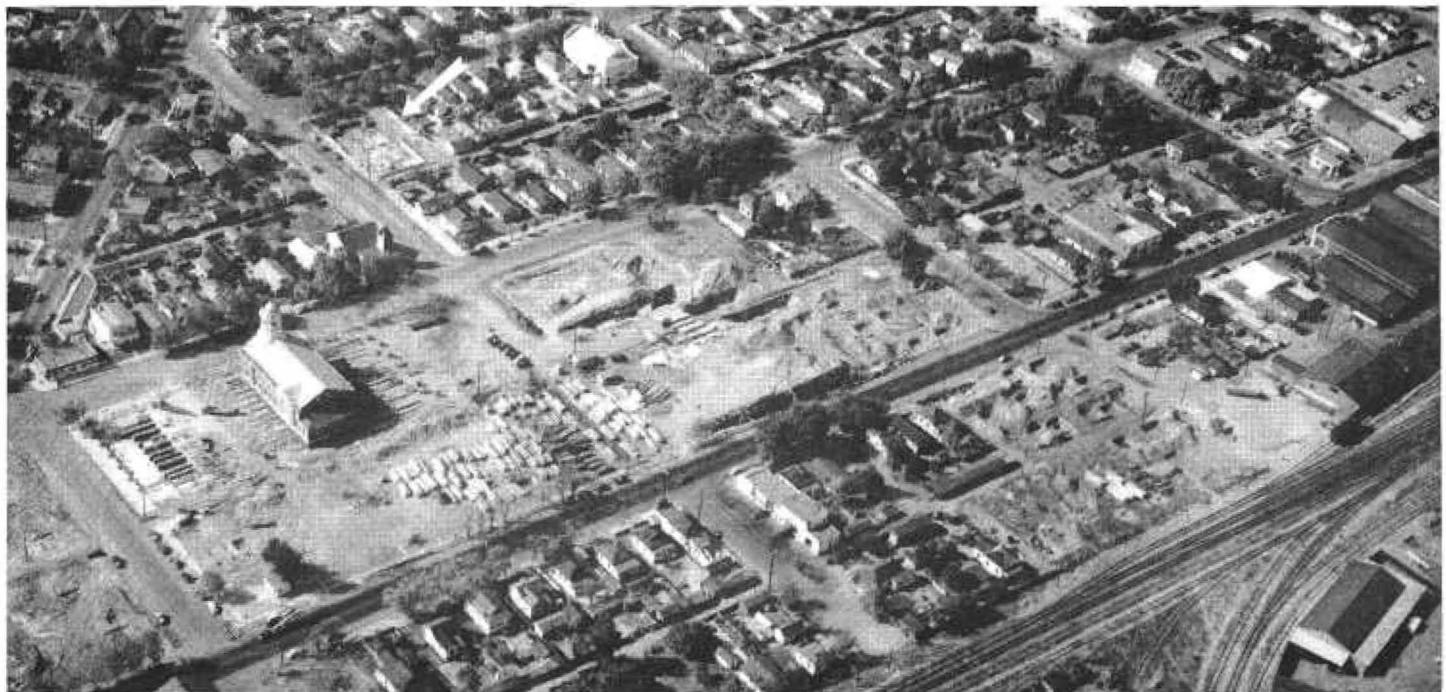
The church move from the air. Note the church on rails. The old foundation with part of the cribbing in left foreground; the new foundation being readied on the next street above as indicated by arrow
