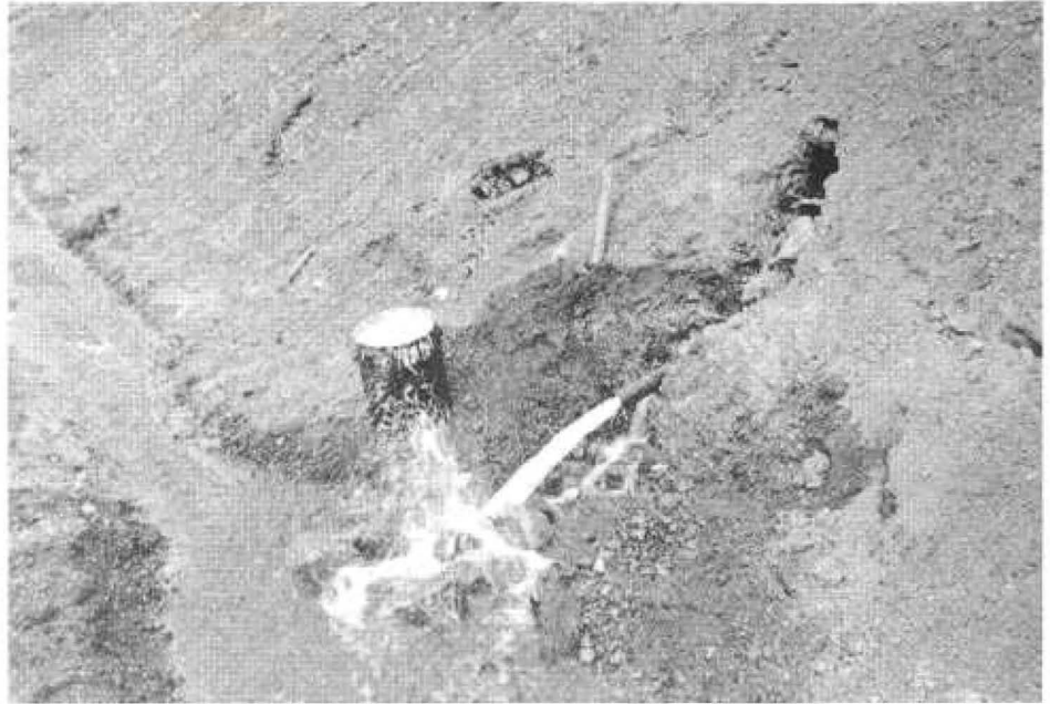
Flow from horizontal drain in Cloverdale slide at rate of six thousand gallons per hour
