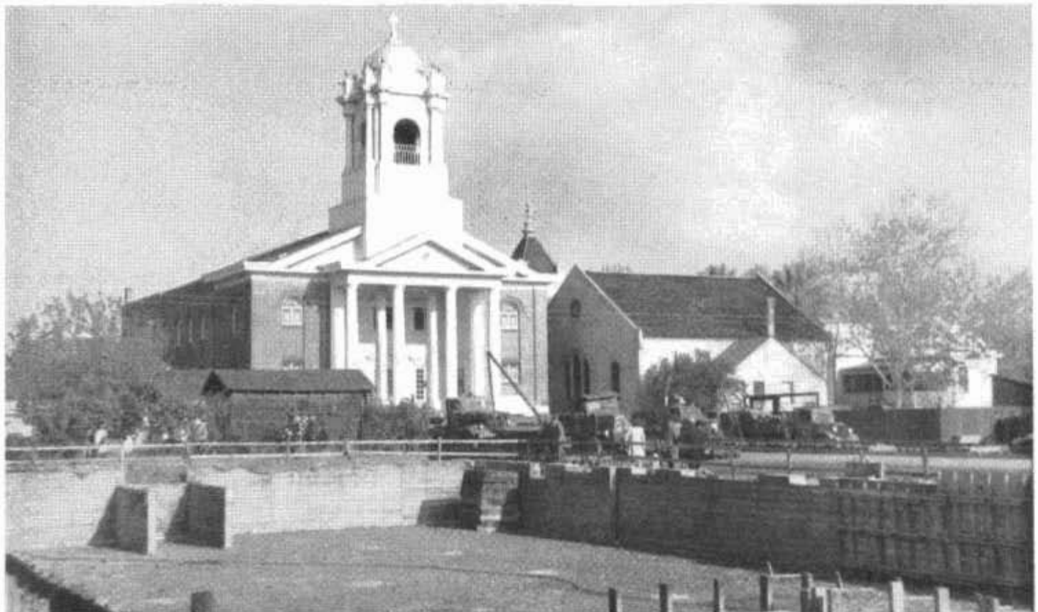
View of church being towed longitudinally along city streets with the newly constructed basement and concrete foundation in the foreground
