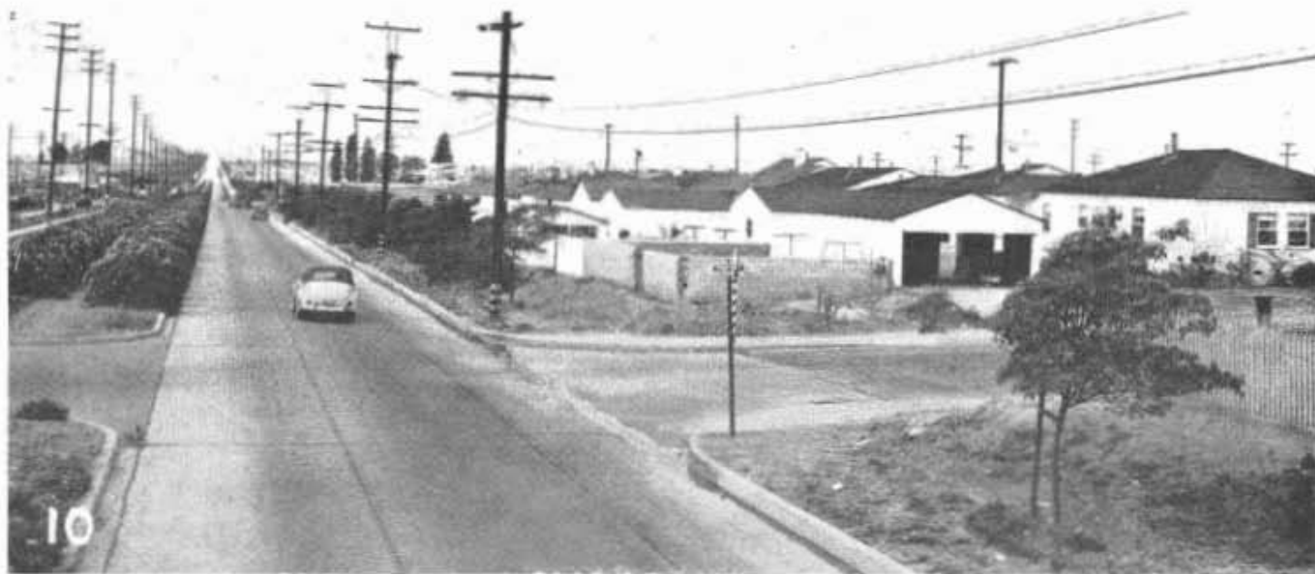
Looking west along Manchester Avenue at Truxton Avenue, in southwest Los Angeles
