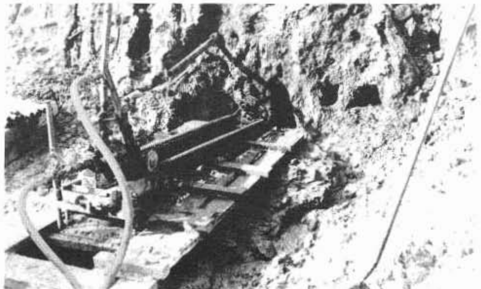
Drilling slide at Camp Cajon with hydrauger
