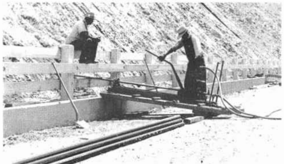
Hydrauger in drilling position at Grapevine slide
