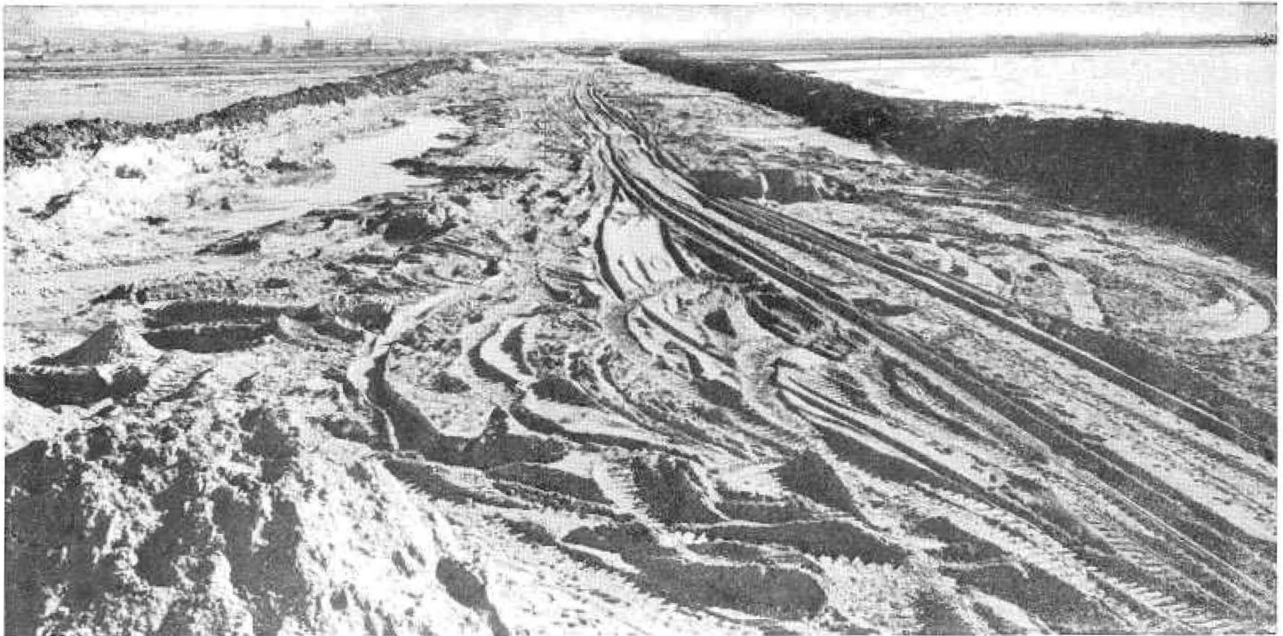
Damon Slough, looking south, showing completion of first link of hydraulic fill.
