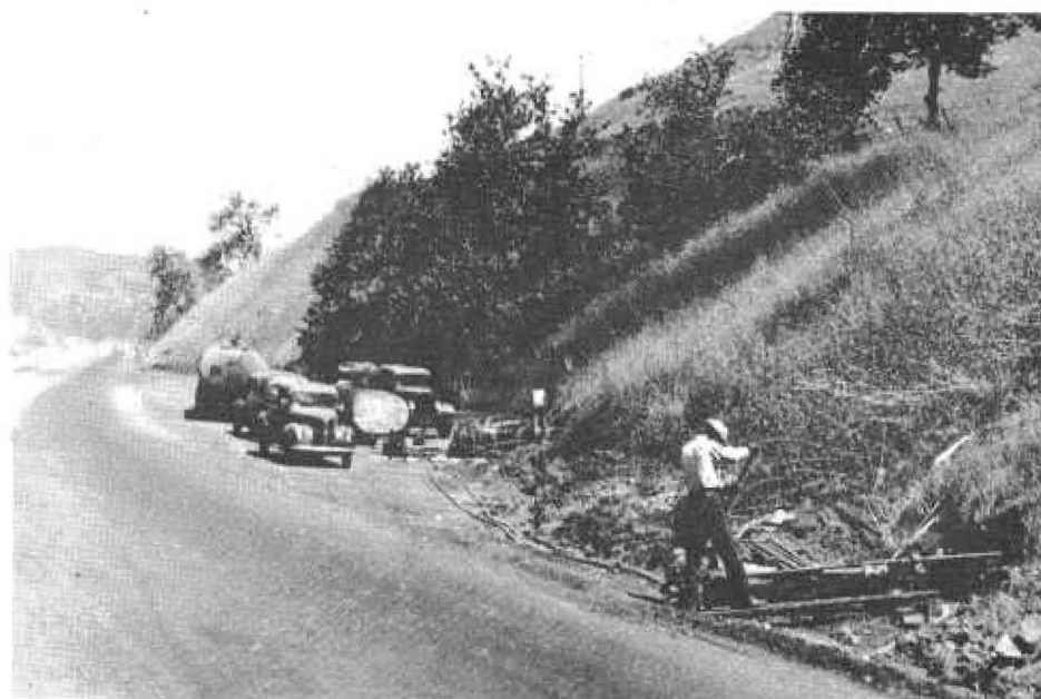
Two units drilling at Cuesta Grade
