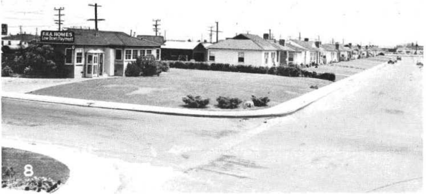
This is front view of subdivision section shown in photograph No. 7
