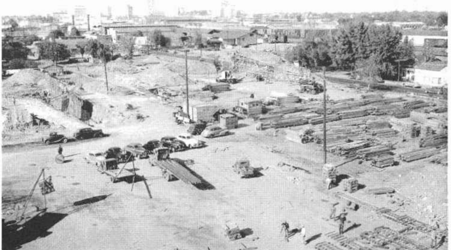
UPPER—View southerly from the church tower during the move. The old foundation with part of the cribbing used in the move is in the foreground with the cleared right of way extending beyond. Once filled with buildings, there remained only the fire station on the left with the beer wholesaler just beyond and the bar being moved when the picture was taken. LOWER—View northerly from the church tower. In the foreground workmen are laying tracks for another move. Note the retaining walls for the Monterey Street overpass that curves to the right
