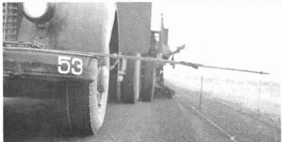
UPPER—Looking down on steering guide from operator's seat. CENTER—Side view of paver, showing steering guide. LOWER—Steering guide for trucks. →
