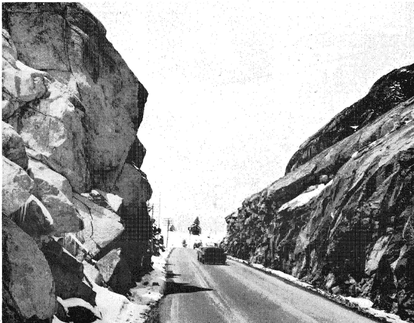
Looking west at rock cut to be widened at Donner Summit
