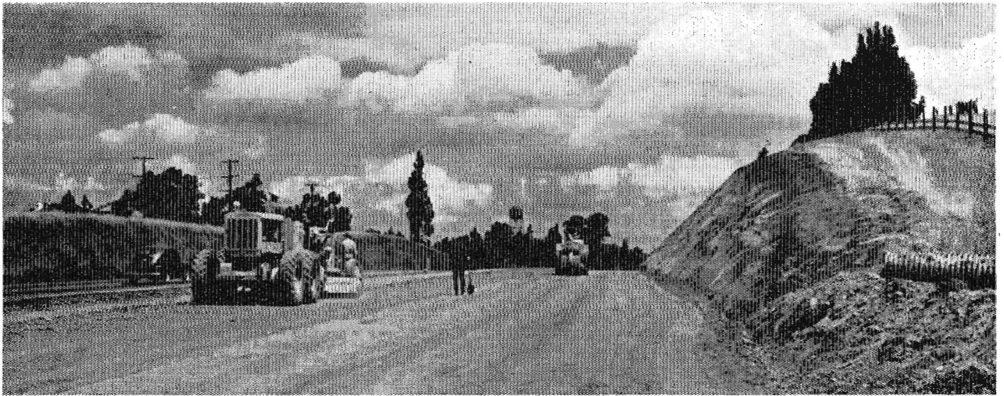
Finishing rough grade near Fleming Avenue
