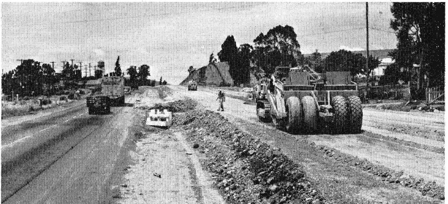
Finishing rough grade near Tennessee Street
