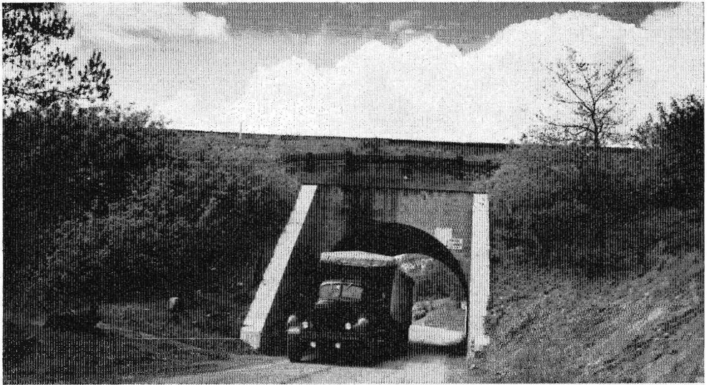
Old narrow underpass which is being replaced by the new Bailey Hill Underpass
