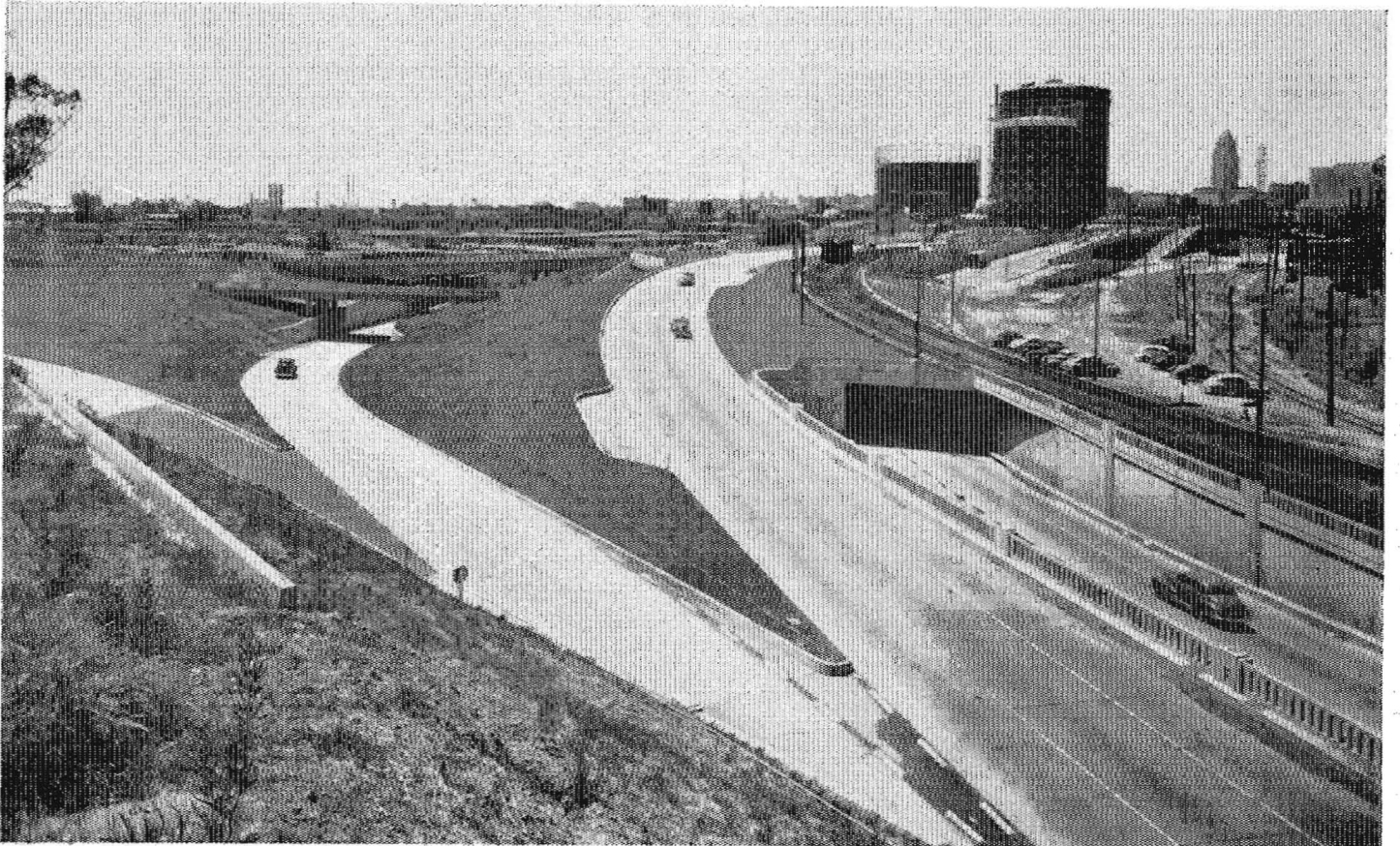
LOWER—Junction between Ramona Freeway and Santa Ana Freeway, looking westerly, showing general view of the fully completed Aliso Street grade separation crossing
