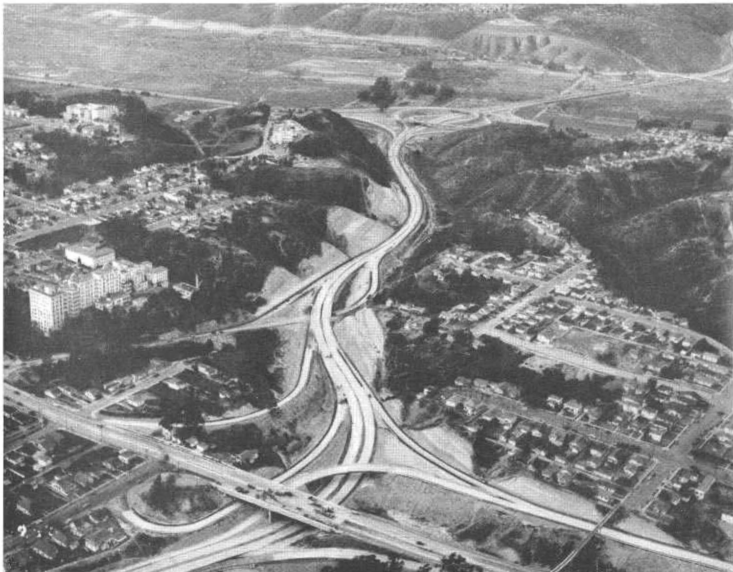
Cabrillo Freeway traversing Hillcrest District, with separations in the foreground across Robinson, University, Washington, and Pascoe Streets
