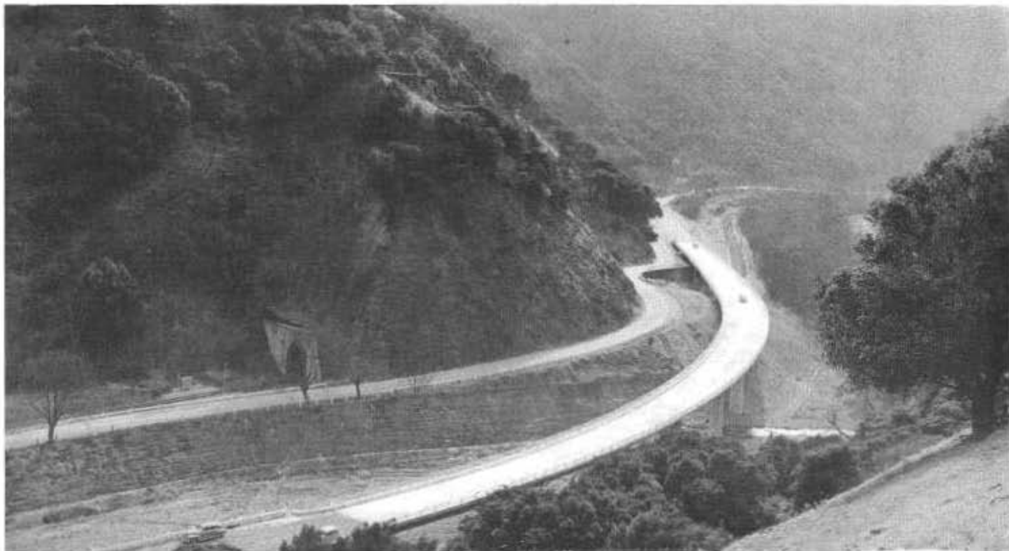
This is the new $450,000 Alameda Creek Bridge and overhead four miles east of Niles in Alameda County
