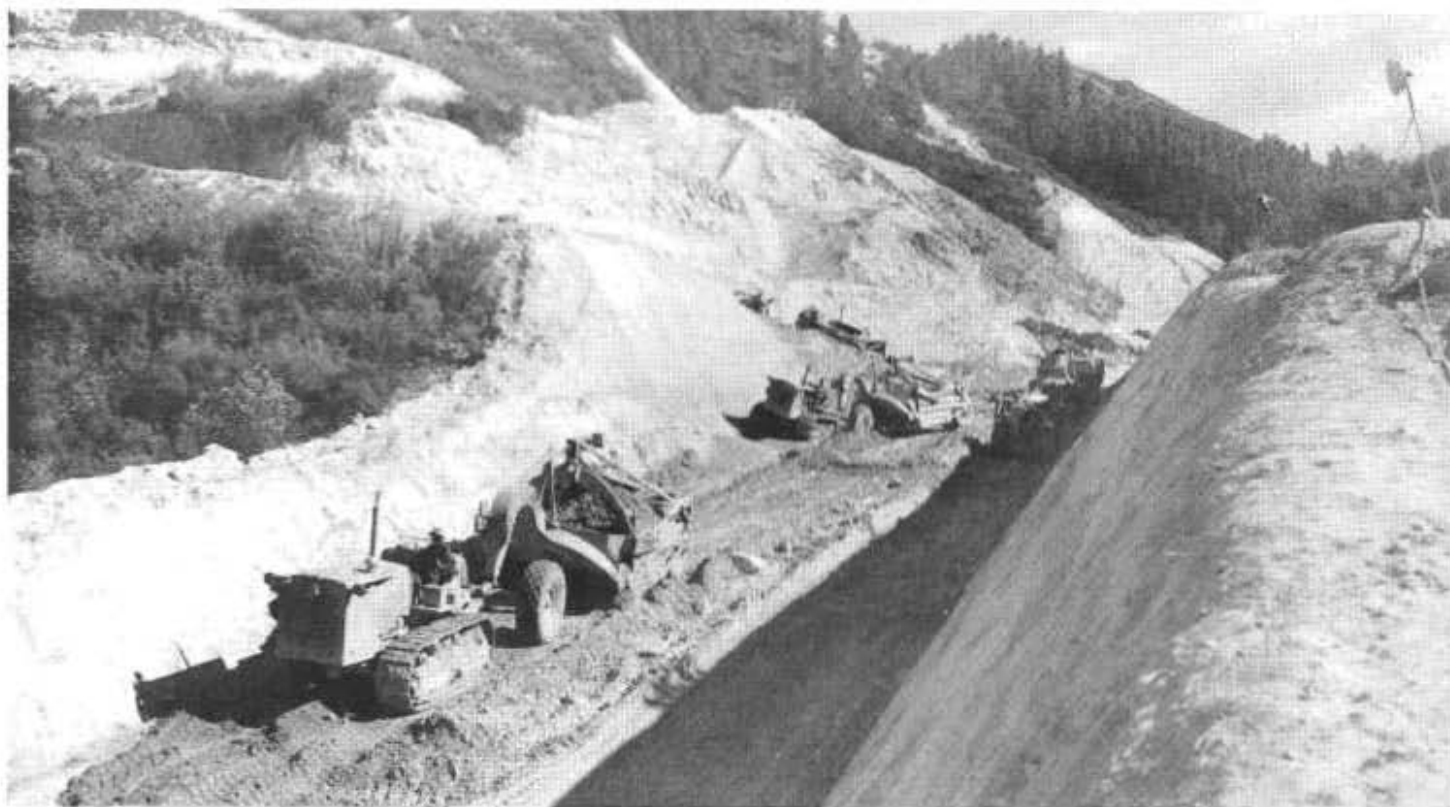
Typical view of grading operations on the Second Unit of the City Creek Road now under construction in San Bernardino County
