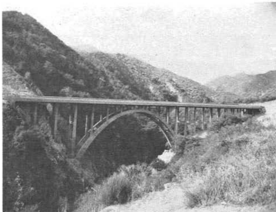
Recently completed arch bridge, which will provide a link in the new City Creek Road near San Bernardino
