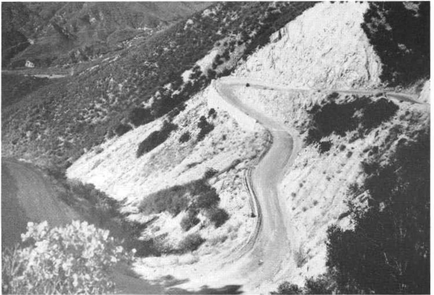
View of present City Creek Road on the Second Unit, looking down toward "Dutch John's Flat." Its steep grades, sharp curves, and narrow roadway are now being replaced by a modern mountain highway
