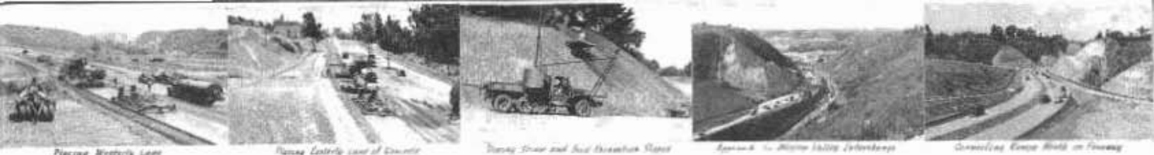
Placing Concrete Slabs
