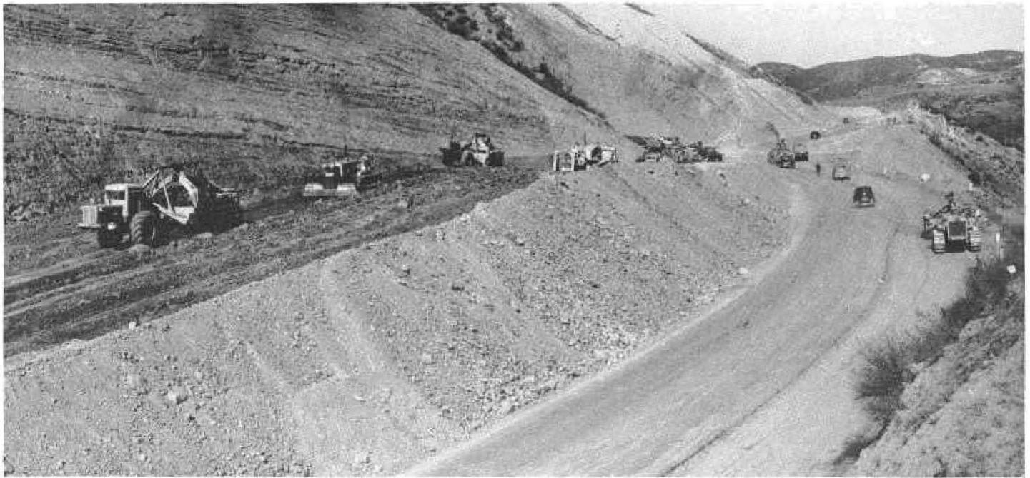
Heavy grading on five-mile grade north of Castaic
