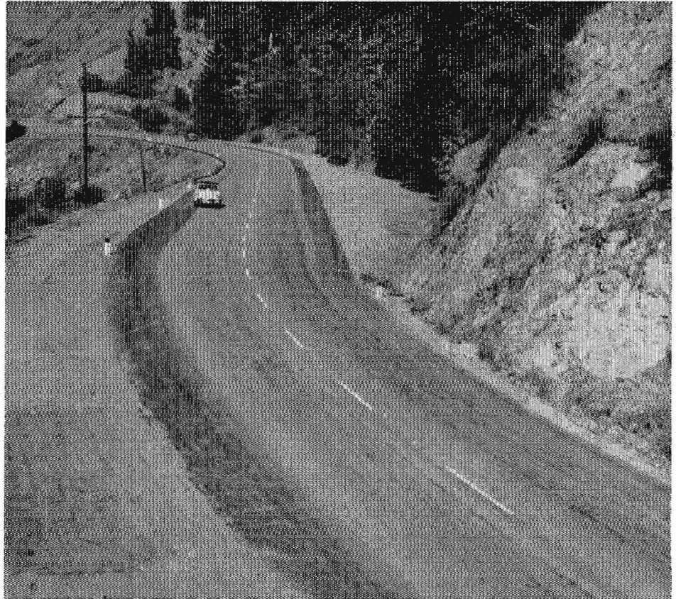
Upper—Wide roadway replaces former narrow road through unstable area. Lower—Easy curves along Eel River replace former winding road
