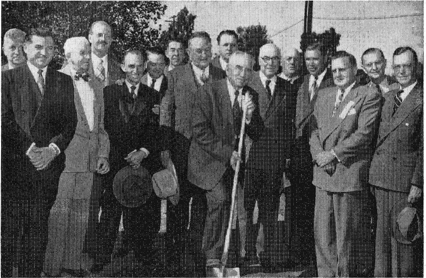
Charles C. Lee spades first earth for Roseville Underpass. Left to right: Stewart Mitchell, Bridge Engineer, Division of Highways; Joseph T. Barbieri, President Roseville Chamber of Commerce; C. H. Whitmore, Marysville, District Highway Engineer; Councilman James Ford, Supervisor J. B. Paolini, Councilman Joe Colnar, Herbert S. Booth of Guy F. Atkinson Company; J. L. Seawell, State Board of Equalization; Mayor Harold T. Johnson, Senator-elect; Mr. Lee; Director of Public Works C. H. Purcell; M. L. Jennings, Division Superintendent, Southern Pacific; J. W. Corbett, San Francisco, Vice-President, Southern Pacific; Carl G. Laughridge, Secretary-Manager Roseville Chamber of Commerce; Deputy State Highway Engineer Fred J. Grumm, and Earl Mayo, Chief Engineer, Southern Pacific
