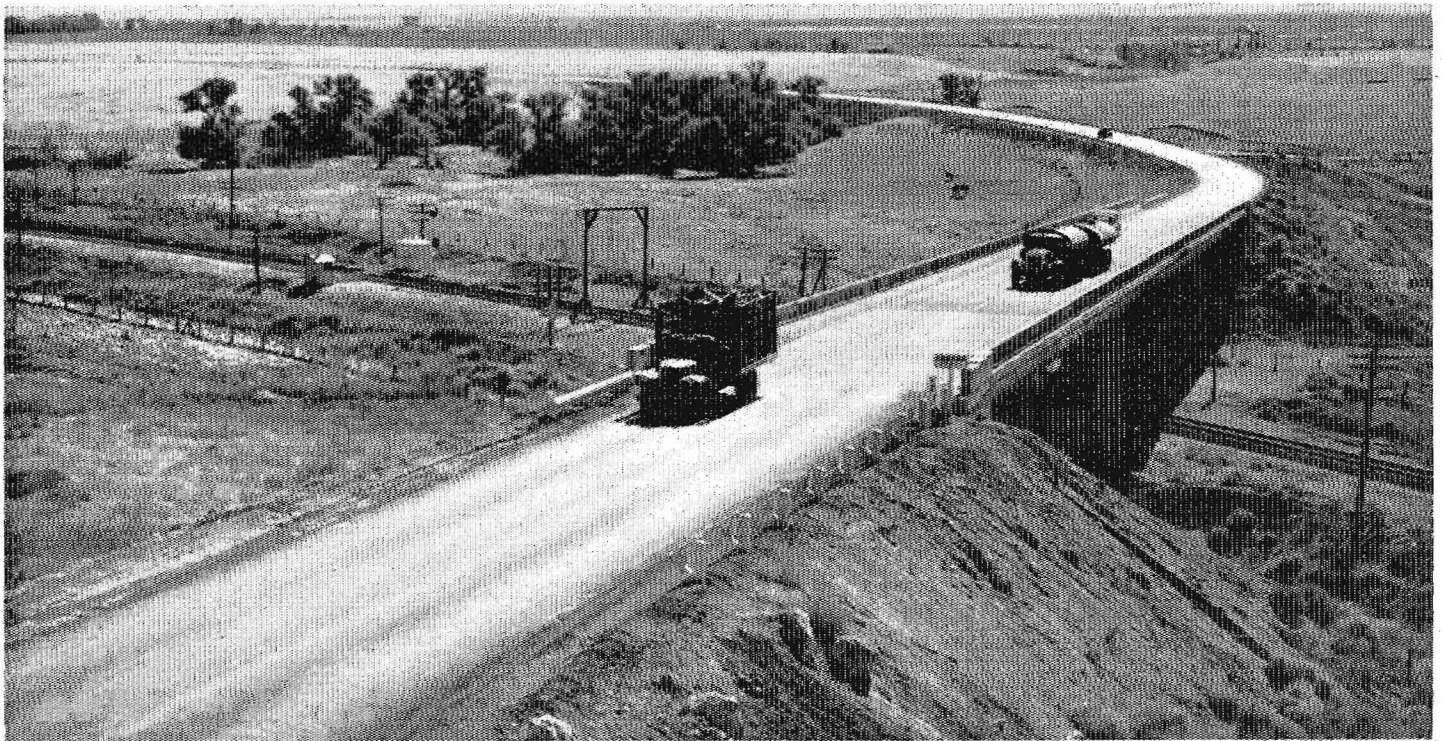
This view shows new Keene-Tehachapi highway crossing Tehachapi Overhead
