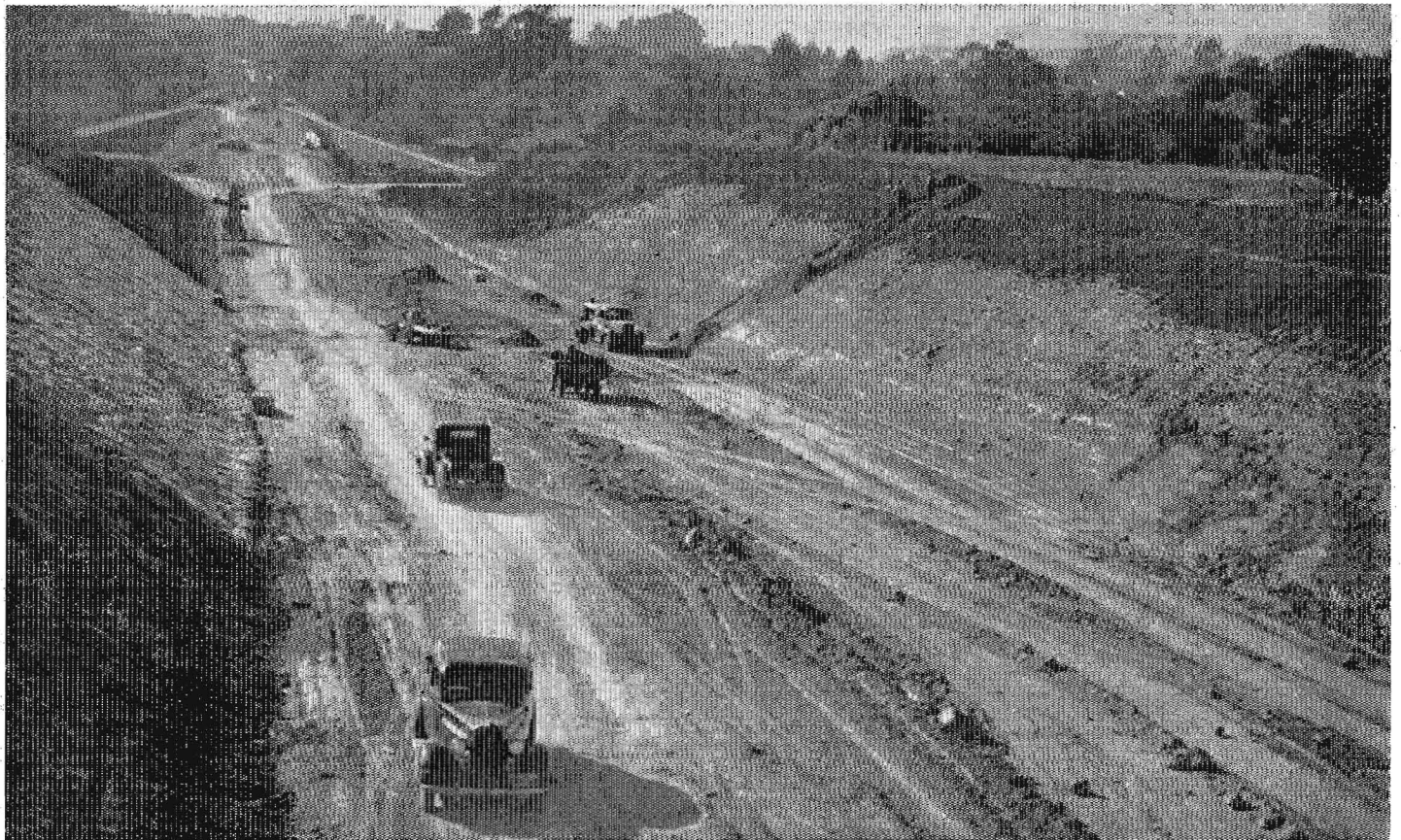
Deep excavation work in progress on new freeway near Soquel, looking toward Santa Cruz (see Page 10)
