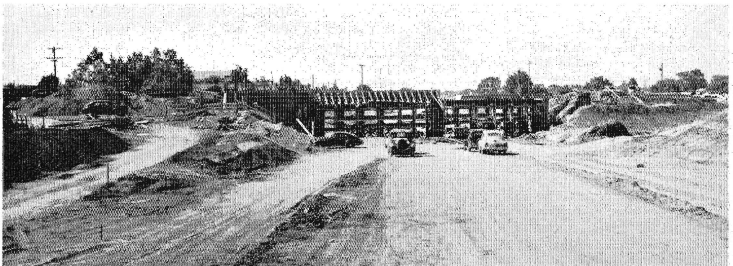
One of structures on Stockton By-pass now under construction
