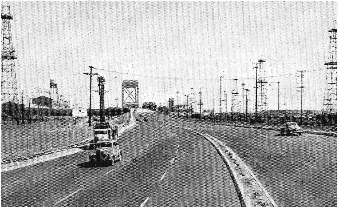
Terminal Island Freeway looking south toward Cerritos Channel Bridge
