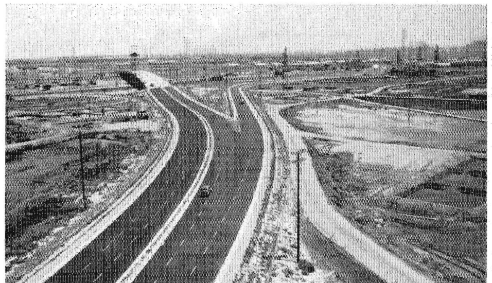
Freeway looking northeasterly toward Anaheim Street Viaduct over Union Pacific, Southern Pacific, and Pacific Electric Railroad tracks, and Anaheim and I Streets. Off ramp to Anaheim Street in Long Beach is roadway to right
