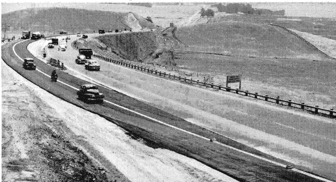
US 40 for a distance of 4.6 miles through the American Canyon is being widened to four-lane divided standards
