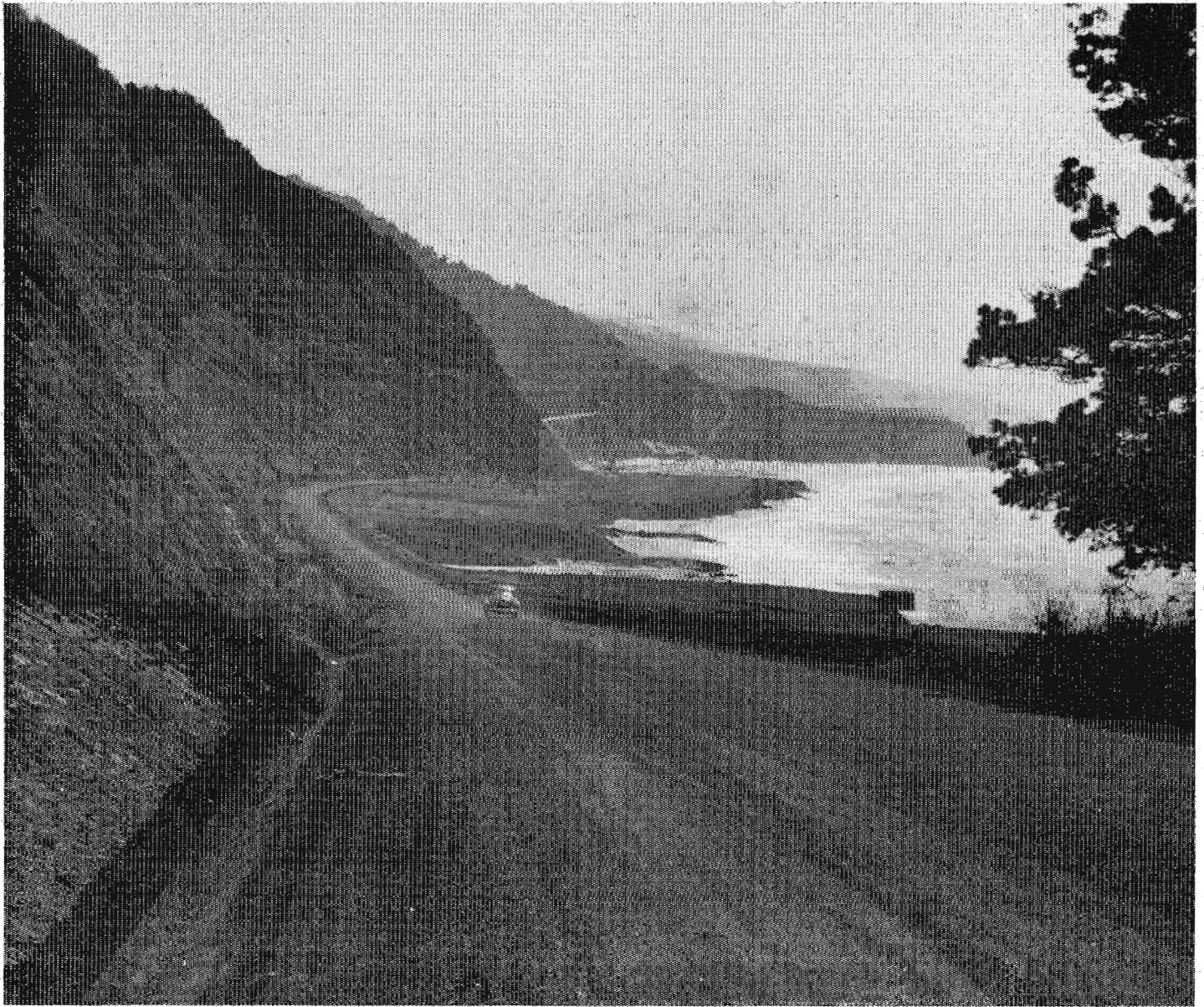
When this picture of the new Waddell Bluffs Highway was taken, paving and striping were about to begin
