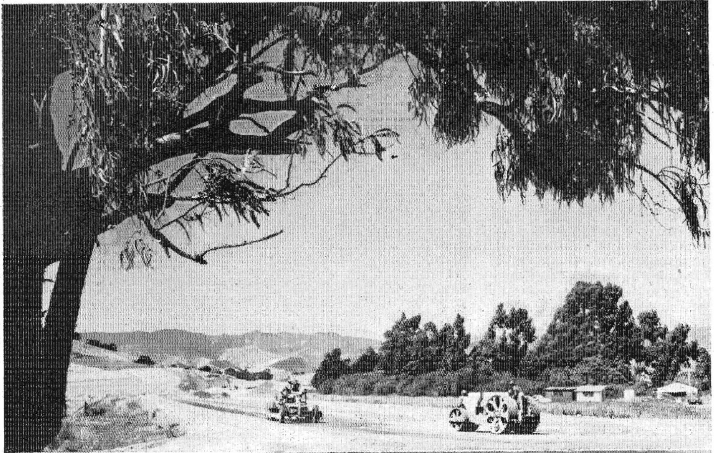
Upper—Looking north from French Street, making finished grade. Lower—Freeway looking northerly, showing Santa Lucia Range in distance
