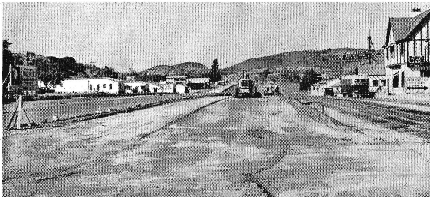
Looking northerly through Buellton, showing construction under way. All structures on right and left were moved back off the existing 60-foot right of way to provide a roadway width of 176 feet
