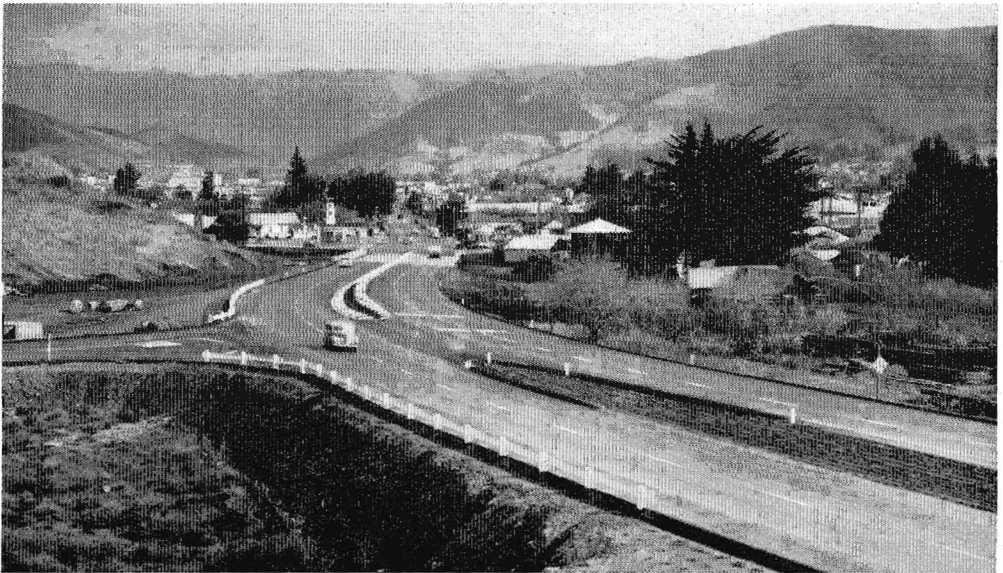
New four-lane divided freeway at southerly entrance to San Luis Obispo
