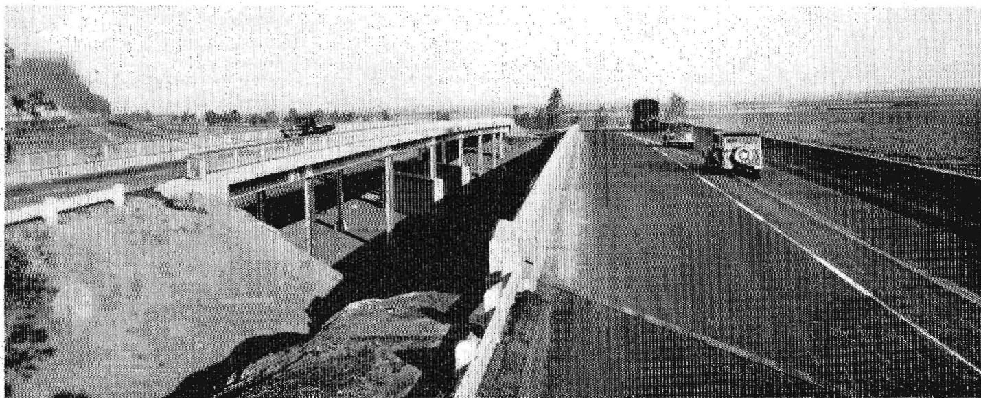
Looking northerly from south end of existing overpass at main line tracks of the Southern Pacific. New structure is on the left
