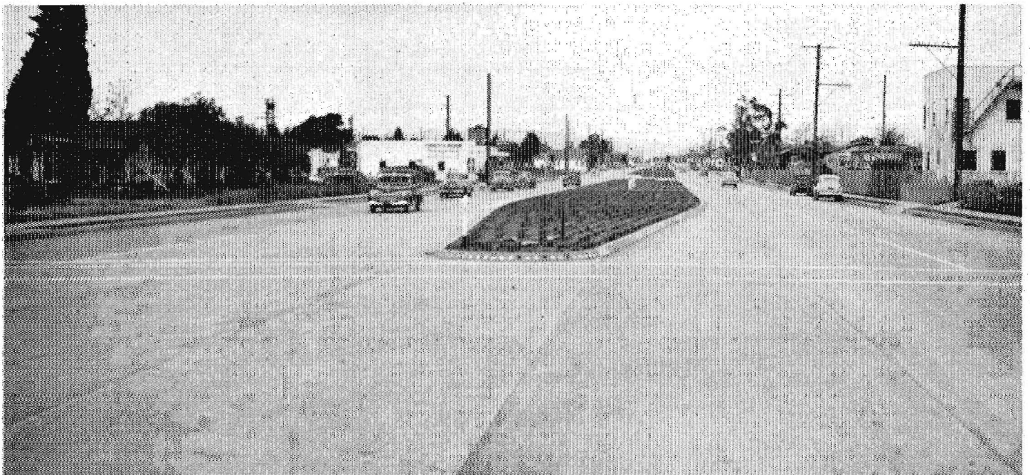
Olympic Boulevard extension looking easterly from near Lincoln Boulevard, showing newly completed divided highway construction
