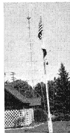
LOWER—Radio antennae tower at Garberville
