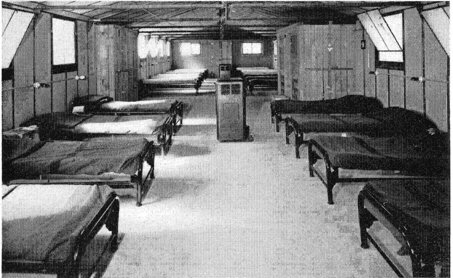
Upper—Barracks housing 24 men each at Camp 40 in San Diego County. Lower—Interior of one of the 24-man barracks at Camp 40
