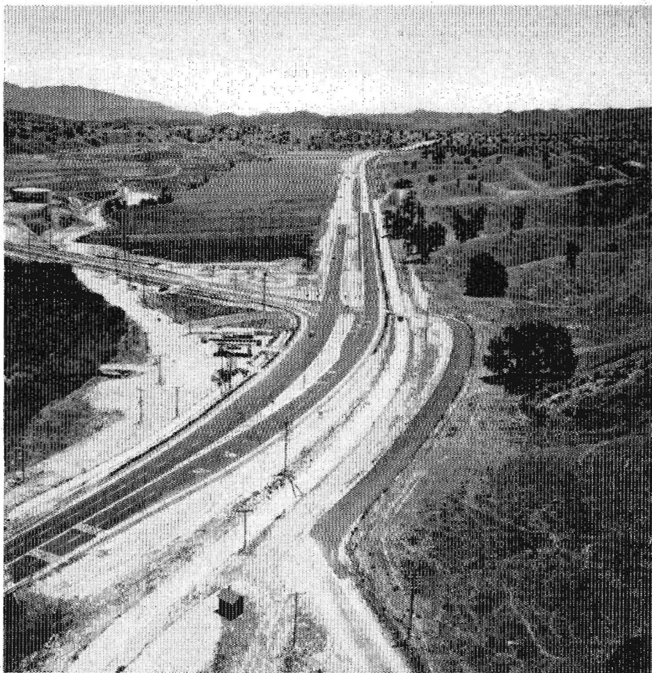
Completed section of Ridge Route looking southerly from the Santa Clara River crossing, showing channelized intersection with State Highway Route 79 to Saugus
