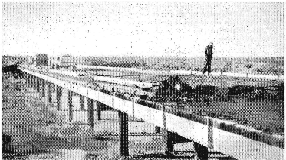
Removing surfacing from desert bridge preparatory to redecking
