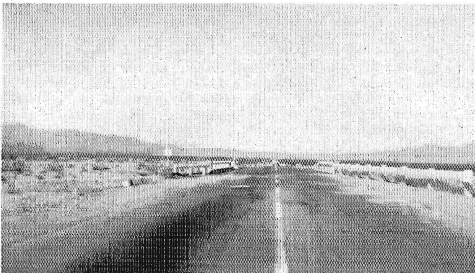
Typical desert alignment and typical desert bridge
