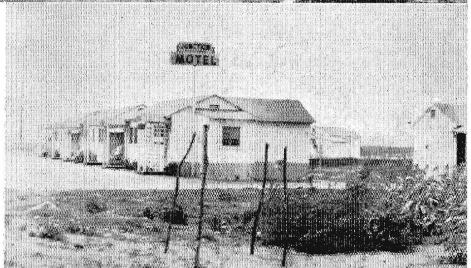
Upper—Photo taken in May, 1949. At right center is a boulevard stop for cars entering the freeway from the outer highway. Lower—Photo taken in October, 1946. Motel units shown in center of picture were moved back to make room for outer highway construction
