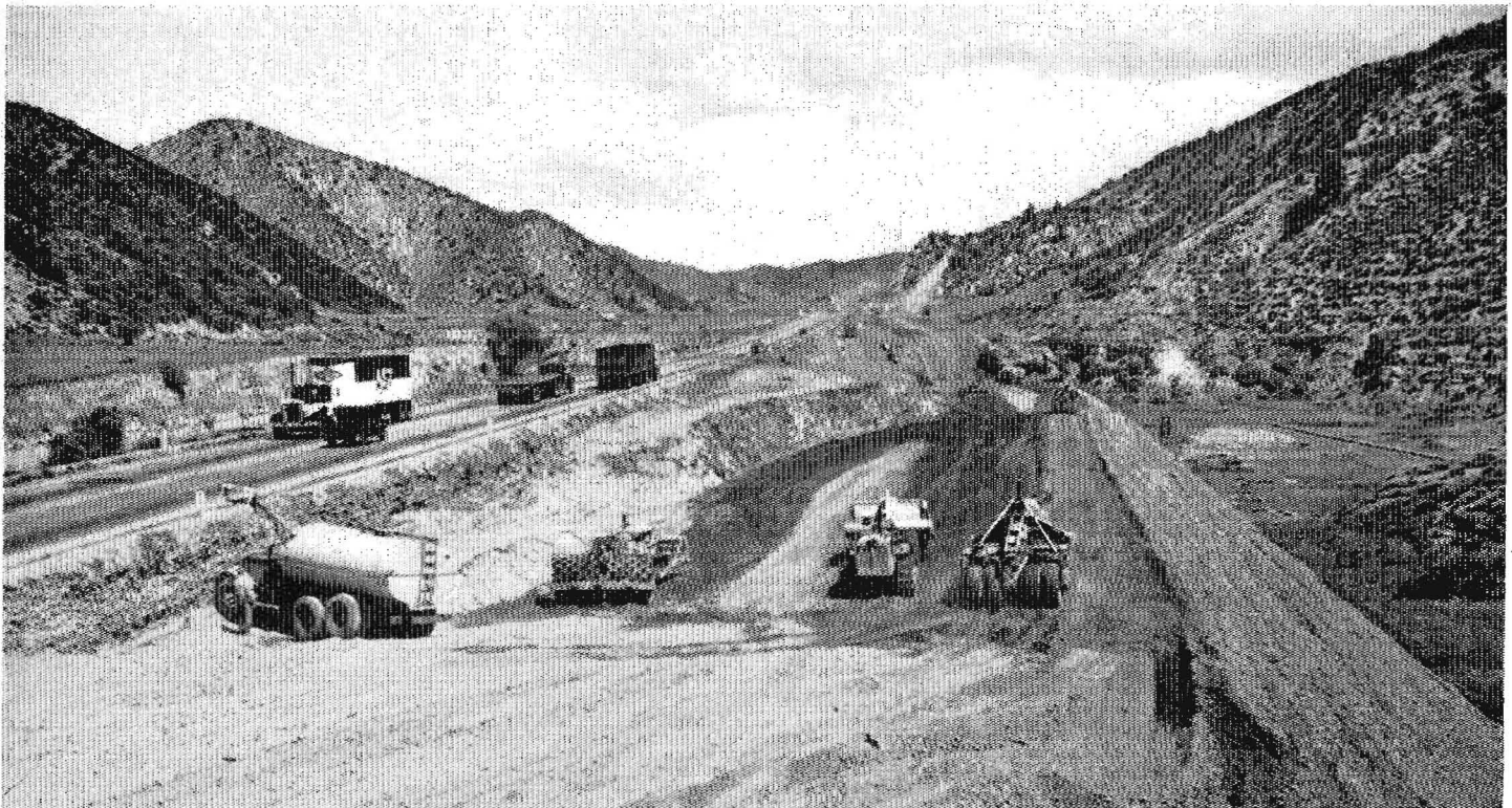
Portion of Ridge Route near northerly end, showing grading operations in progress. Existing 30-foot pavement now used for two-way traffic will become one-way roadway for southbound traffic after the new roadway for northbound traffic is completed
