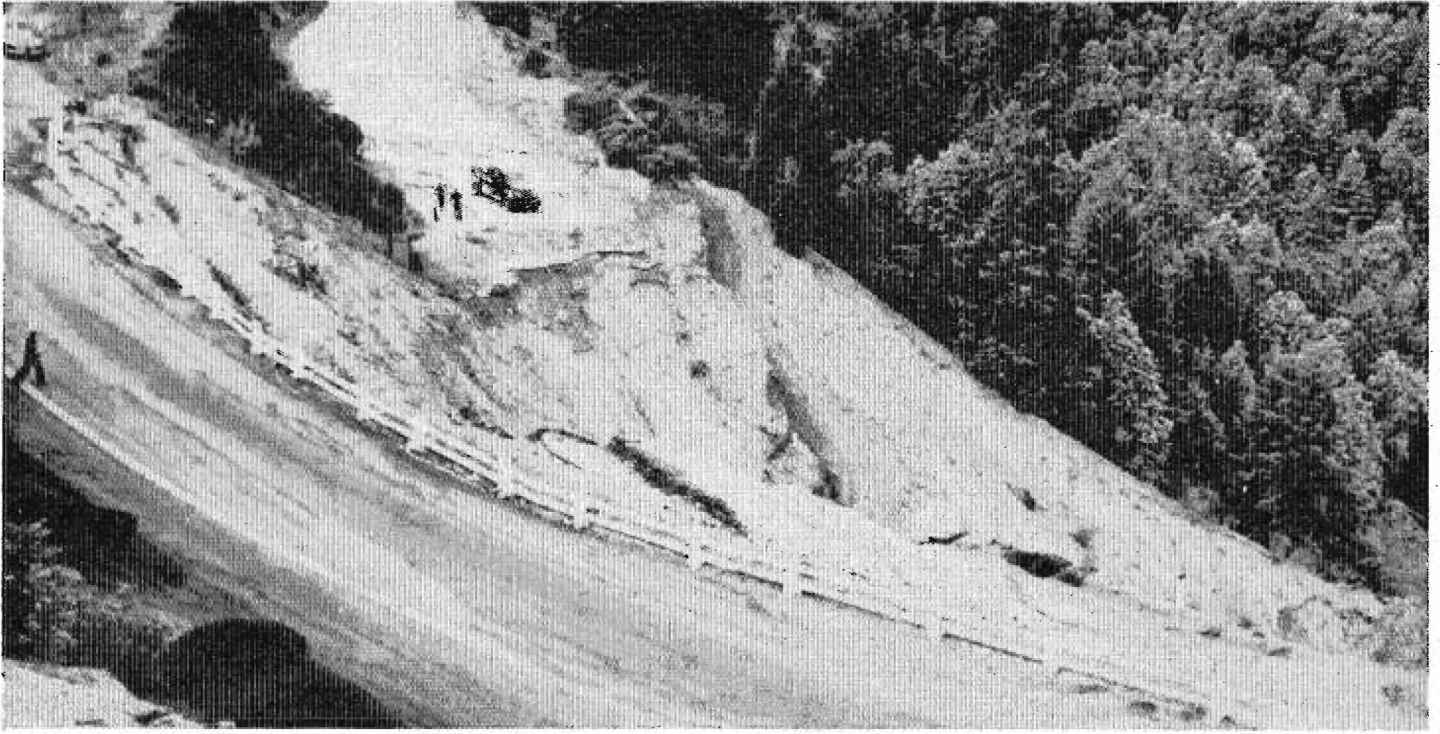
Large fill slipout was later corrected by combination of stripping, rock drains, toe support fill and horizontal drains
