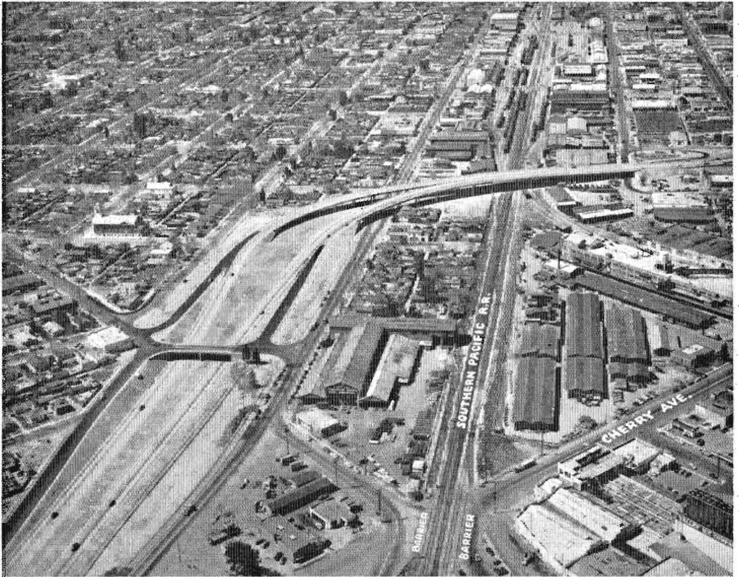
Aerial view of recently completed Monterey overhead in Fresno. Cherry Avenue now closed at Southern Pacific Railroad grade crossing
