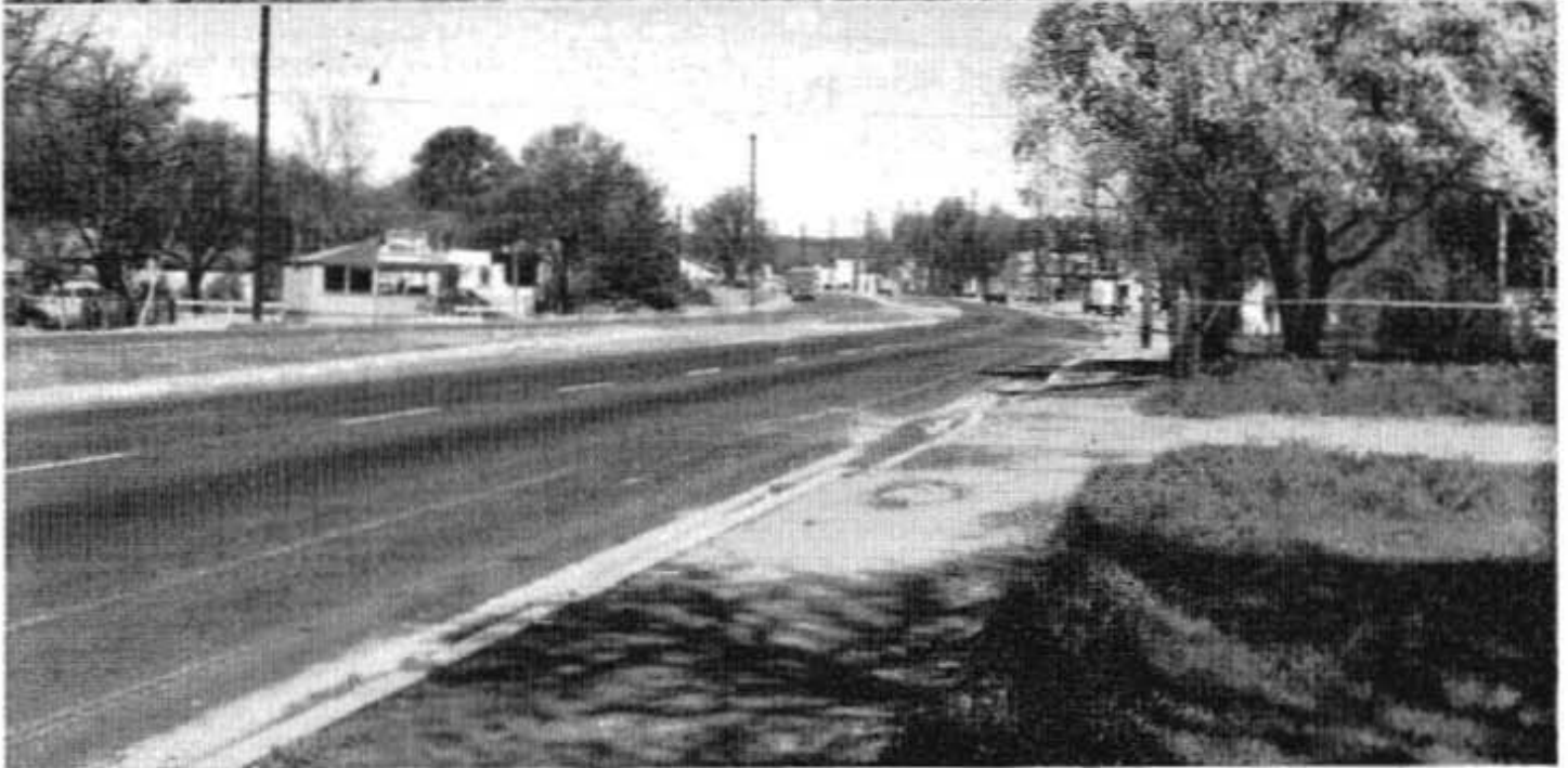
Upper—Aerial view showing old, winding road on left and new highway on right on top of Cottonwood Hill. Lower—Four-lane divided highway into Cottonwood
