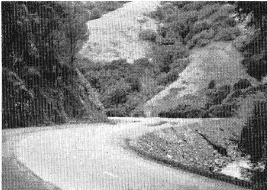
Looking eastward at rock cut, where double reverse curve was eliminated
