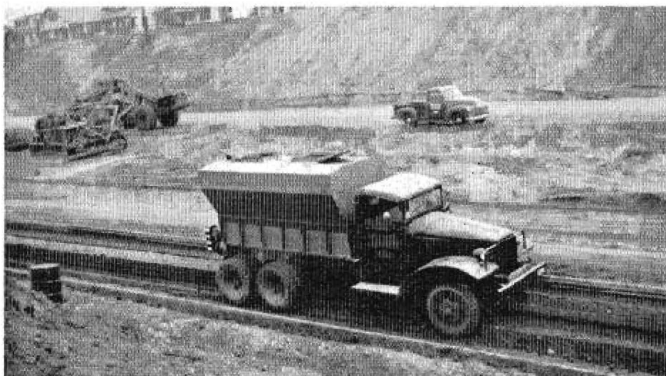
Center—Cement spreader truck in operation
