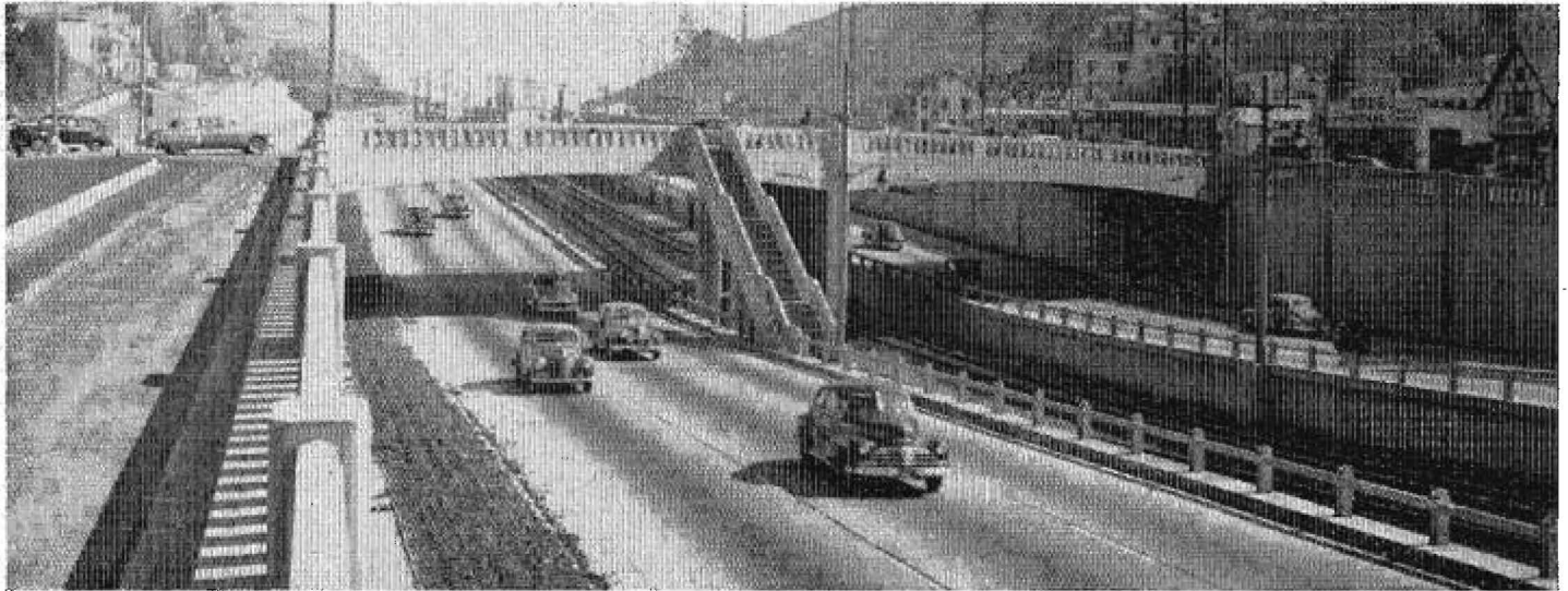
This is a closeup of the Barham Boulevard separation structure completed some years ago under a Los Angeles city contract
