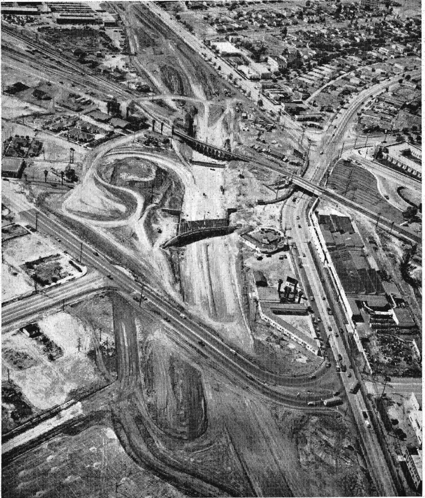
Aerial view of construction area on Santa Ana Parkway looking westerly, Atlantic Boulevard detour in foreground with new grade separation and Union Pacific Railroad shoofly trestle in center
