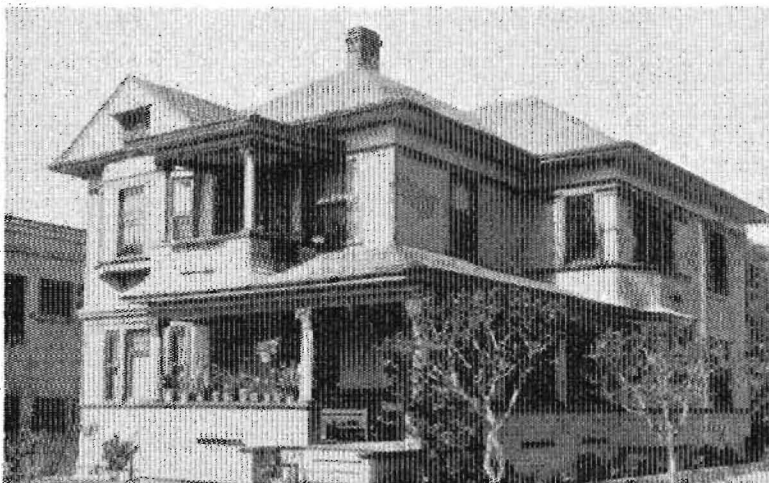
BEFORE —The old-fashioned structure pictured above was formerly located at 439 North Belmont Street. It was removed to allow construction of the Hollywood Freeway.
