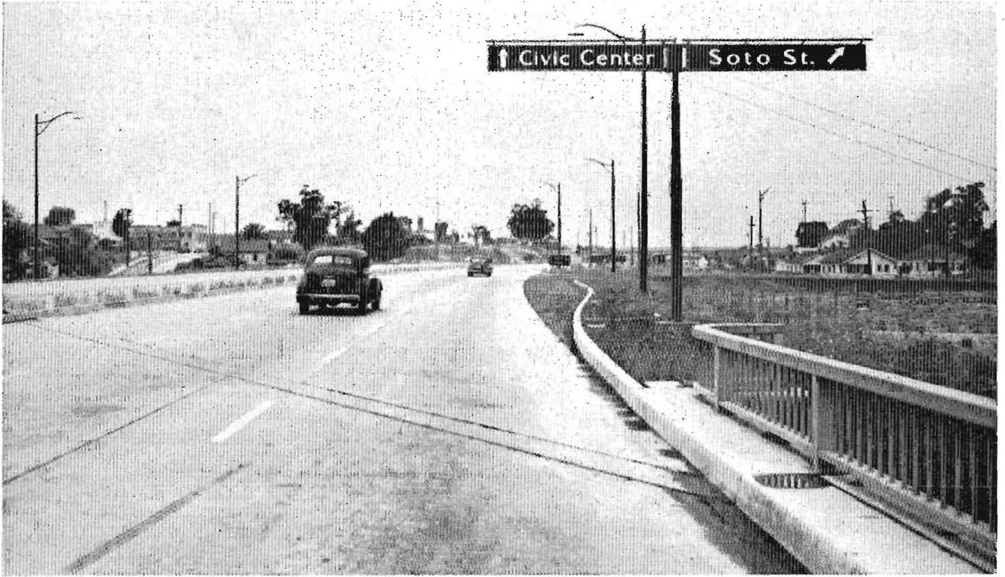
UPPER—View westerly along Santa Ana Freeway from Olympic Freeway grade separation bridge. LOWER—View easterly along the Santa Ana Freeway from near Grande Vista Street, showing Lorena Street grade separation bridge
