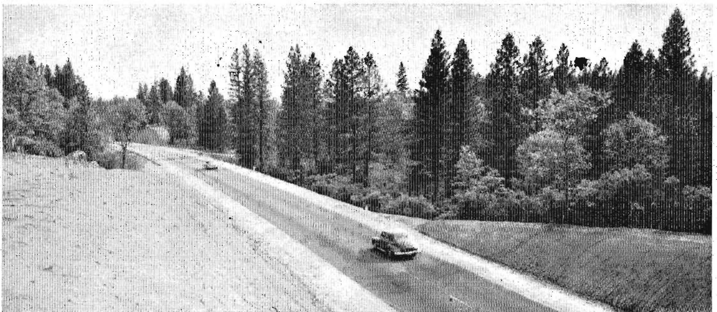
Looking toward Auburn from a point about two miles south of Grass Valley
