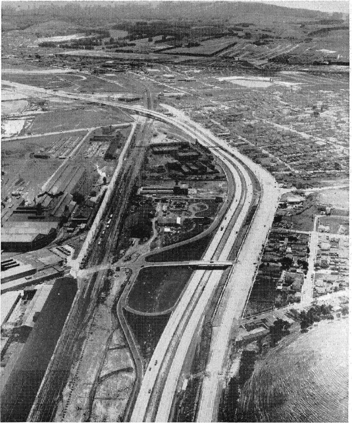
Butler Road overcrossing in South San Francisco. Pedestrian overcrossing in central section and Grand Avenue overcrossing in background
