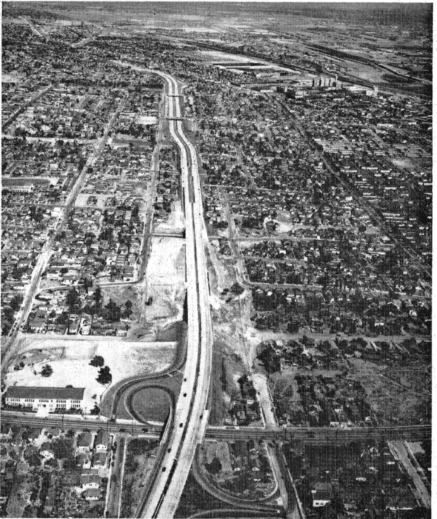
Aerial view taken May, 1949, from approximately same location as picture on opposite page, showing freeway construction completed easterly to Eastman Avenue and Public Works
