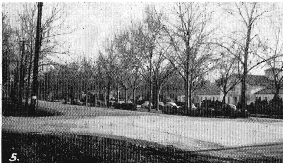
Parking along the outer highway leaves the main center roadway clear for through traffic
