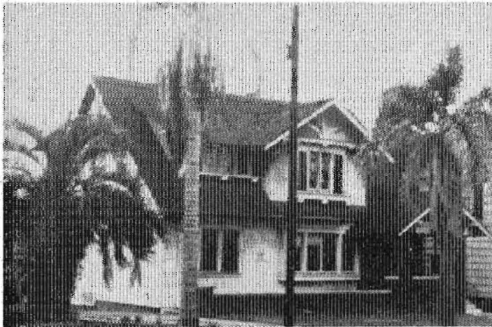
BEFORE —This typical old, two-story building was located at 1422 Bellevue in the right of way of the Hollywood Freeway.
