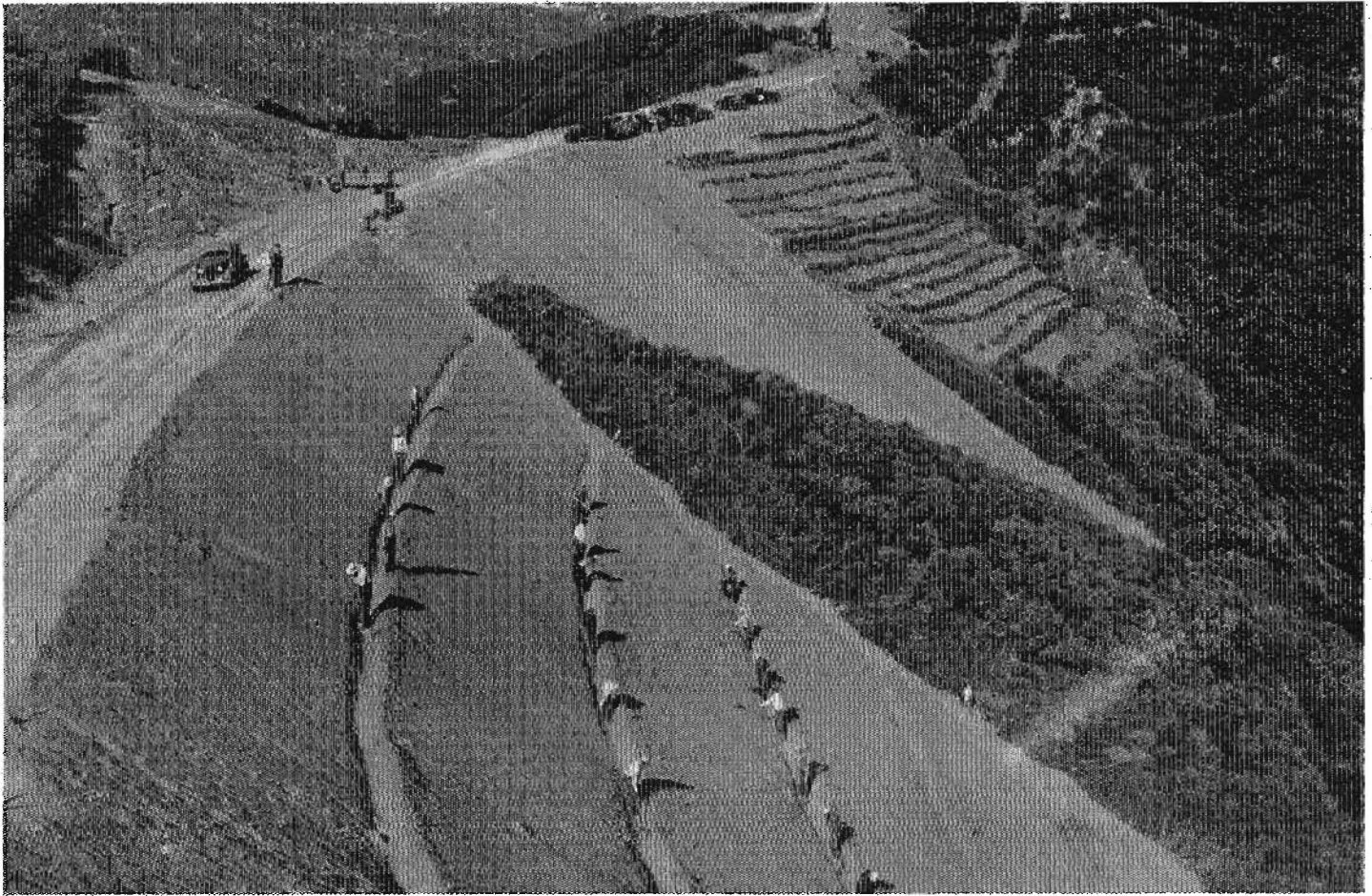
Erosion control with prison labor on Angeles Crest Highway, Los Angeles County, in 1938. Finished work is shown in background
