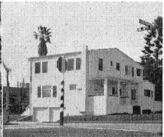
AFTER —The relocated building now stands at the northwest corner of Fourth Street and Serrano. It has been changed so as to be hardly recognizable.
