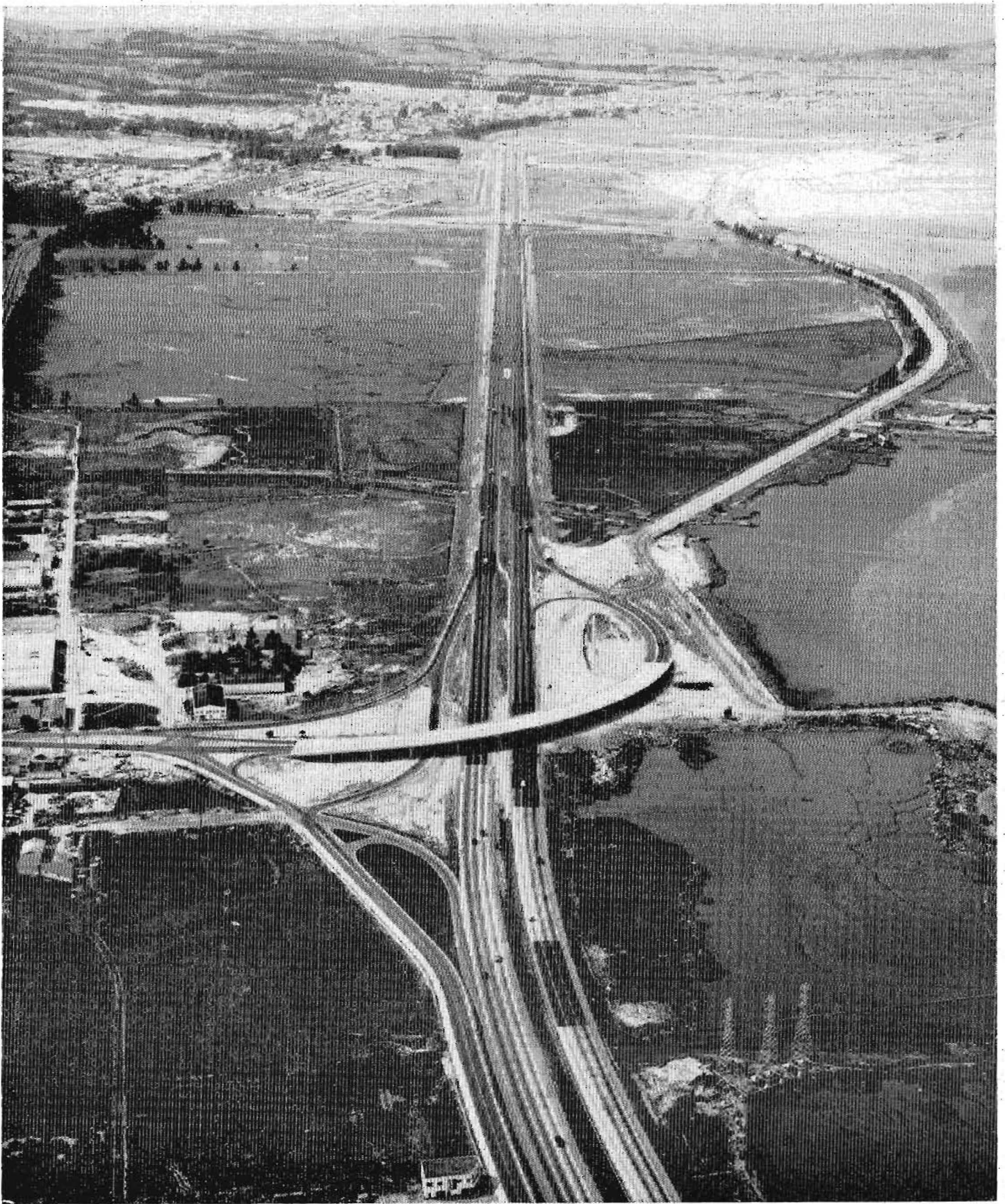
Broadway overcrossing in Burlingame looking north. Old Bayshore Highway is on right
