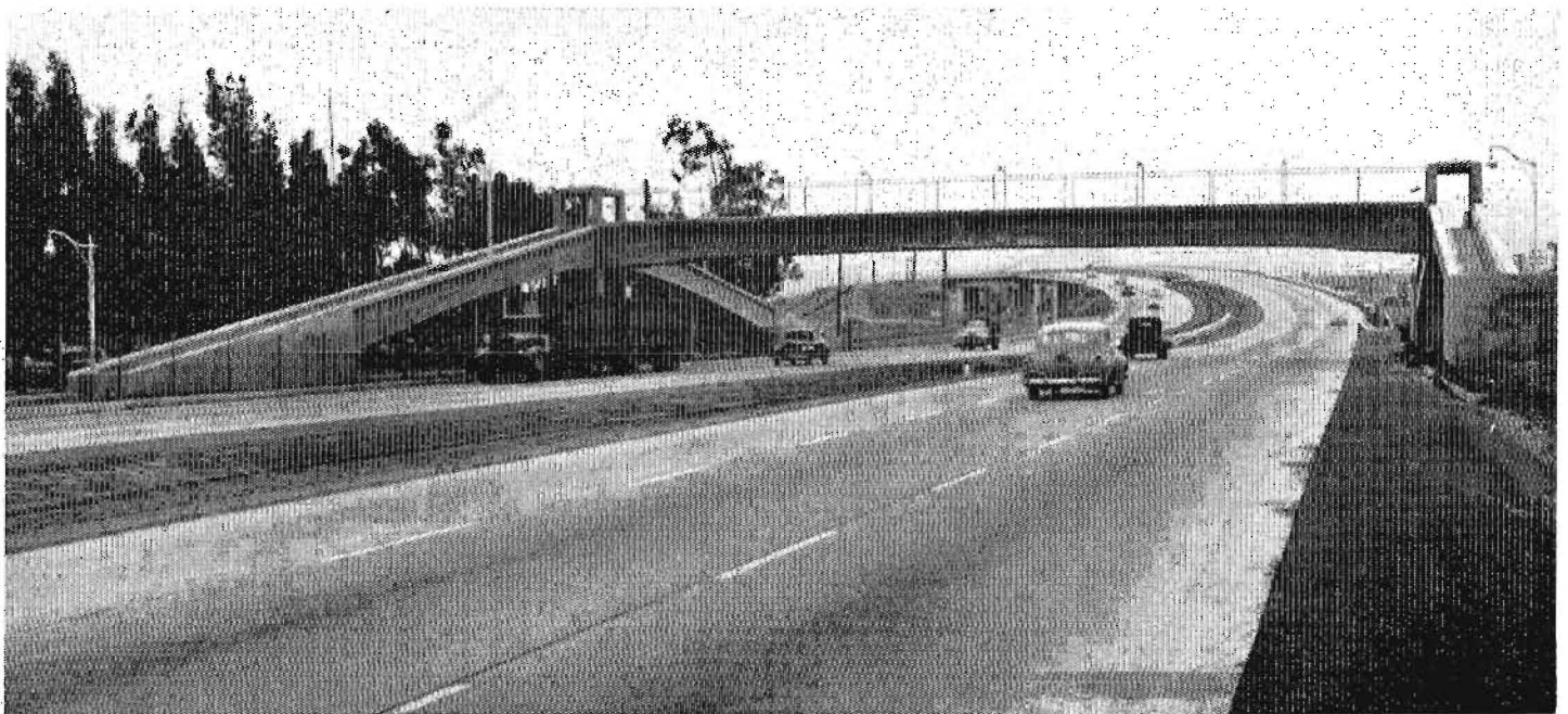
Pedestrian overpass in South San Francisco, showing 120-foot clear span across new Bayshore Freeway
