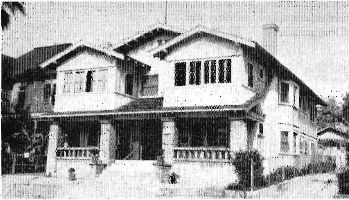
BEFORE —The large, old-fashioned two-story building pictured above was located at 433-437 North Beaudry in the right of way of the freeway and required considerable remodeling to retain attractiveness.
