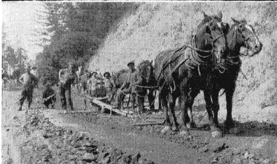
Hand labor methods of building highways in mountainous areas with inmate labor. UPPER—Track and dump car in Shasta County in 1916. LOWER—Teams, plows and fresno scrapers along Smith River in Del Norte County in 1923
