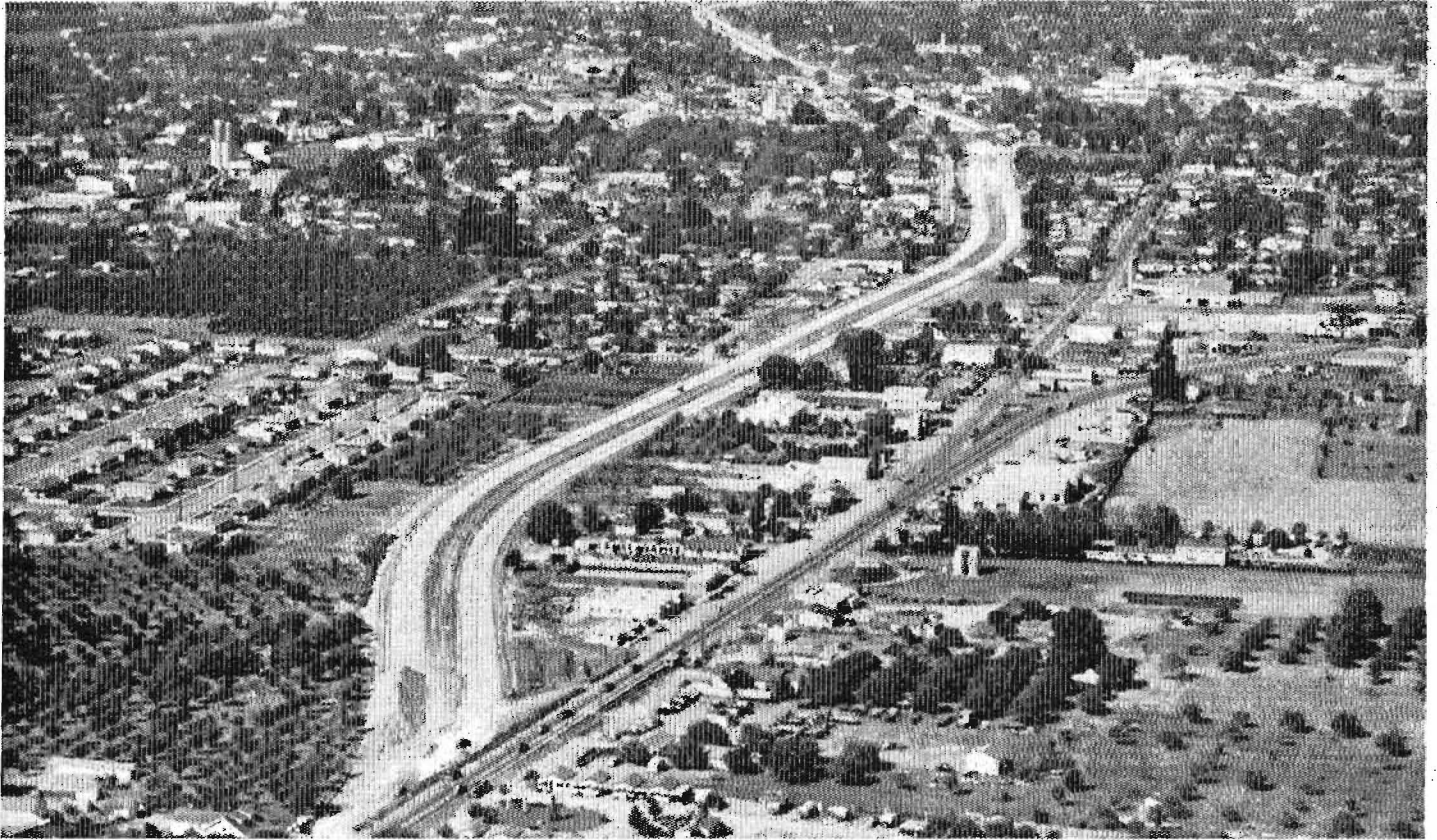
Aerial photo looking north from intersection of new freeway and existing highway south of Santa Rosa. This was taken in October, 1948, when grading was completed and paving started north of Santa Rosa Creek only, and clearly shows the new freeway in comparison to the old route through town
